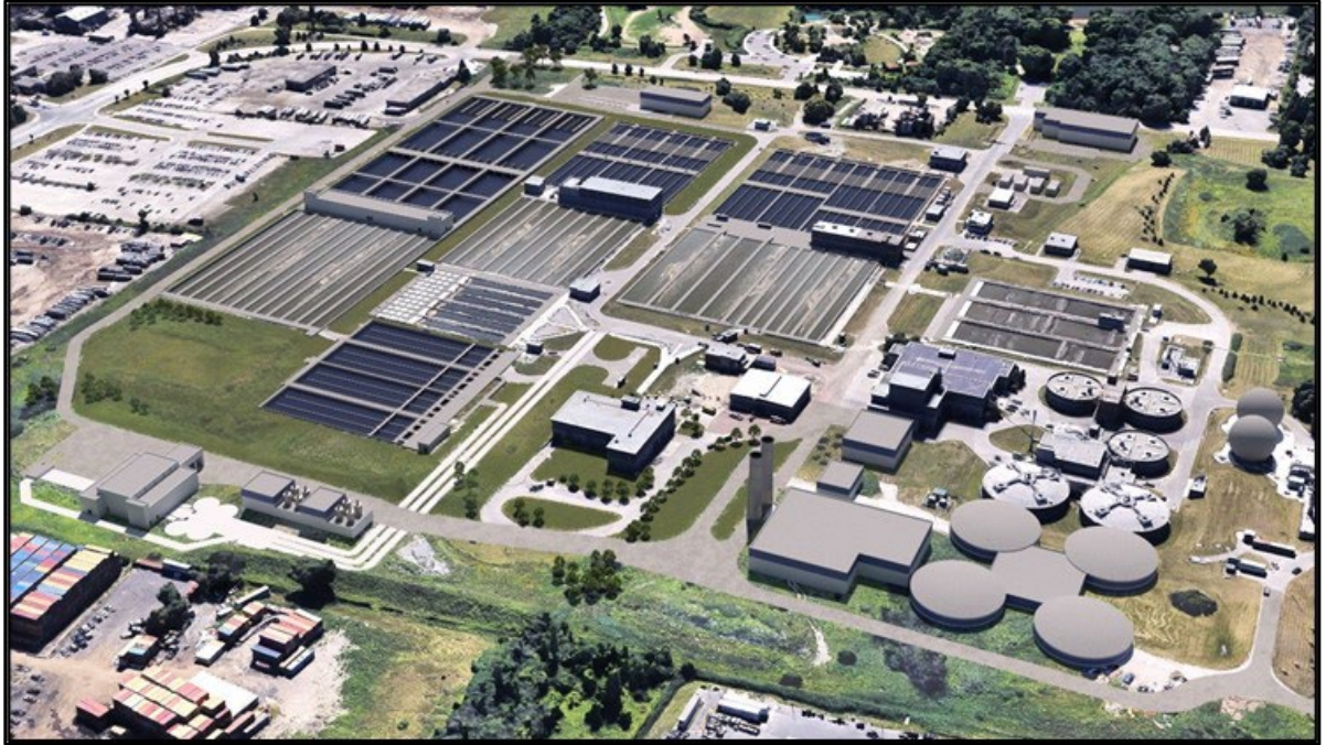
Figure 9-3. Future Clarkson WRRF (after expansion).
