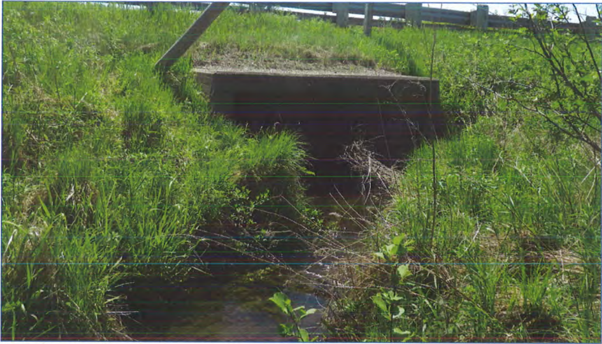
Photo 11: Tributary - view downstream towards entrance of culvert at Highway 136.
