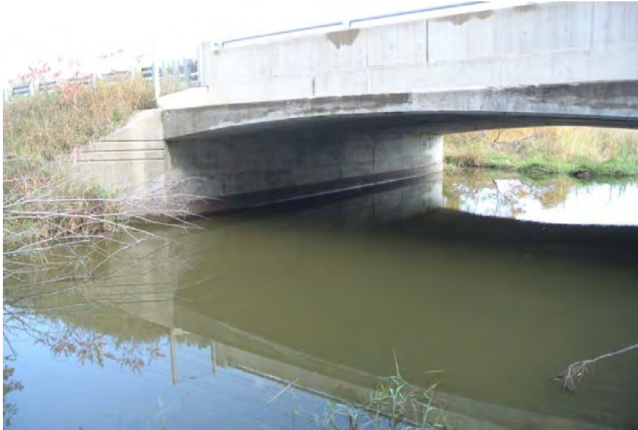
Plate 13: View towards the north abutment, looking northeast.
