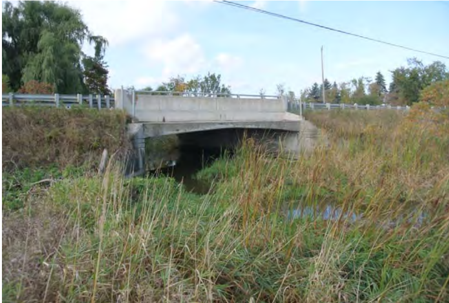
Plate 1: East elevation of the subject bridge, looking northwest.
