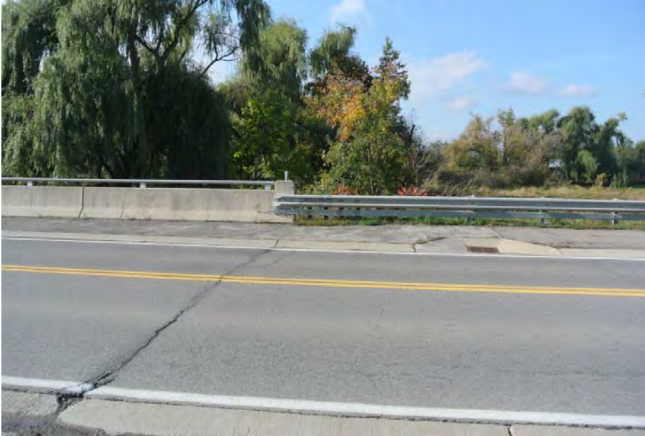
Plate 7: View towards the railing system and metal barrier system located on the west side of the bridge, looking west.
