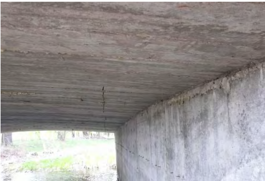
Plate 16: Detail of the bridge soffit and north abutment, looking west.
