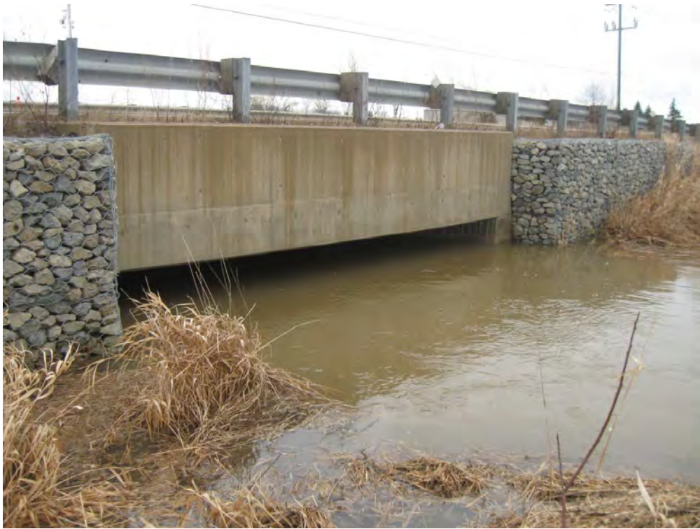
5. Culvert Inlet – East Gabion Retaining Walls
