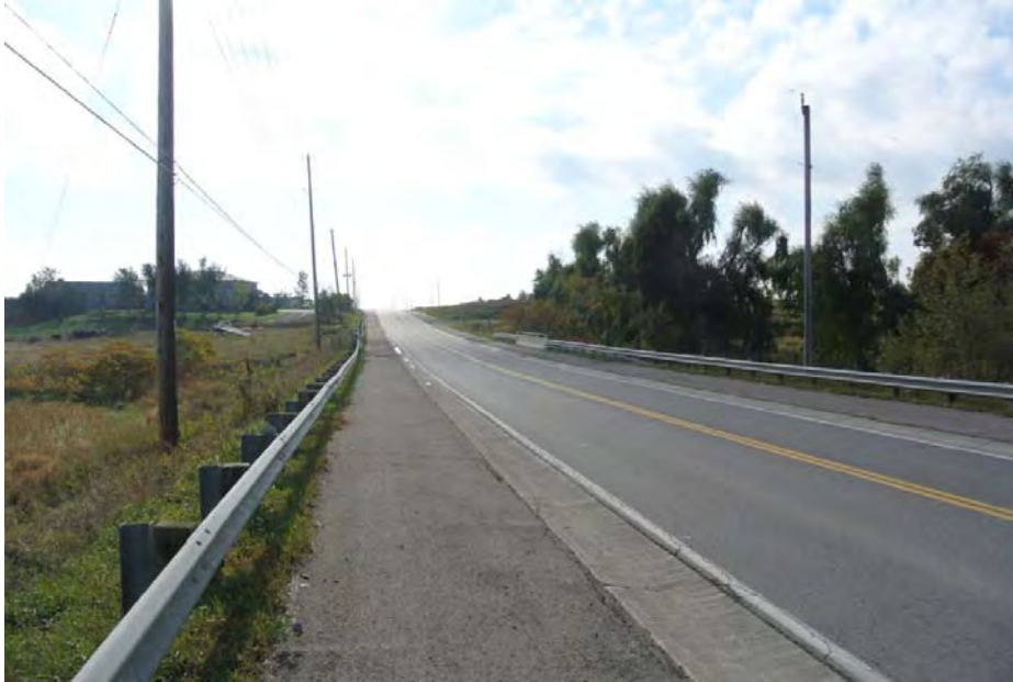
Plate 19: View of the northern approach to the bridge, looking south.
