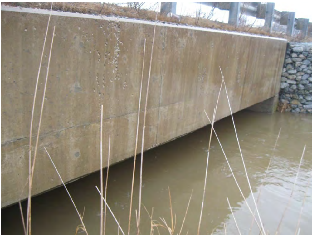
6. Culvert Inlet – East Headwall
