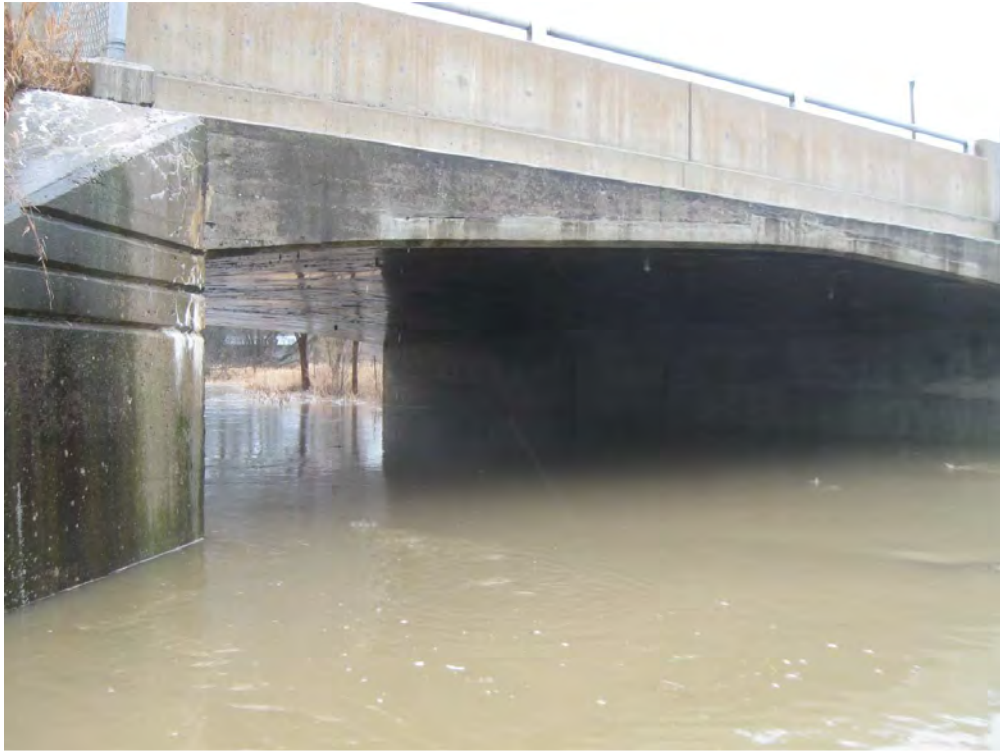
9. Looking West Through Bridge
