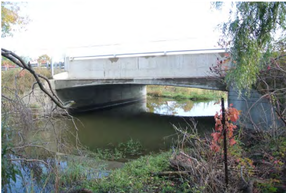
Plate 2: West elevation of the bridge, looking northeast.
