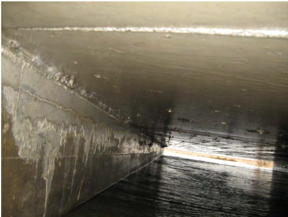
2. Looking West through East Barrel
