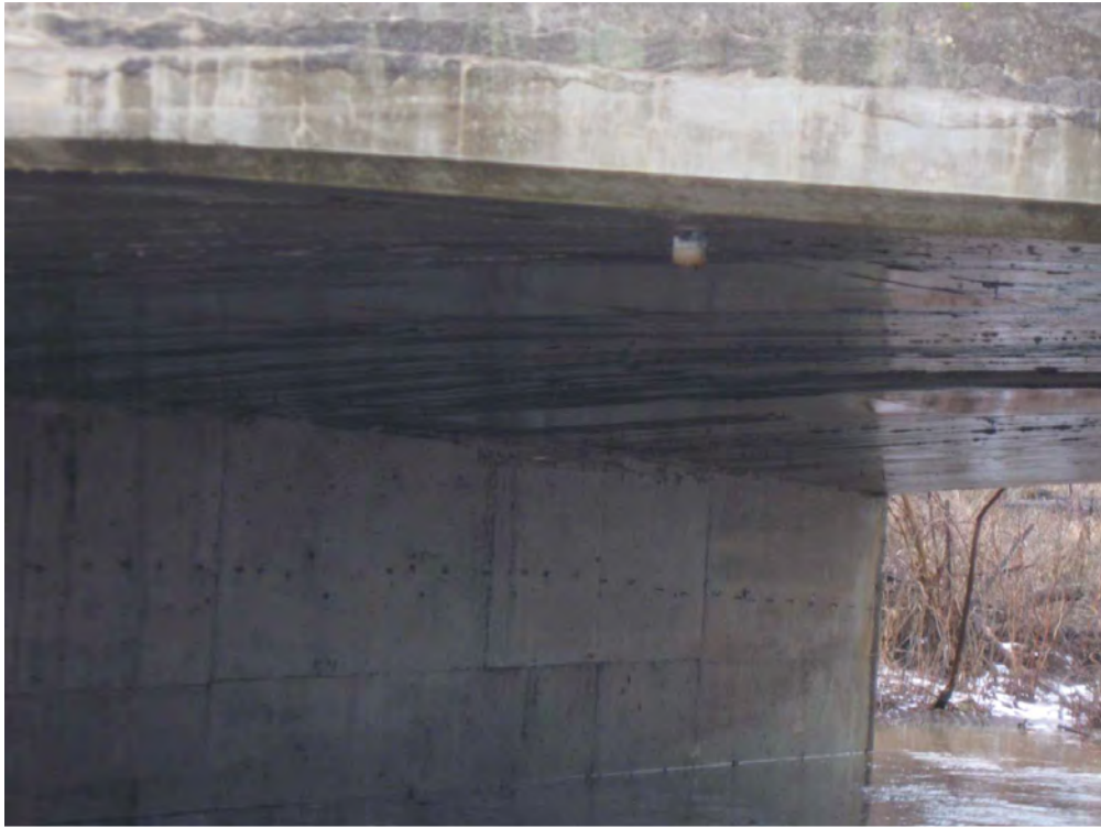
11. Deck Drain in Soffit
