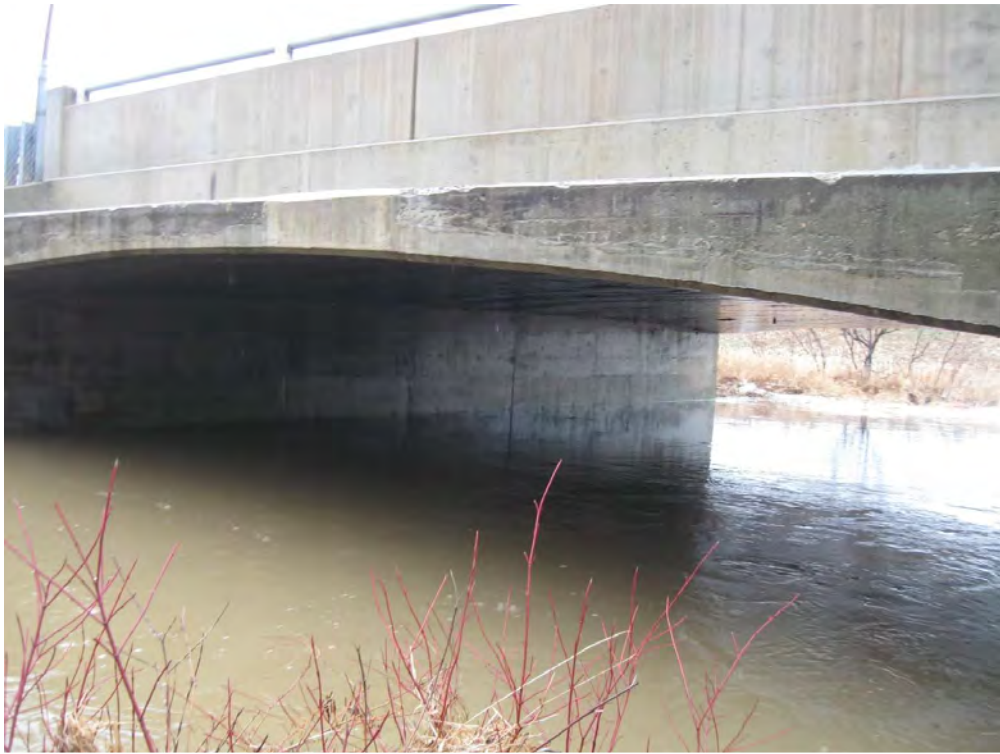
5. Bridge Barrel looking East
