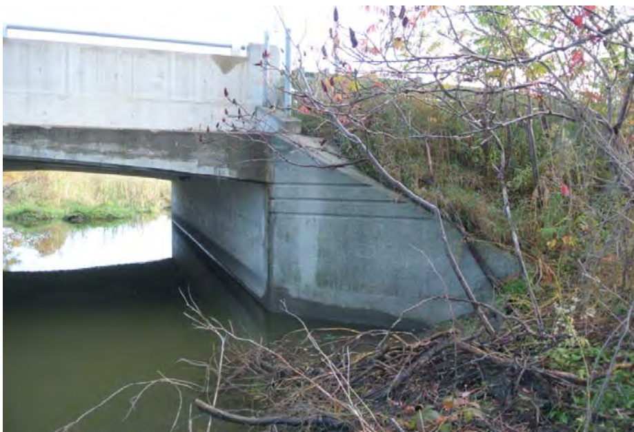
Plate 10: Detail of south abutment, looking east. Note the horizontal fluting on the wingwall.
