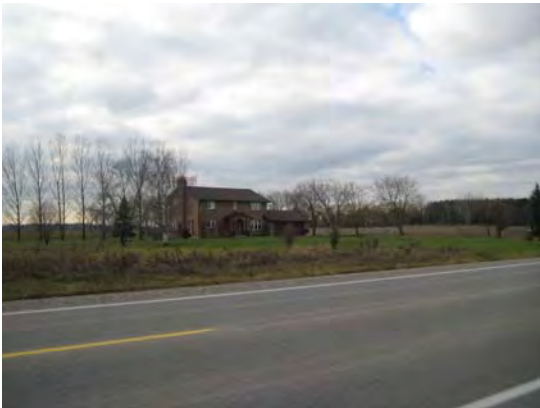
Plate 9: West view across Airport Road. ROW and recent residential development – no potential. Potential in fields adjacent to residential lot.
