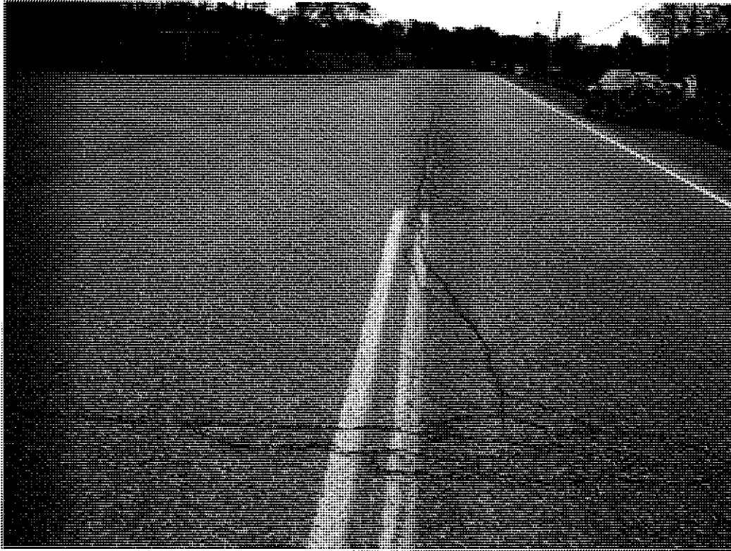
Sta. 0 + 000 approximately looking east.
