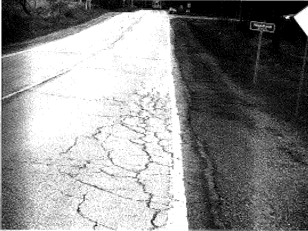
Sta. 41 + 500 approximately looking north.
