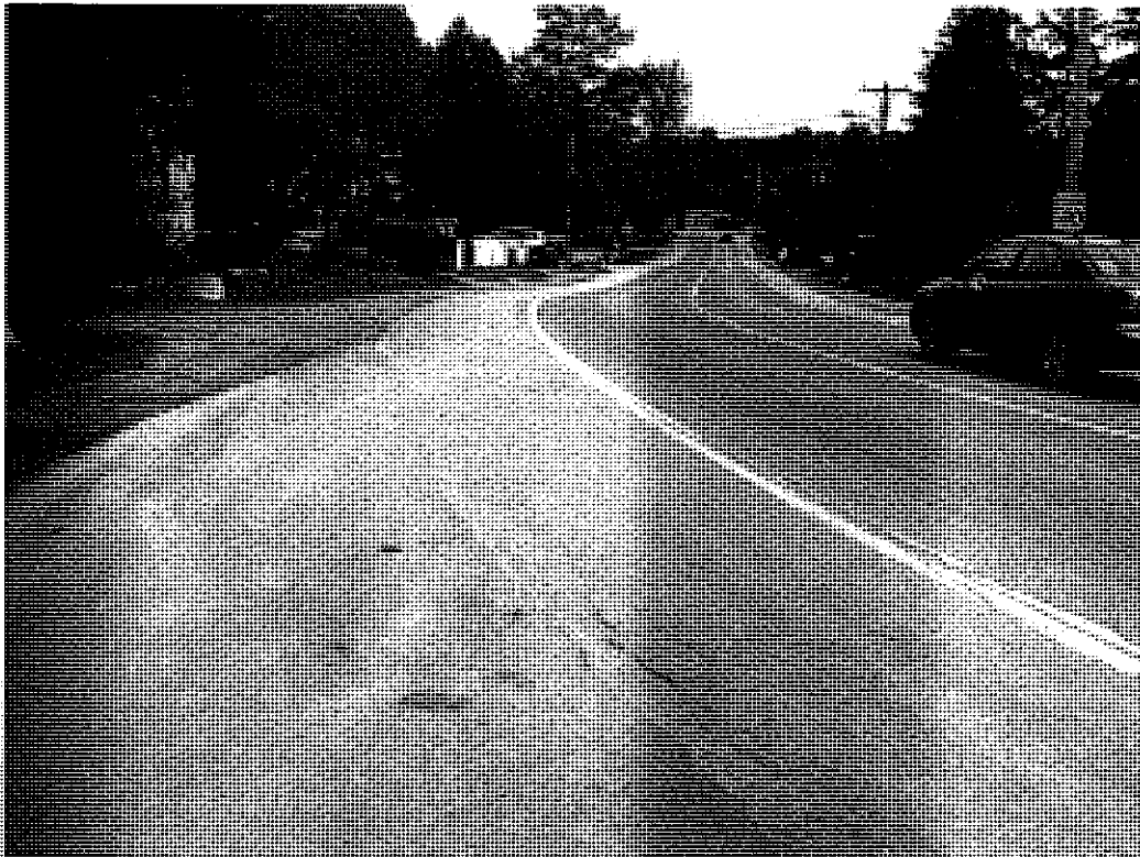
Sta. 42 + 825 approximately looking north.
