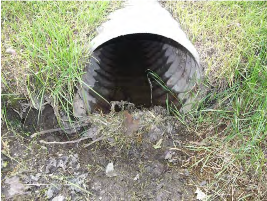
Photo P73 – Additional Culvert#26
