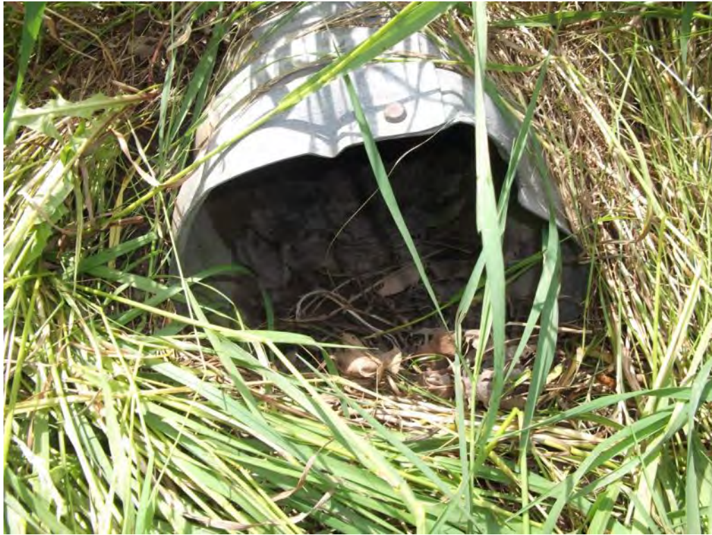
Photo P69 – Additional Culvert#24
