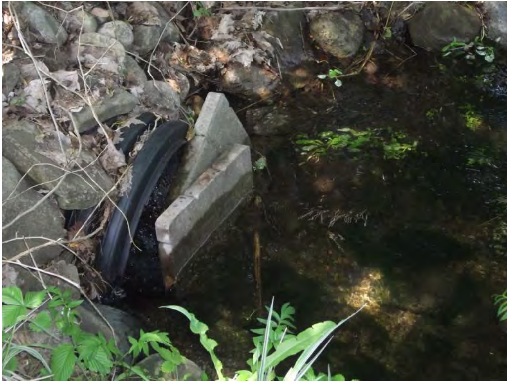
Photo P13 – Additional Culvert # 2
