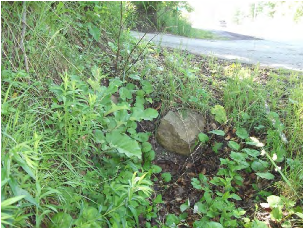
Photo P50 – Additional Culvert#14
