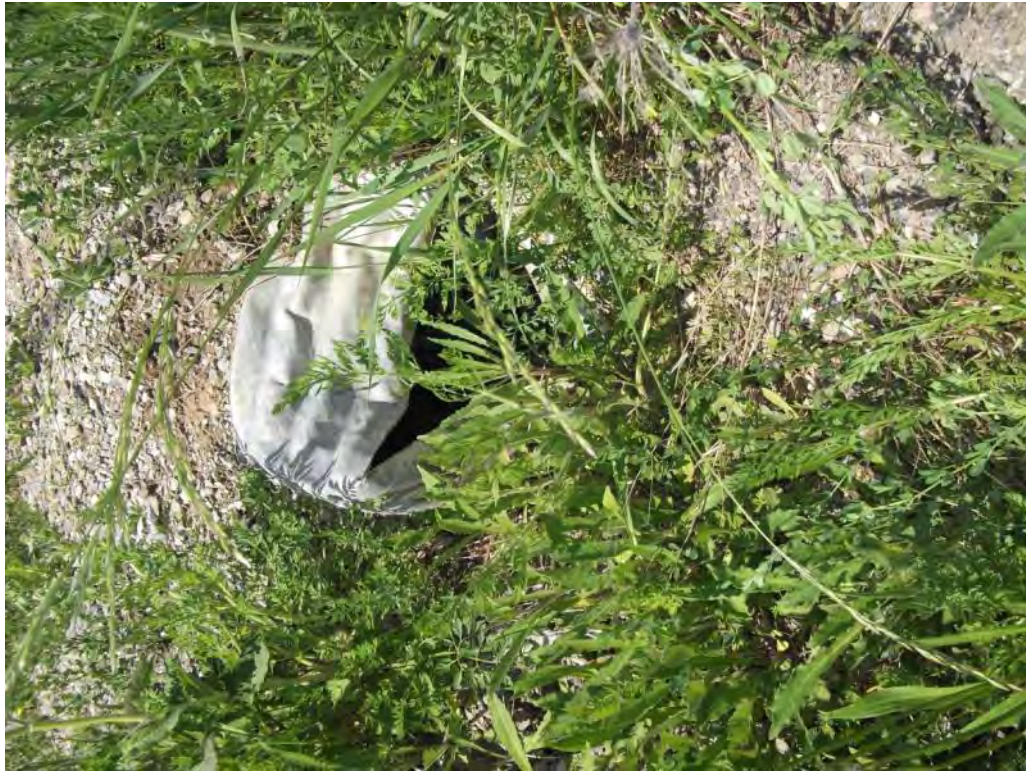
Photo P25 – Additional Culvert#2
