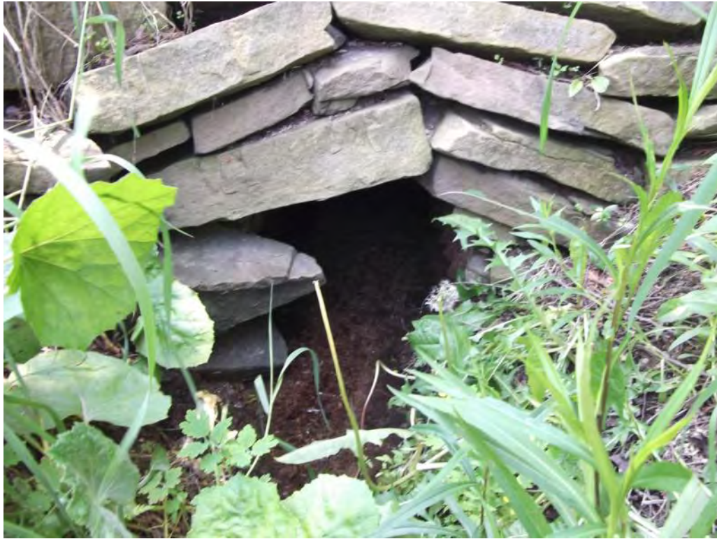
Photo P39 – Additional Culvert#9
