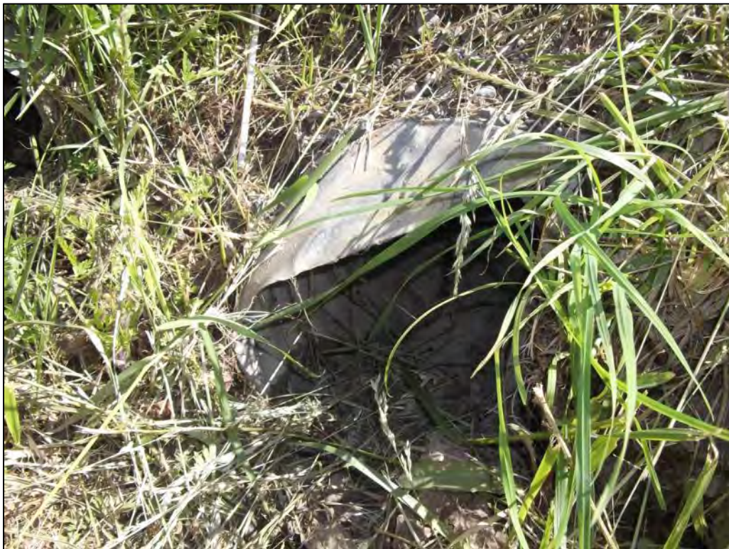
Photo P122 – Additional Culvert#2
