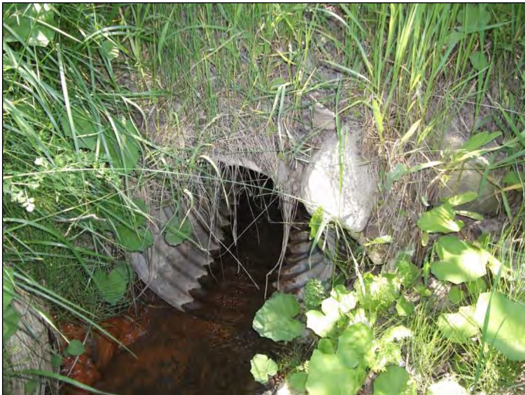
Photo P128 – Additional Culvert#5
