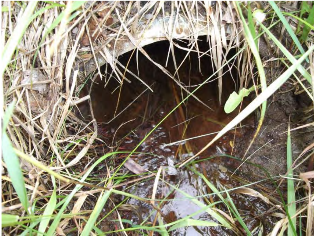
Photo P57 – Additional Culvert#18
