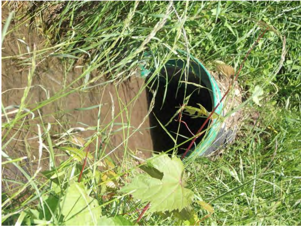
Photo P33 – Additional Culvert#6
