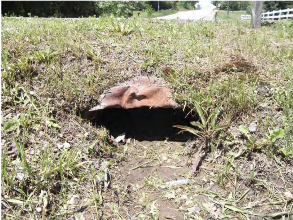
Photo P47 – Additional Culvert#13
