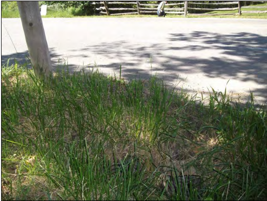
Photo P121 – Additional Culvert#2
