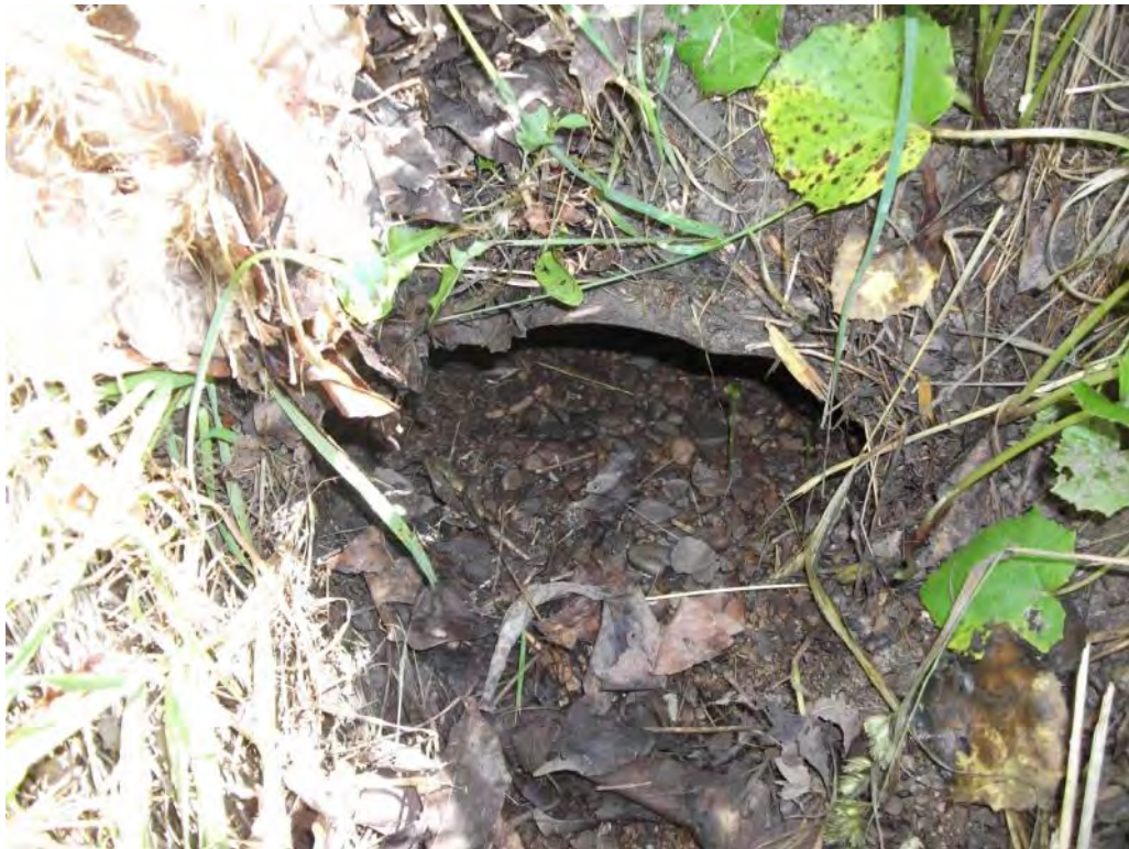
Photo P54 – Additional Culvert#16
