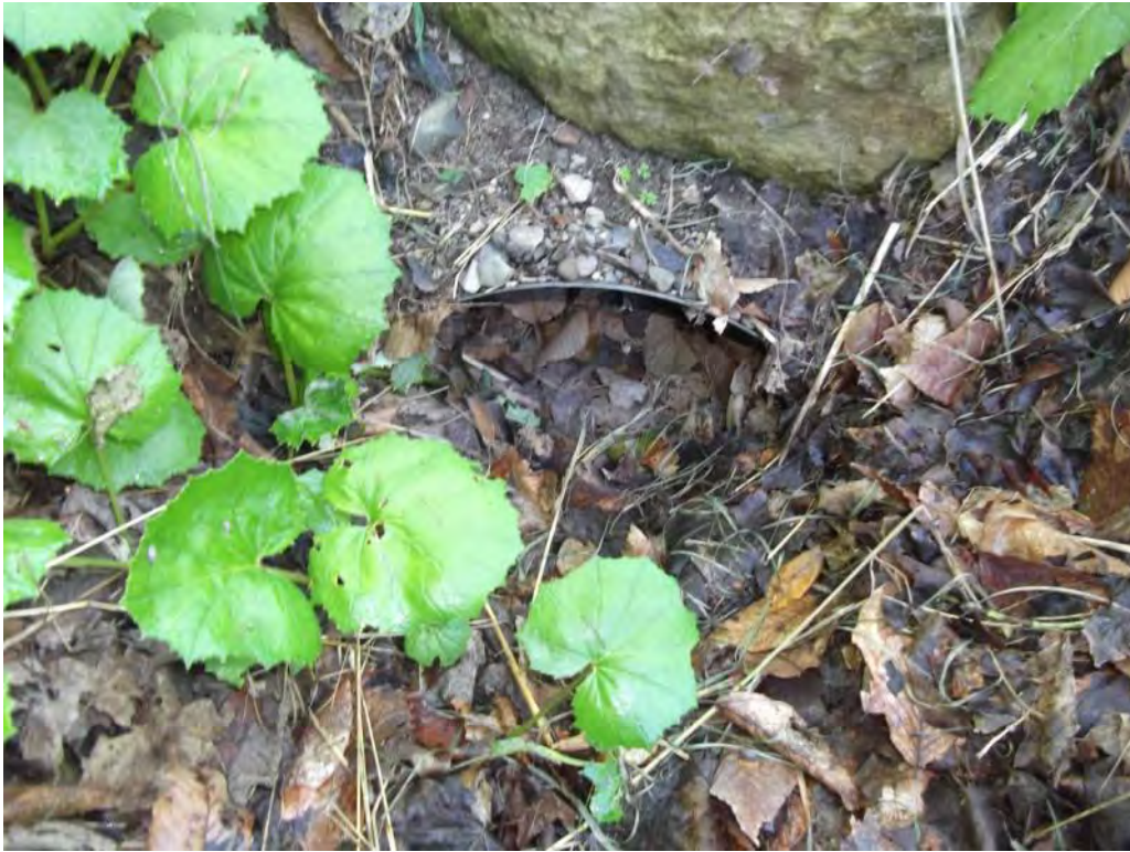
Photo P49 – Additional Culvert#14
