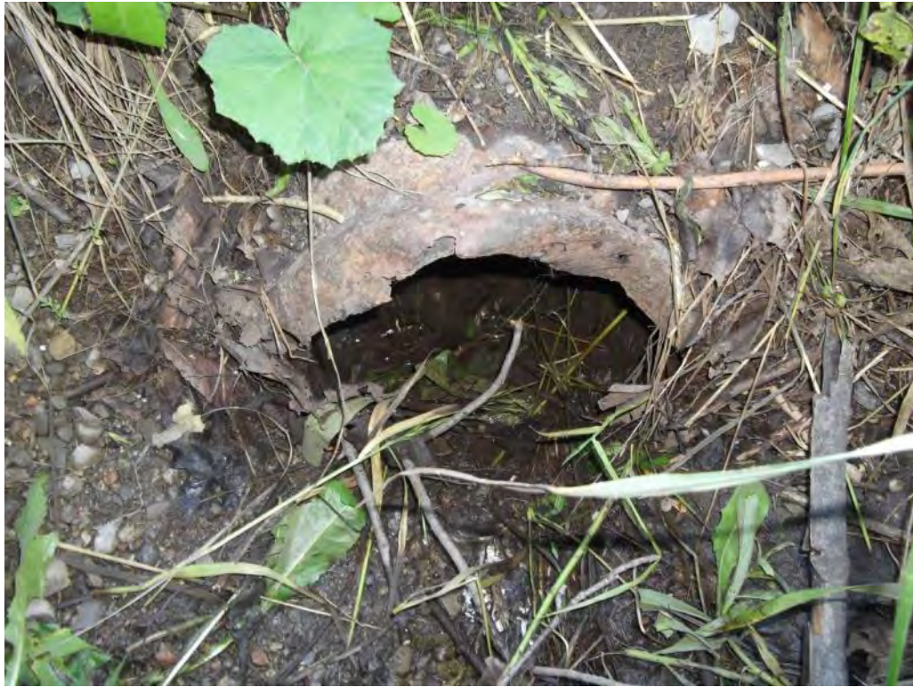
Photo P53 – Additional Culvert#16
