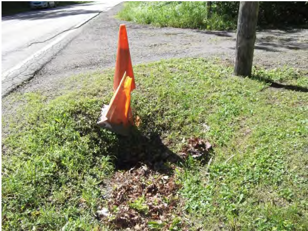
Photo P52 – Additional Culvert#15
