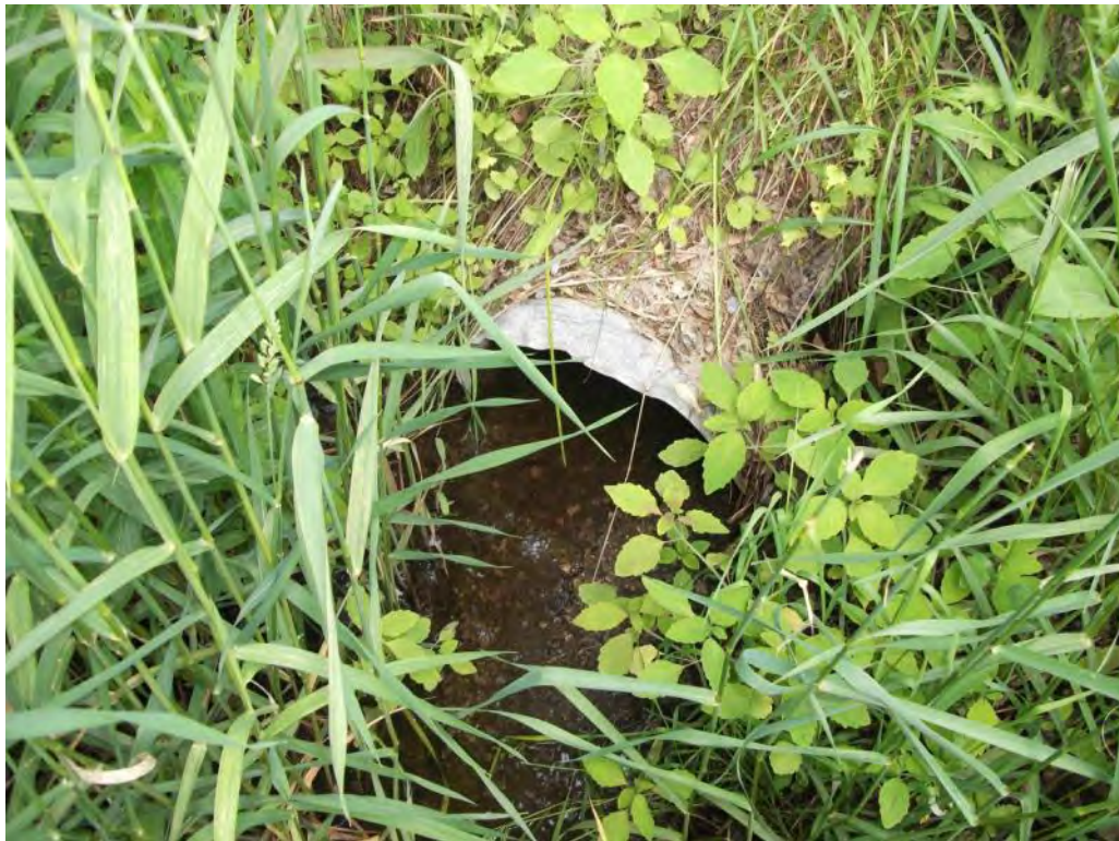
Photo P62 – Additional Culvert#20
