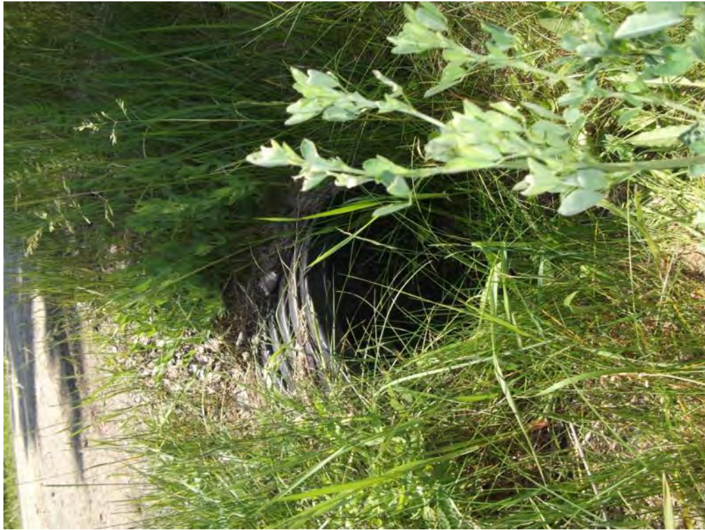
Photo P23 – Additional Culvert#1
