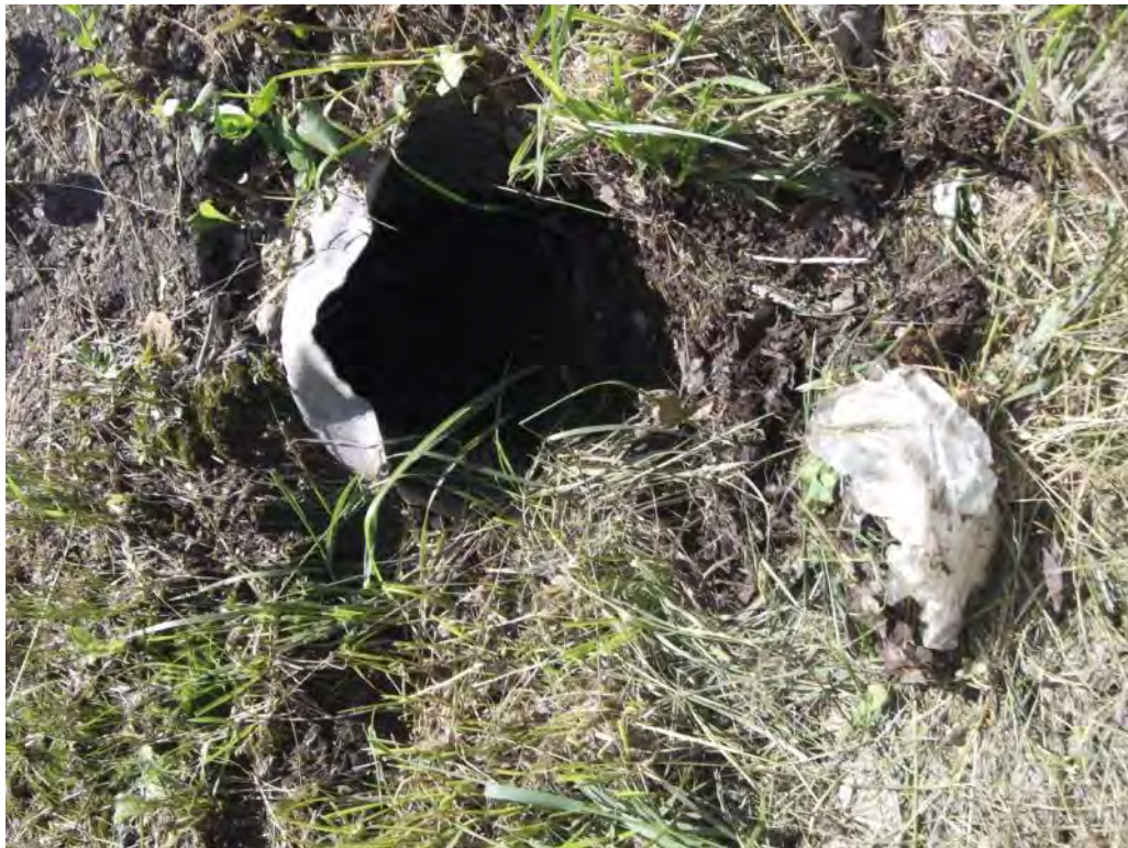
Photo P46 – Additional Culvert#12
