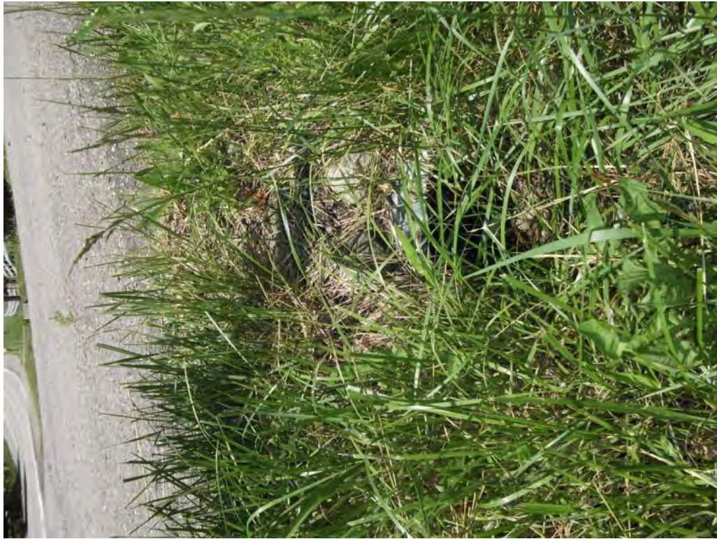
Photo P45 – Additional Culvert#12
