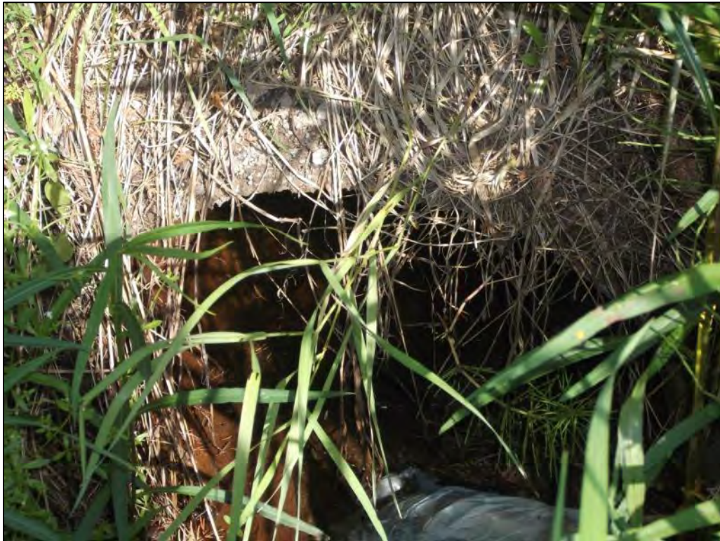
Photo P124 – Additional Culvert#3
