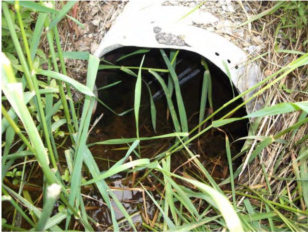
Photo P59 – Additional Culvert#19
