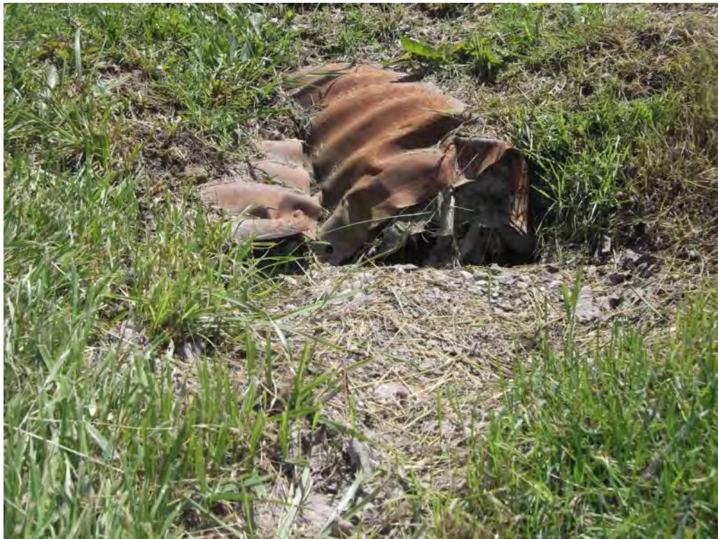
Photo P48 – Additional Culvert#13
