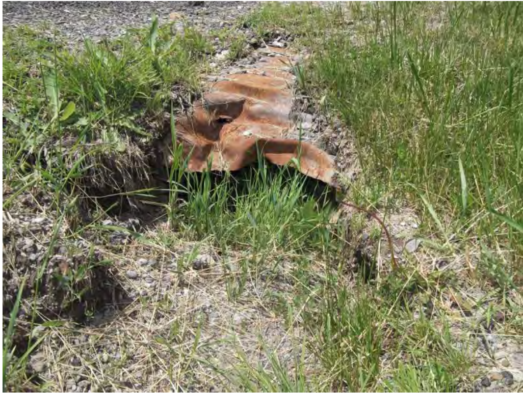
Photo P27 – Additional Culvert#3
