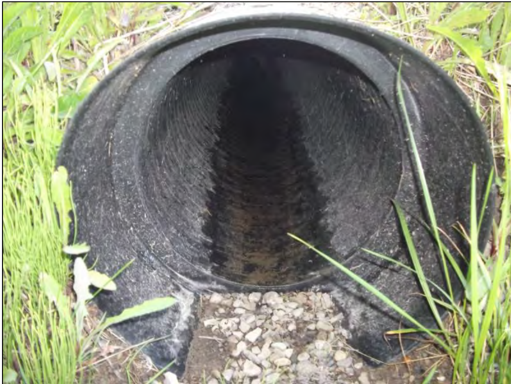
Photo P126 – Additional Culvert#4
