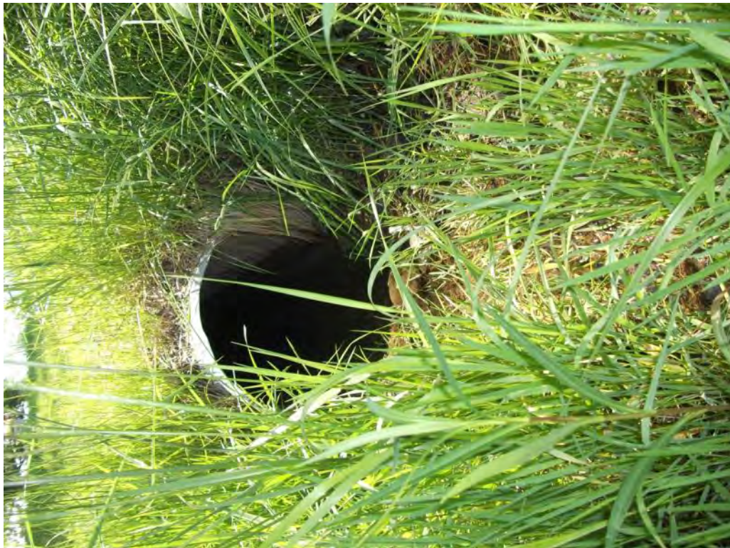
Photo P34 – Additional Culvert#6
