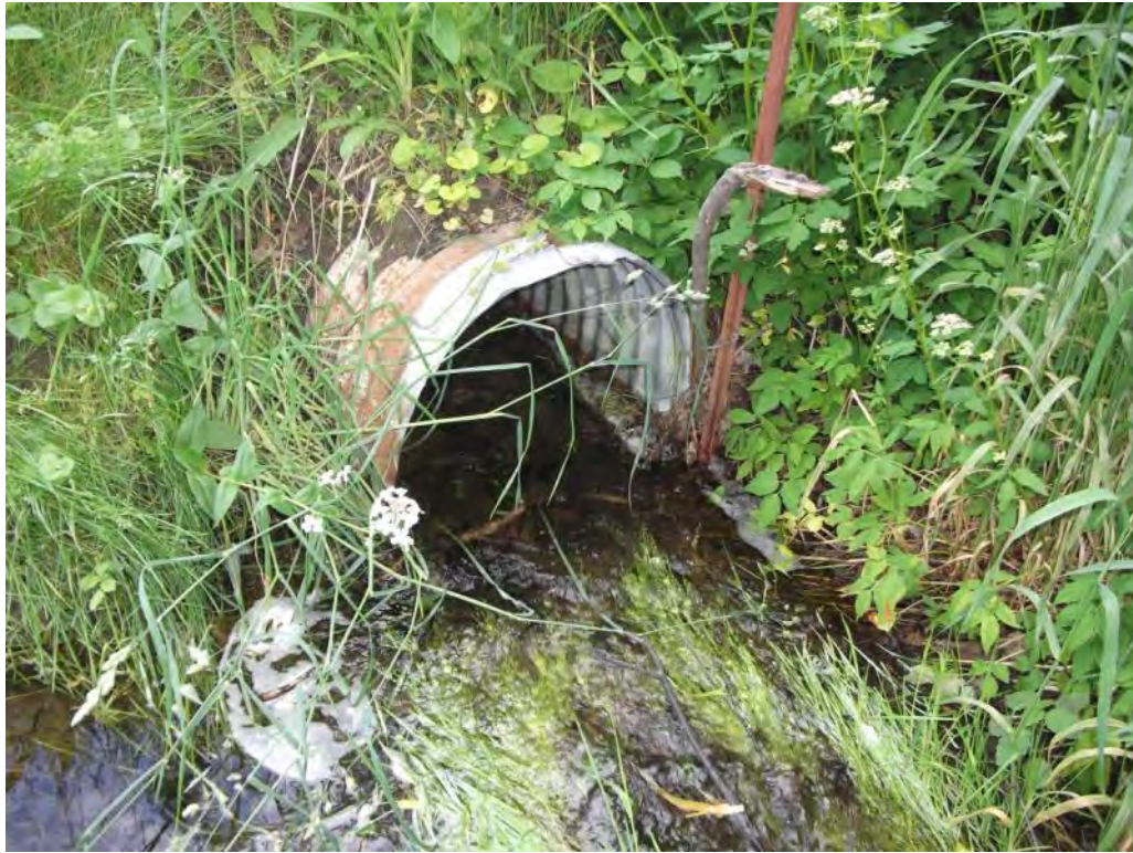
Photo P75 – Additional Culvert#27
