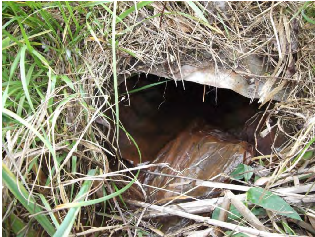
Photo P58 – Additional Culvert#18
