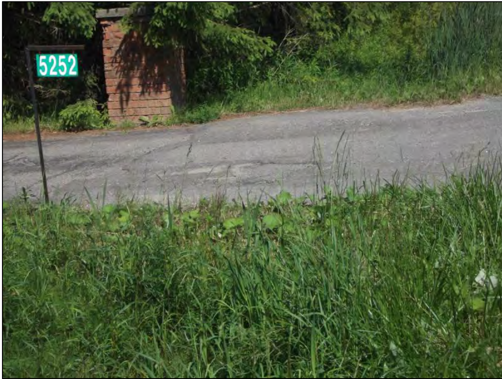
Photo P123 – Additional Culvert#3
