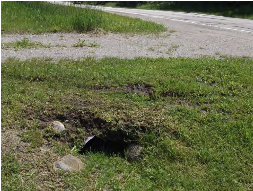
Photo P32 – Additional Culvert#5
