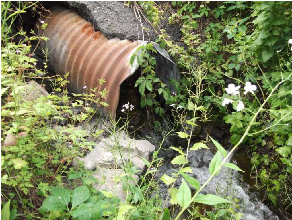
Photo P76 – Additional Culvert#27
