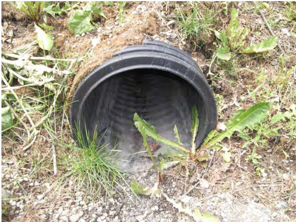
Photo P72 – Additional Culvert#25
