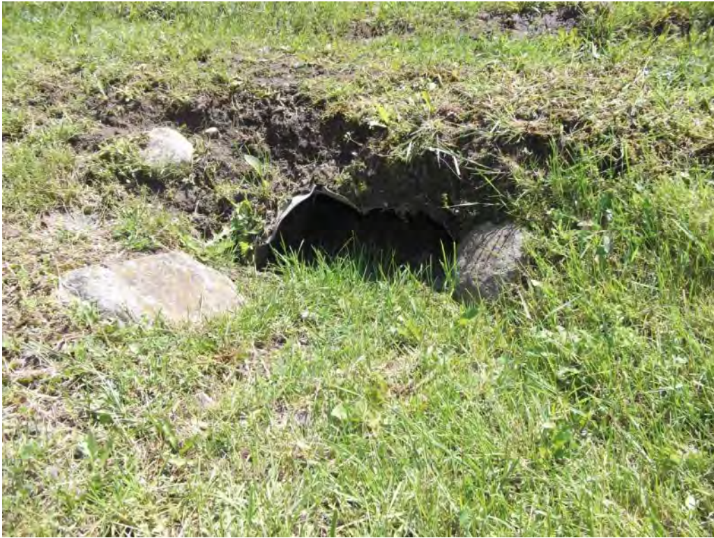
Photo P31 – Additional Culvert#5
