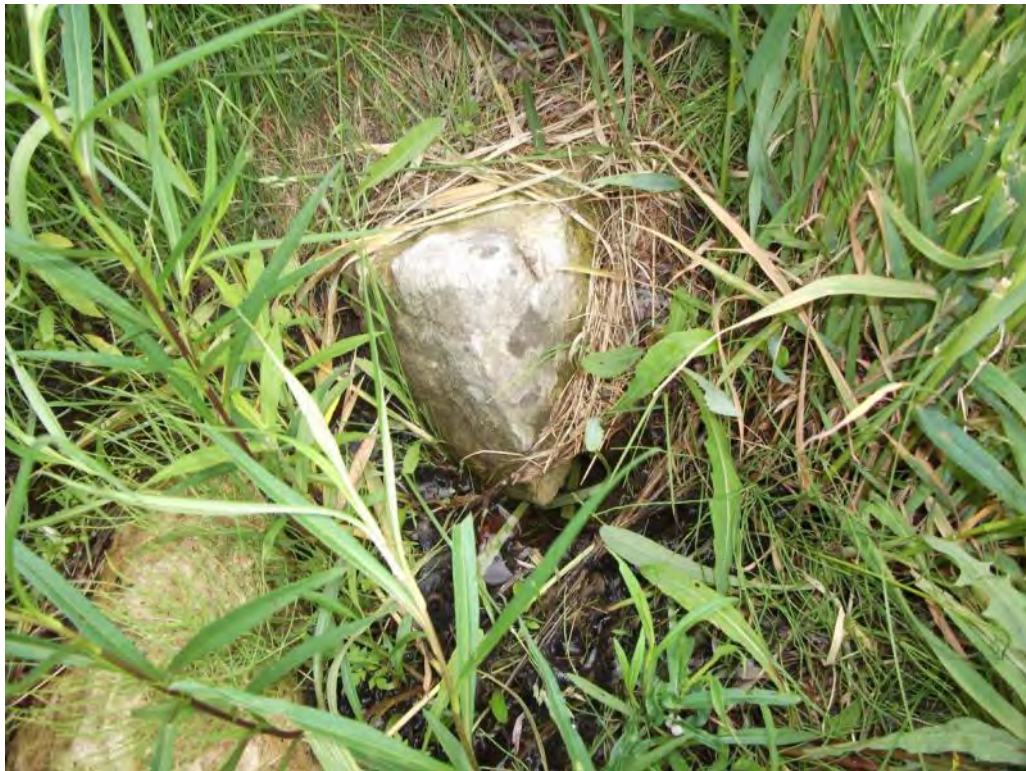
Photo P64 – Additional Culvert#21
