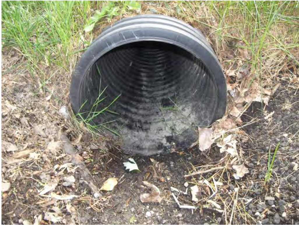
Photo P71 – Additional Culvert#25
