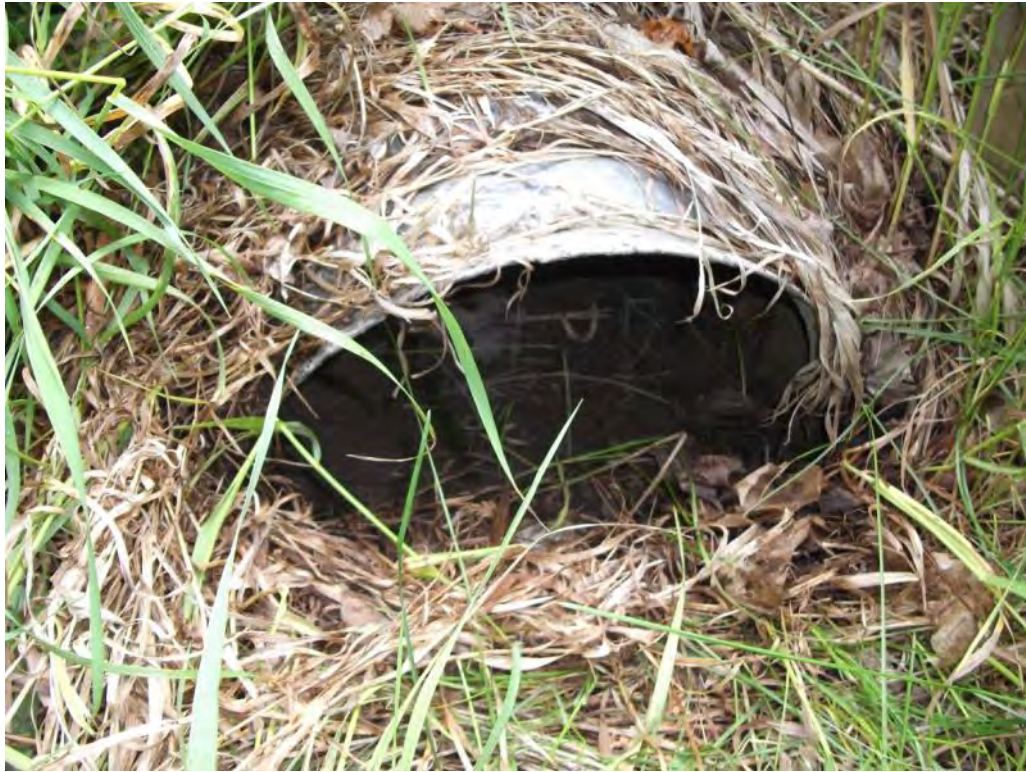
Photo P67 – Additional Culvert#23
