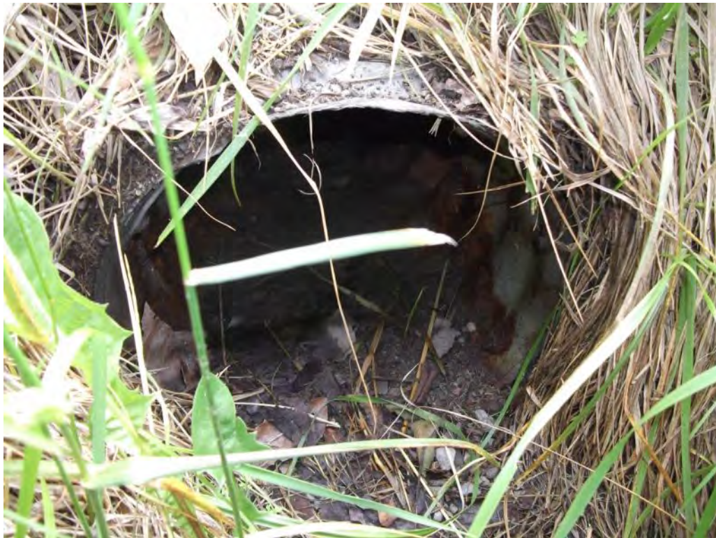
Photo P56 – Additional Culvert#17
