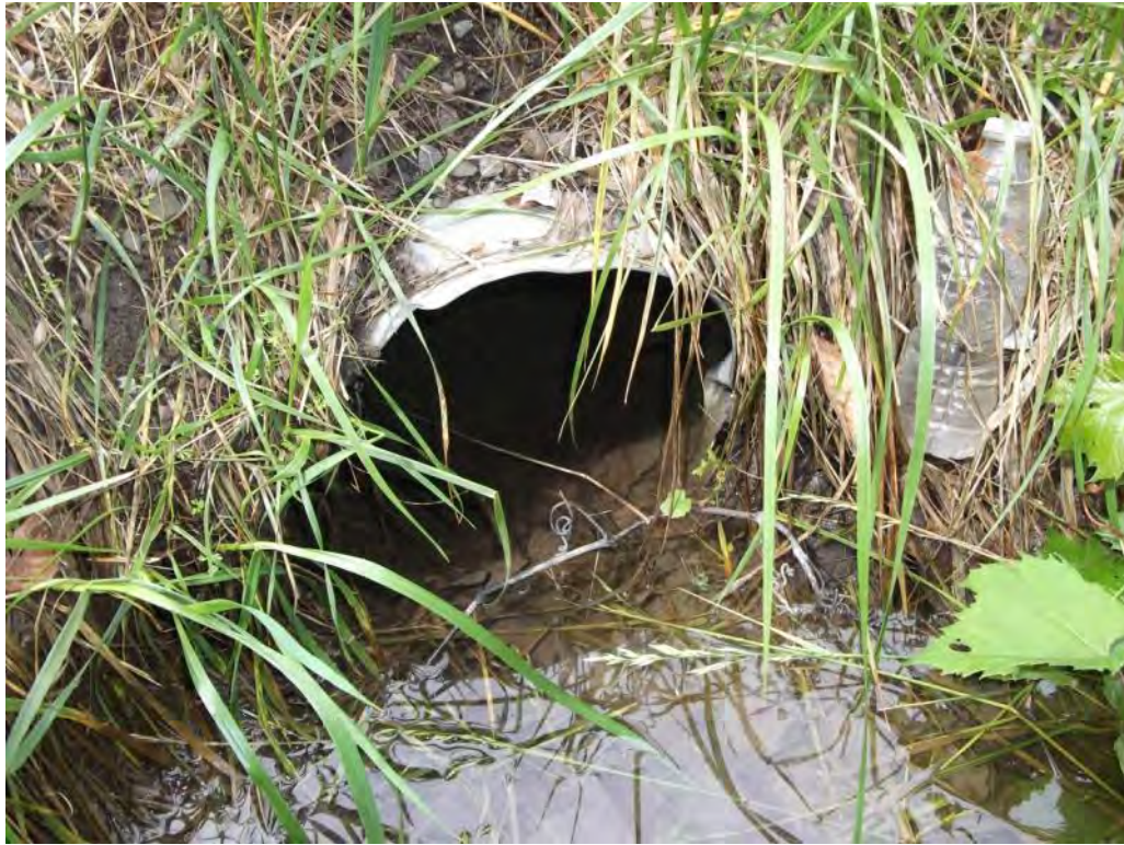
Photo P55 – Additional Culvert#17
