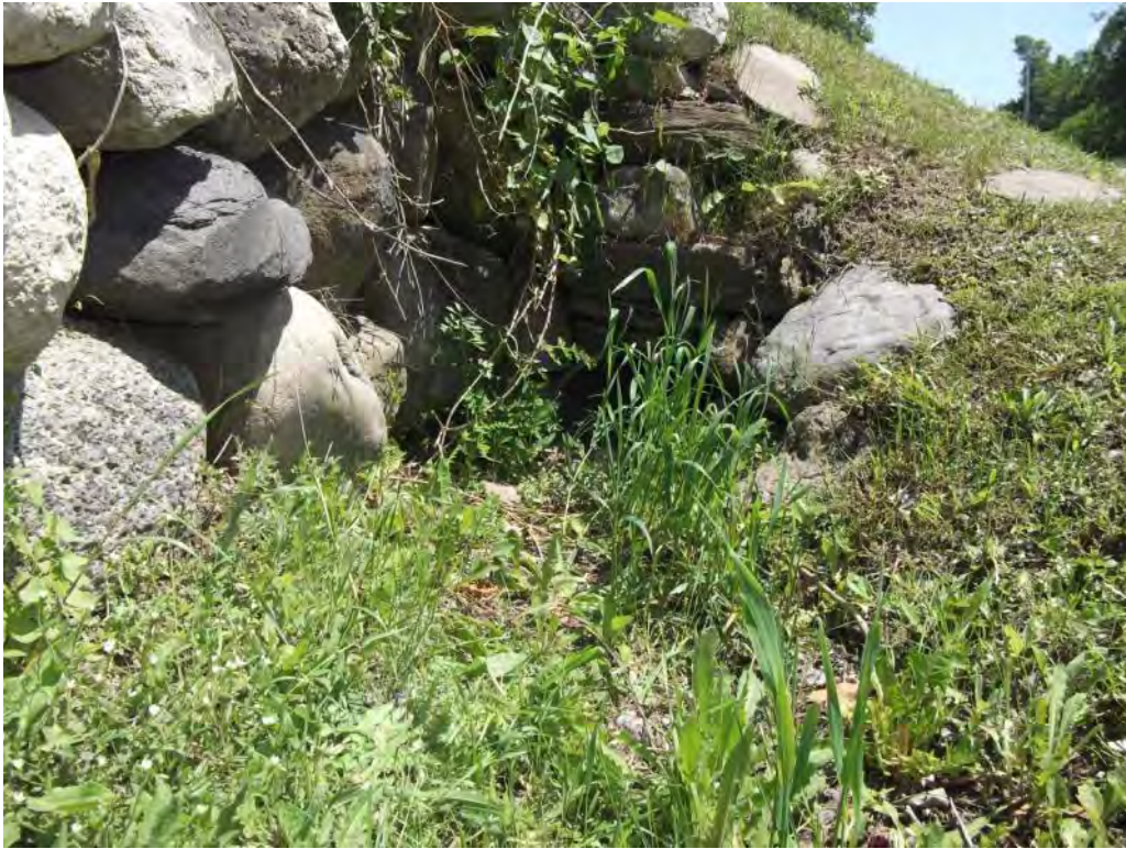
Photo P29 – Additional Culvert#4
