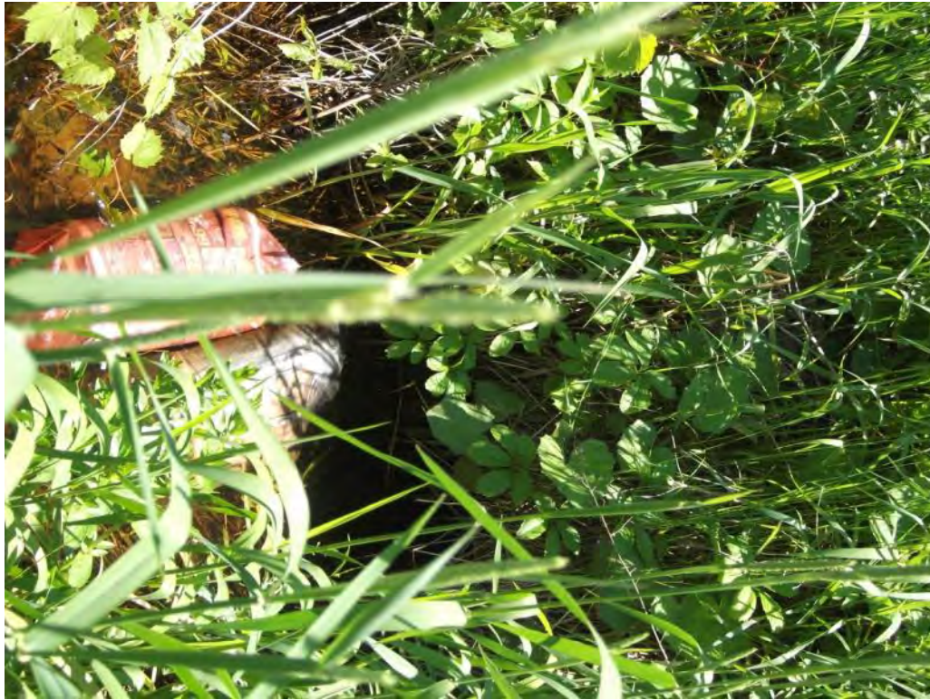
Photo P41 – Additional Culvert#10
