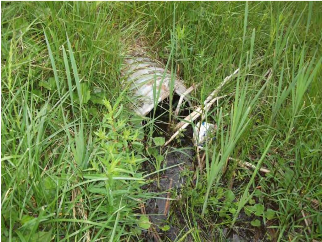
Photo P66 – Additional Culvert#22
