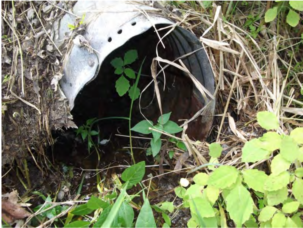
Photo P61 – Additional Culvert#20
