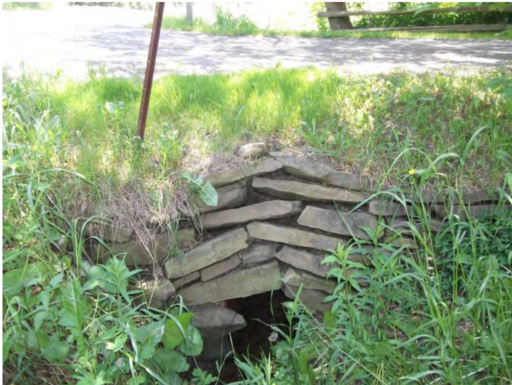
Photo P40 – Additional Culvert#9
