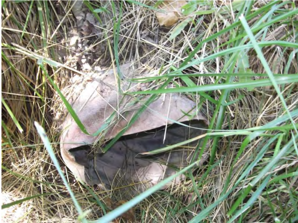
Photo P119 – Additional Culvert#1
