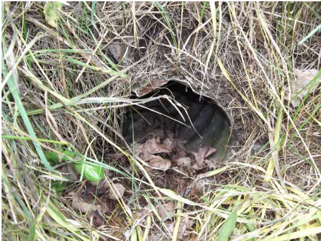
Photo P68 – Additional Culvert#23
