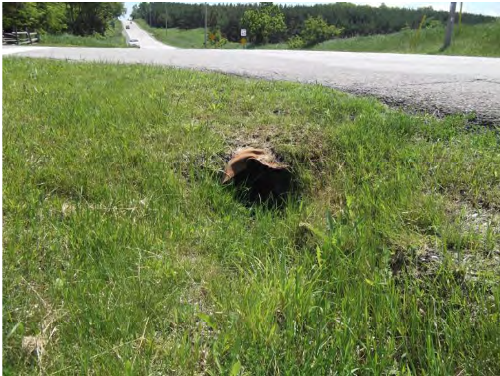
Photo P28 – Additional Culvert#3
