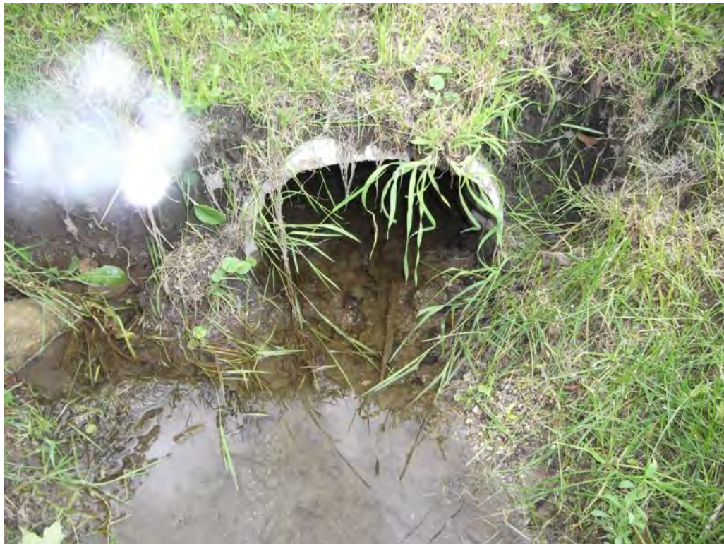
Photo P74 – Additional Culvert#26
