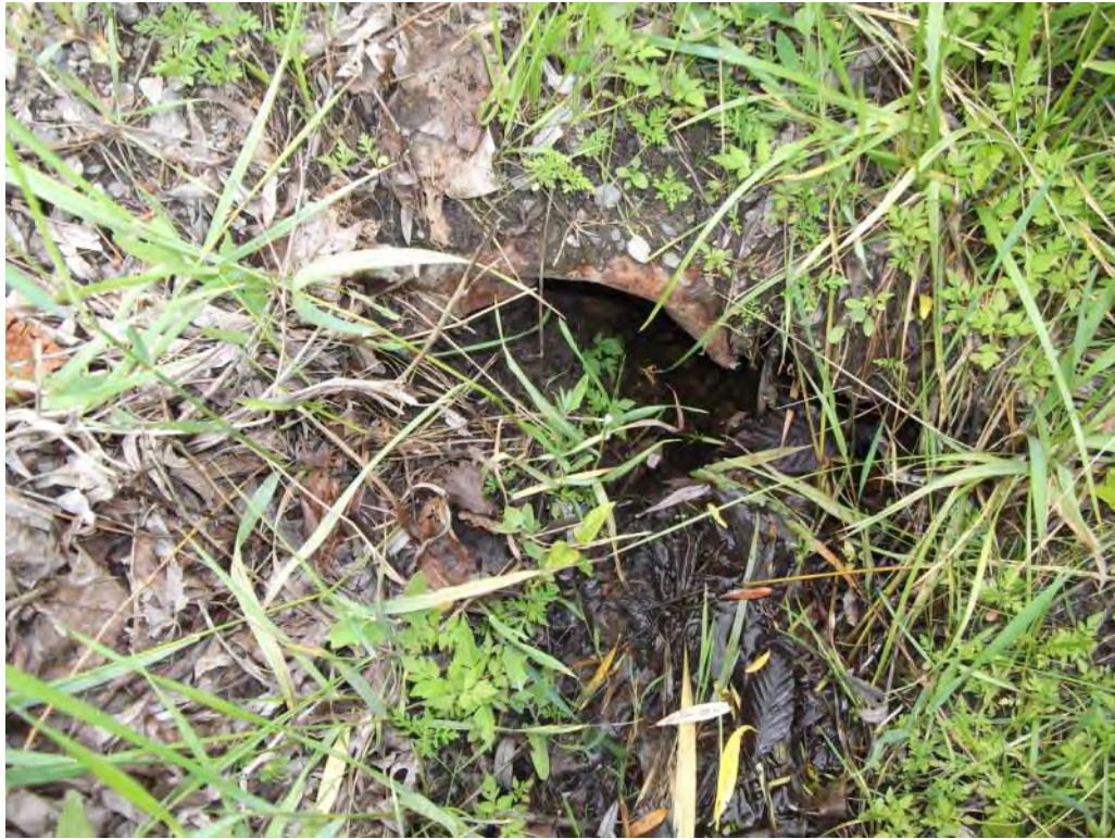
Photo P63 – Additional Culvert#21
