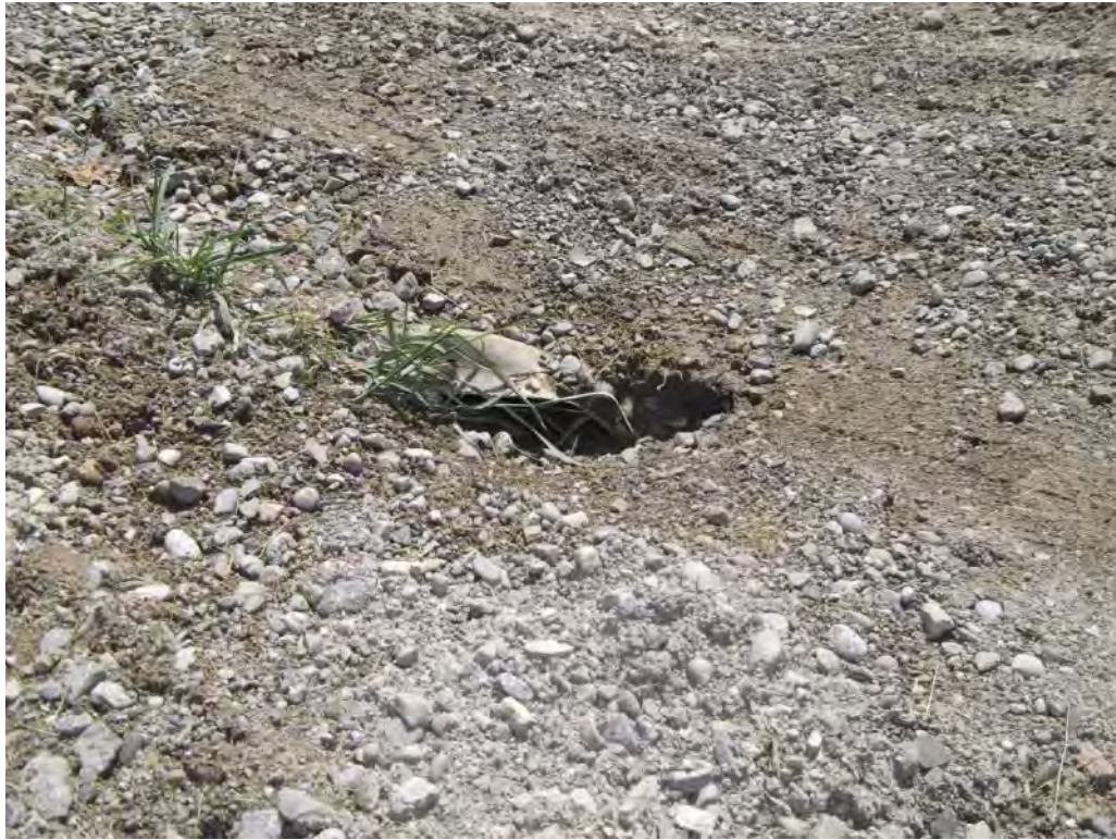
Photo P43 – Additional Culvert#11
