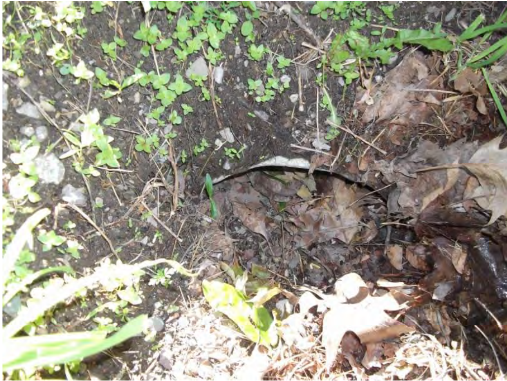
Photo P51 – Additional Culvert#15
