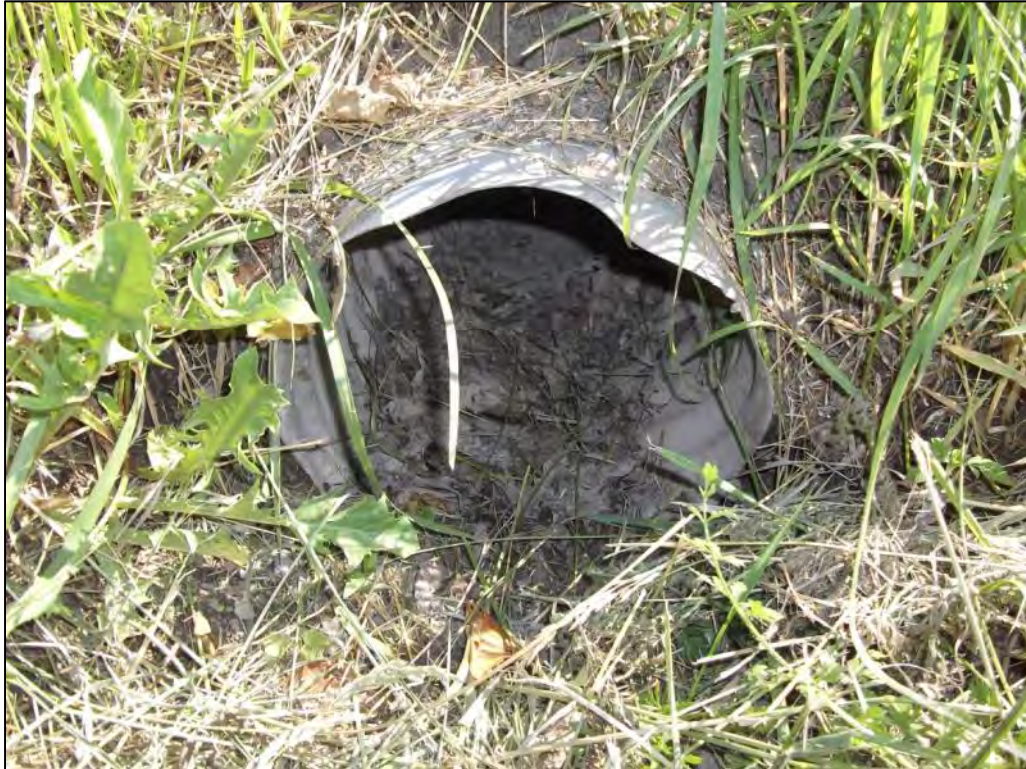
Photo P120 – Additional Culvert#1
