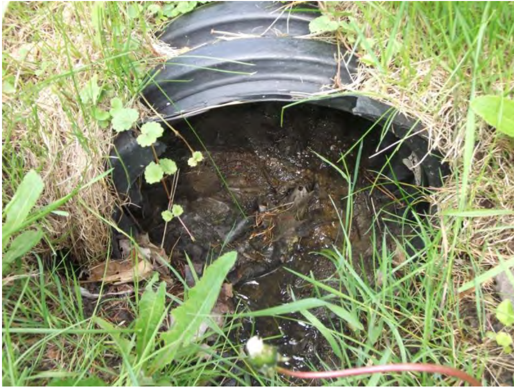
Photo P11 – Additional Culvert # 1
