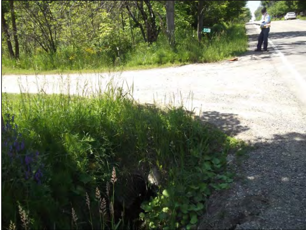
Photo P127 – Additional Culvert#5
