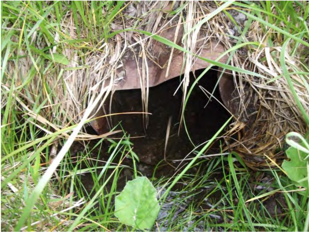
Photo P65 – Additional Culvert#22
