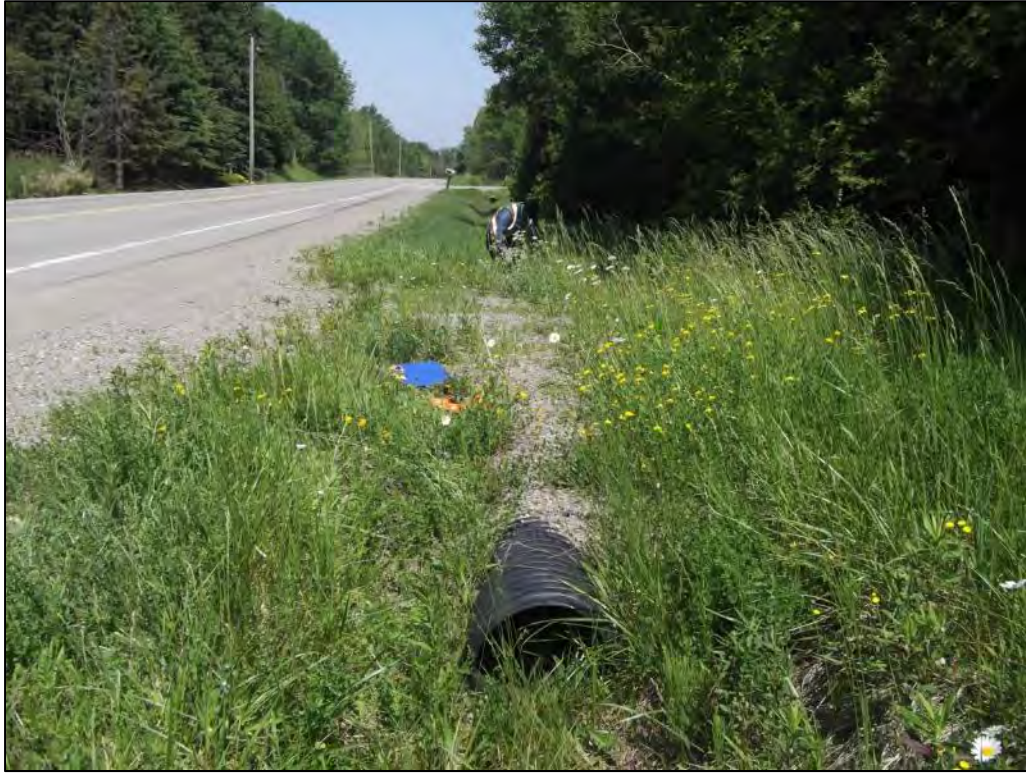
Photo P125 – Additional Culvert#4
