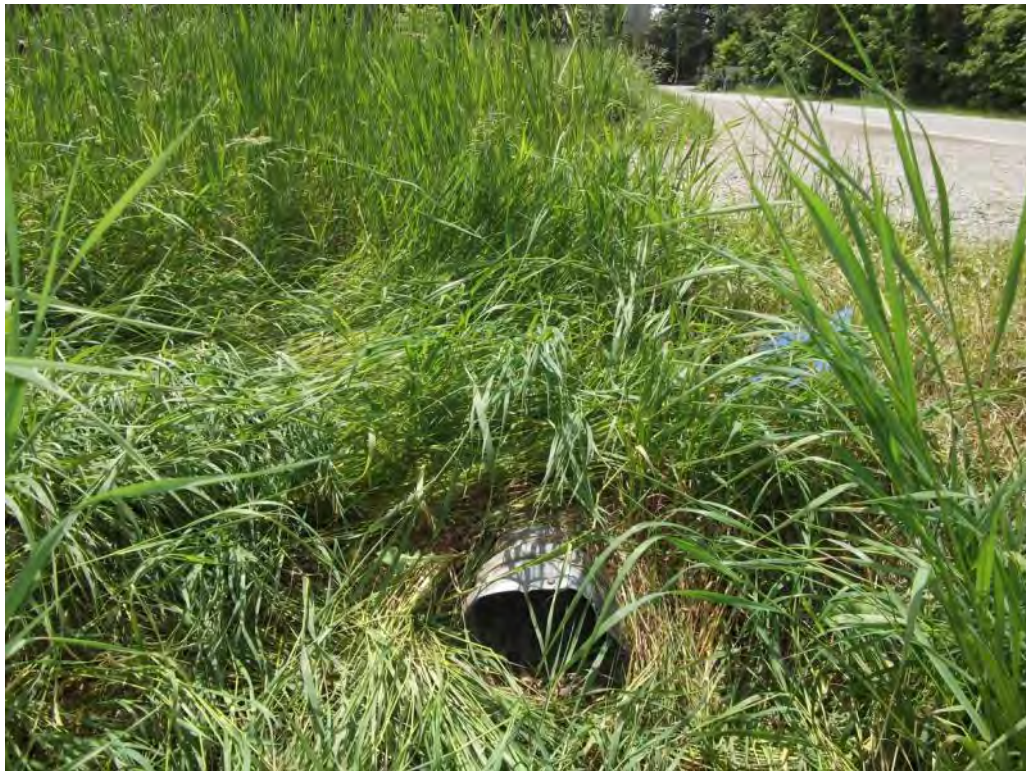
Photo P70 – Additional Culvert#24
