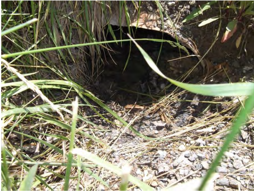
Photo P35 – Additional Culvert#7
