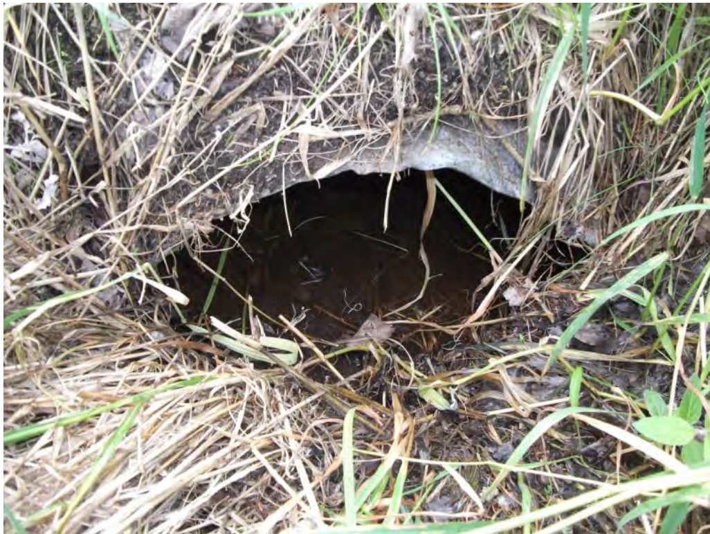
Photo P60 – Additional Culvert#19
