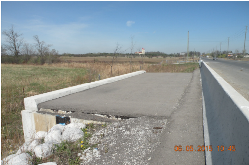
Extension and Header Wall on West Side
