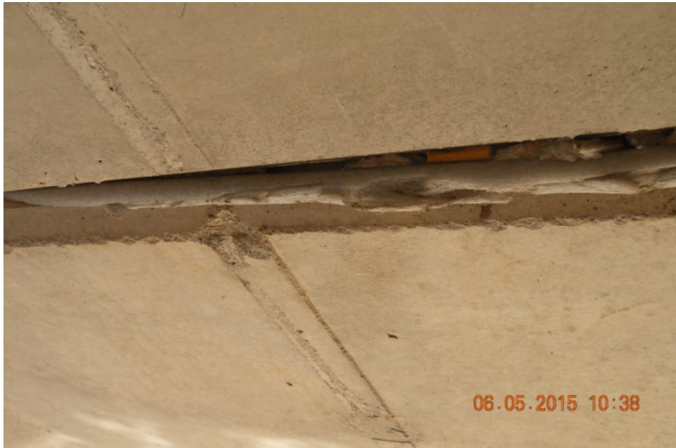
Form at Joint (several joints near East End)
