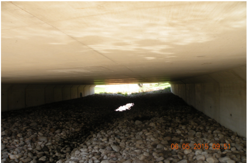
Looking West Under Structure
