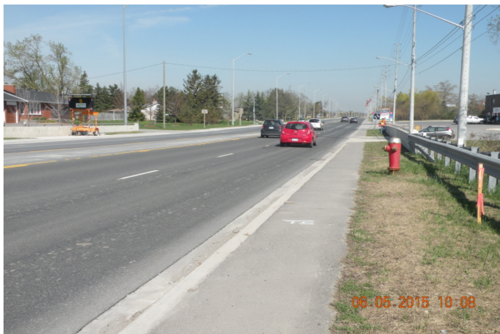
Looking North at Bridge
