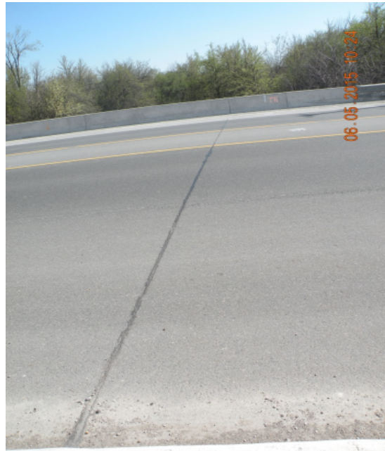
Deck Slab Joint (Typical)
