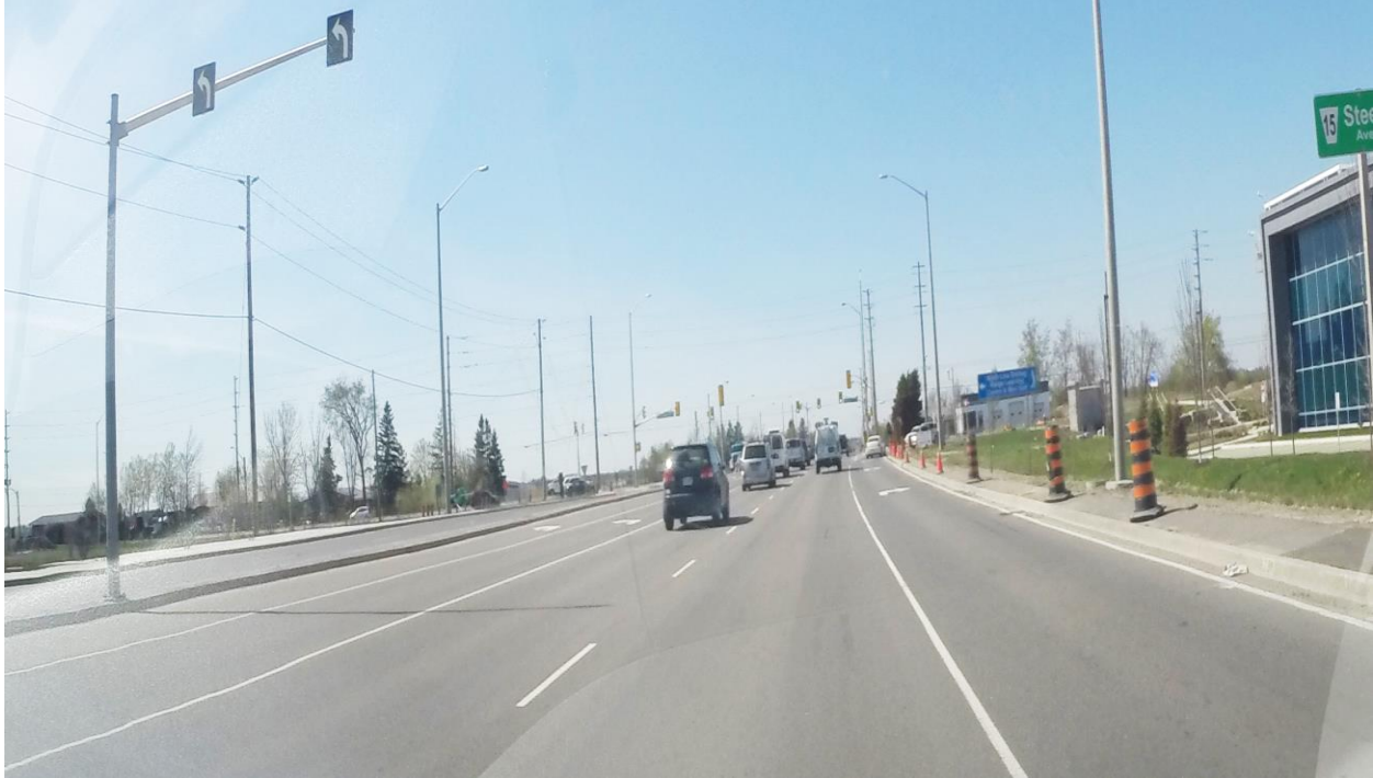
Typical Photograph #1 Winston Churchill Boulevard Northbound at Station 0+944 (Looking Northerly)
