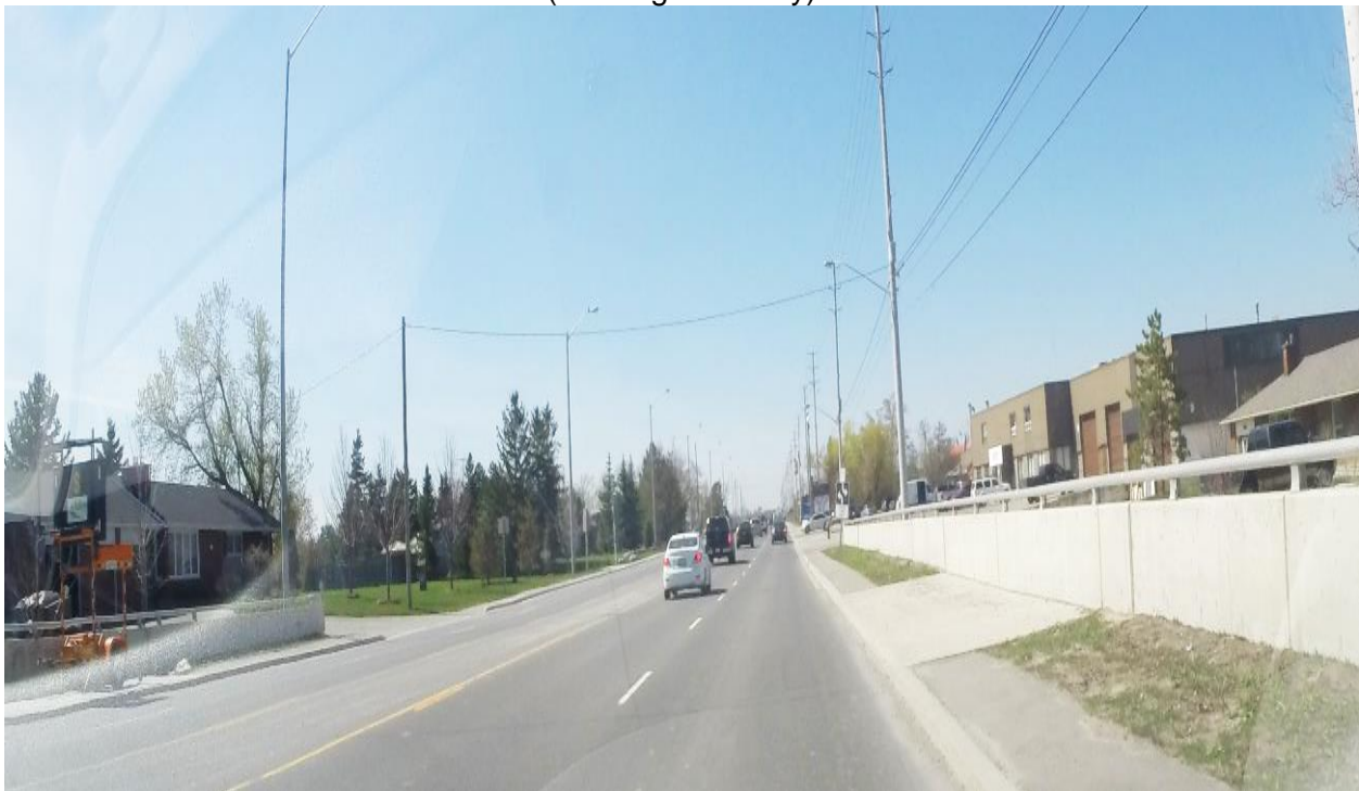
Typical Photograph #2 Winston Churchill Boulevard Northbound at Station 1+400 (Looking Northerly)
