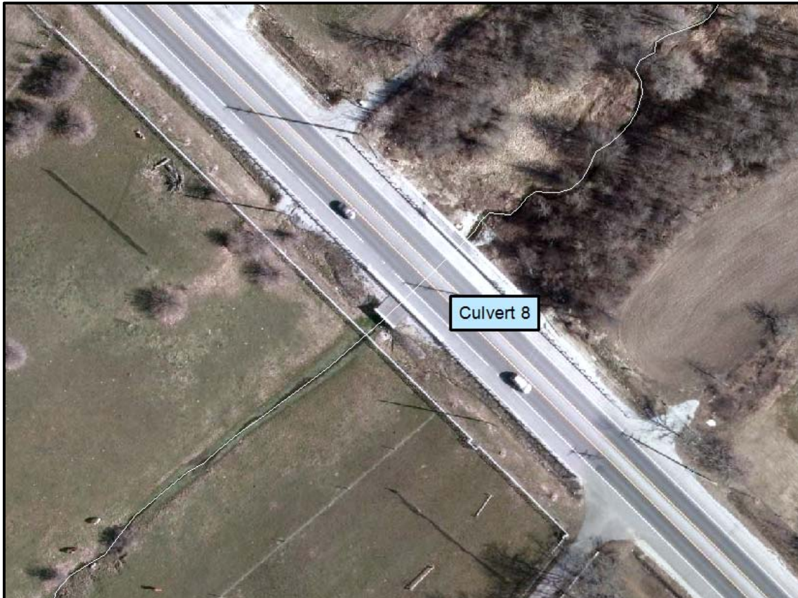
Figure 4: Aerial View of Cu-8 on Levi Creek South
