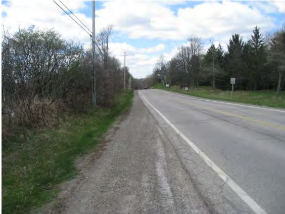
Plate 13: View northwest along Mississauga Rd. Undisturbed land is present on either side of ROW.
