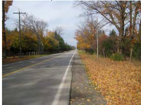
Plate 10: Northwest view along Winston Churchill Boulevard. ROW is disturbed – no potential. Potential on both sides of road beyond ROW.
