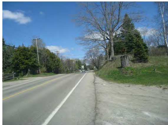
Plate 22: View northeast along Bush St. ROW. Note wide gravel shoulders. Lands adjacent to ROW are sloping or low/wet.
