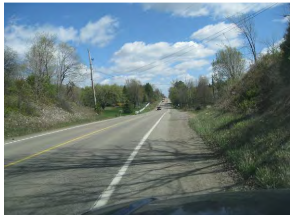
Plate 12: View southeast along Mississauga Rd. Note steep slope adjacent to ROW.
