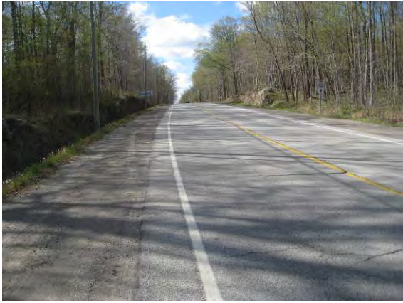
Plate 1: View northwest along Mississauga Rd. Lands adjacent to ROW consists of rocky, uneven ground.
