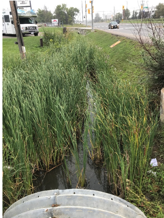
FIGURE 10 Culvert 4 Looking Downstream
