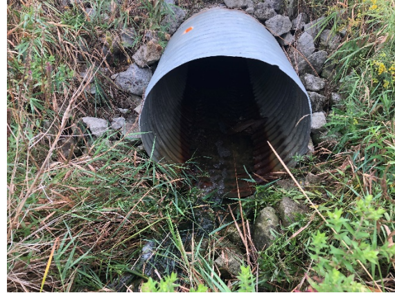
FIGURE 2 Culvert 1A Upstream End
