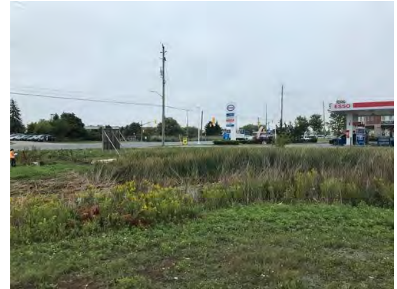
3. Upstream of Culvert 1
