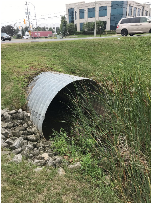
FIGURE 9 Culvert 4 Upstream End
