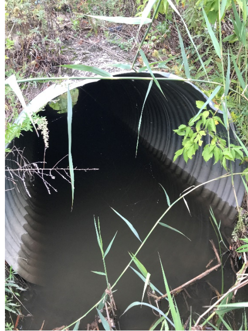
FIGURE 6 Culvert 2 Downstream End
