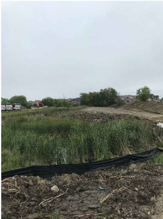
FIGURE 19 Current Channel Realignment Looking Upstream
