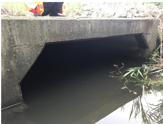
FIGURE 3 Culvert 1 Downstream End
