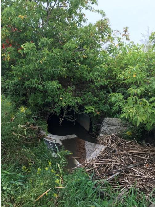
FIGURE 5 Culvert 2 Upstream End
