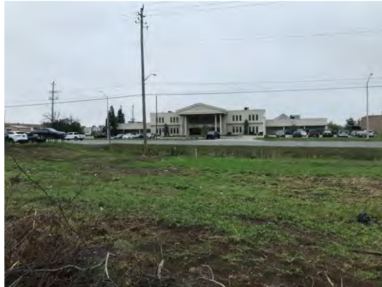
1. Upstream of Culvert 1
