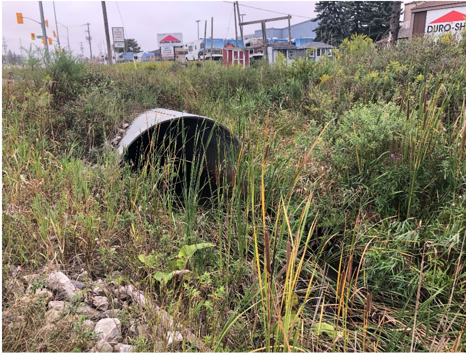
FIGURE 13 Culvert 6 Downstream End
