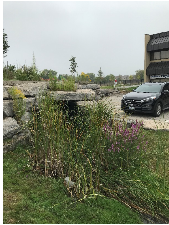
FIGURE 8 Culvert 3 Downstream End
