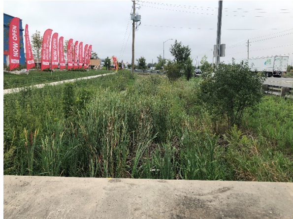
FIGURE 15 Culvert 7 Looking Downstream
