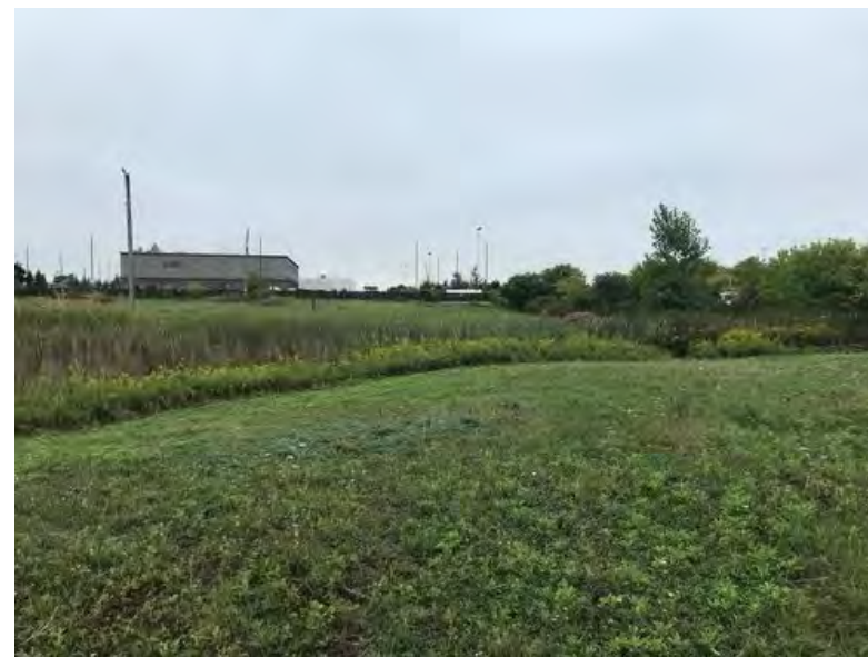
5. Upstream of Culvert 1
