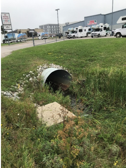
FIGURE 11 Culvert 5 Downstream End
