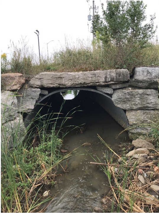
FIGURE 7 Culvert 3 Upstream End
