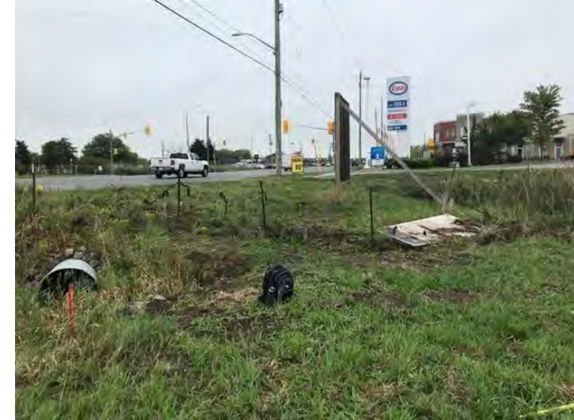
9. Culvert C1a (Inlet)
