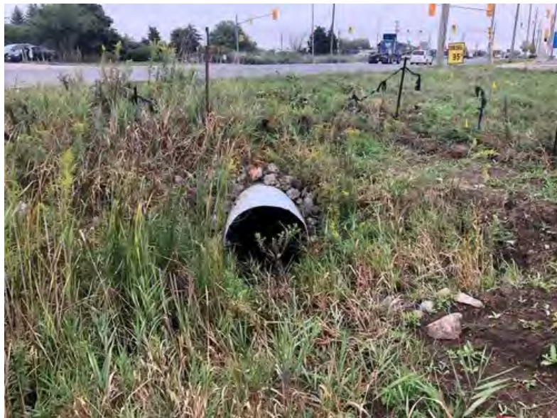
10. Culvert C1a (Inlet)
