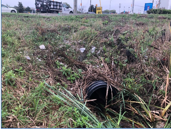
FIGURE 1 Culvert 1 Upstream End
