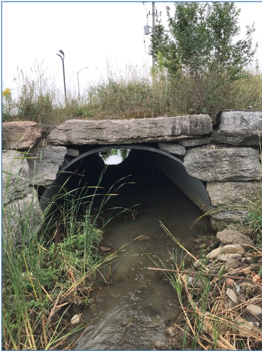
FIGURE 6 Culvert 3 Upstream End
