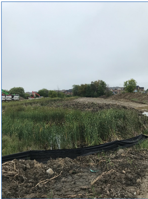
FIGURE 18 Current Channel Re-Alignment Looking Upstream
