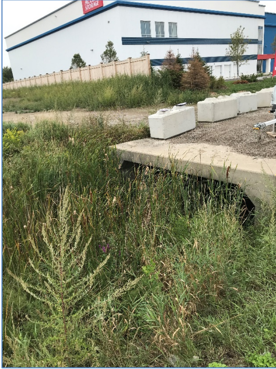
FIGURE 13 Culvert 7 Upstream End
