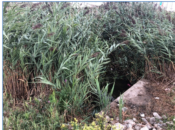
FIGURE 3 Culvert 1 Downstream End
