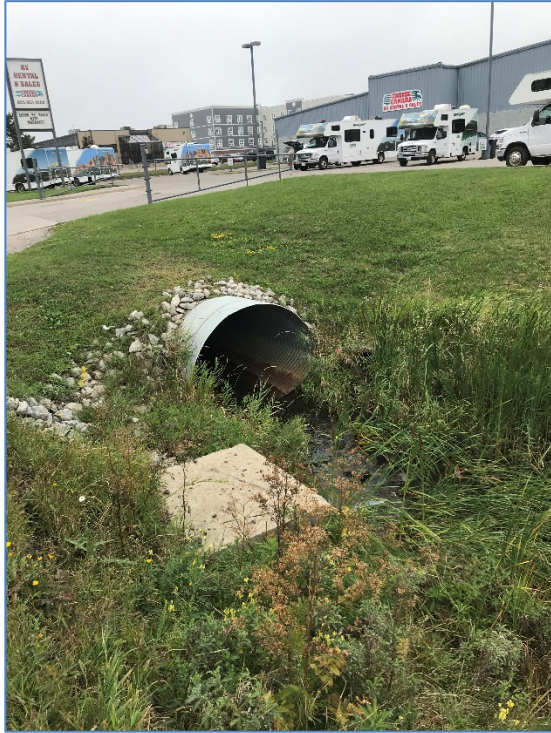
FIGURE 10 Culvert 5 Downstream End
