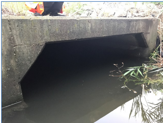
FIGURE 2 Culvert 1 Downstream End
