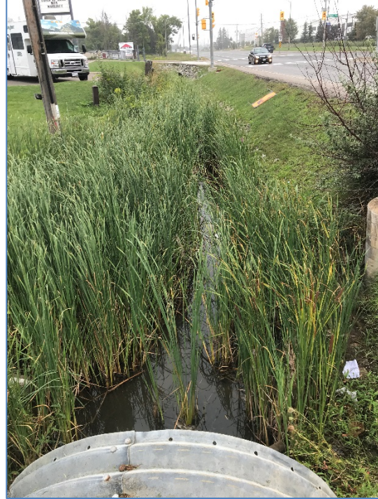
FIGURE 9 Culvert 4 Looking Downstream
