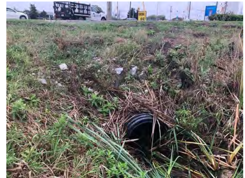
6. Culvert C1 (Inlet)
