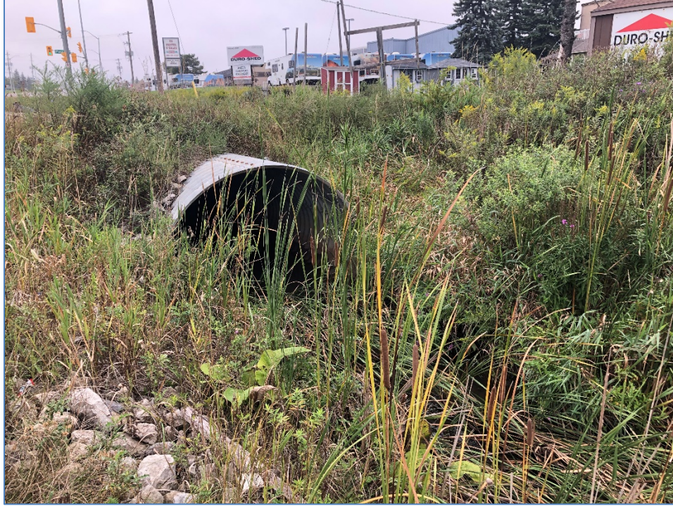
FIGURE 12 Culvert 6 Downstream End
