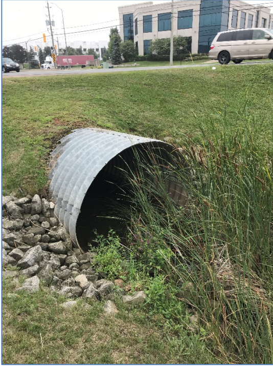
FIGURE 8 Culvert 4 Upstream End
