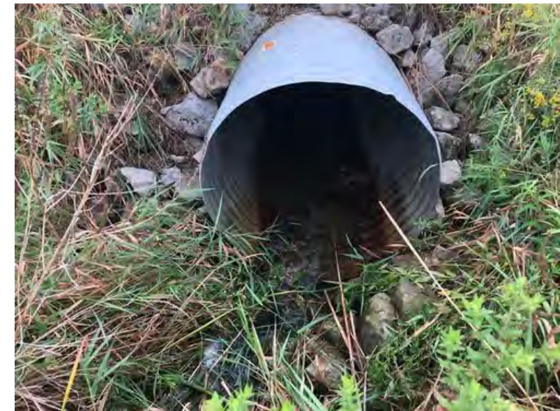
12. Culvert C1a (Inlet)
