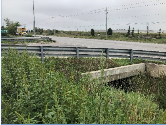
FIGURE 15 Culvert 8 Upstream End
