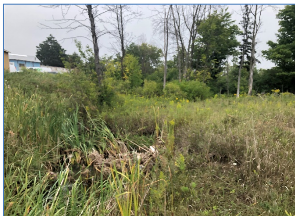
FIGURE 20 Looking Downstream from Culvert 6 (Subject Property on Right)
