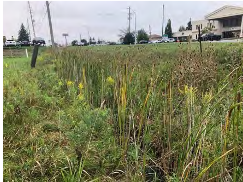
13. Culvert C1a (Inlet)
