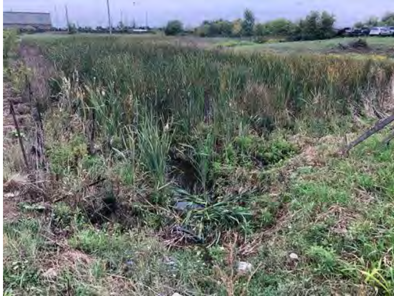
7. Culvert C1 (Inlet)
