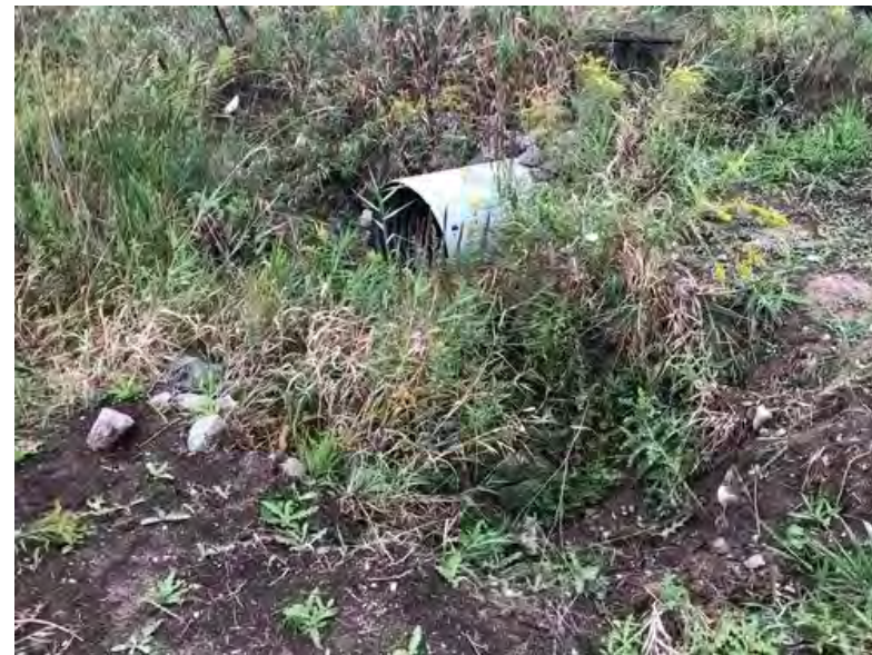
11. Culvert C1a (Inlet)
