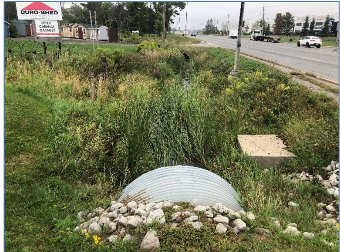
FIGURE 11 Culvert 5 Looking Downstream
