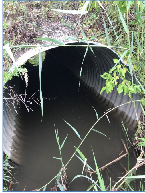
FIGURE 5 Culvert 2 Downstream End
