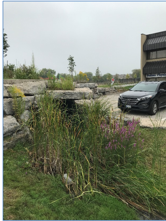
FIGURE 7 Culvert 3 Downstream End
