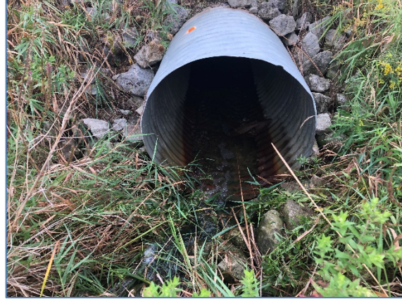
FIGURE 2 Culvert 1A Upstream End
