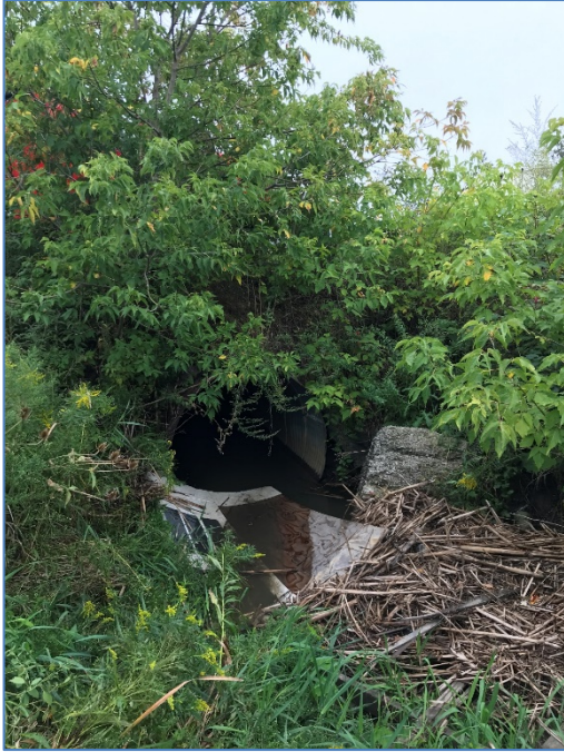
FIGURE 4 Culvert 2 Upstream End
