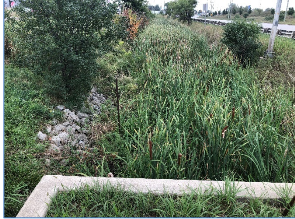
FIGURE 16 Culvert 8 Looking Downstream
