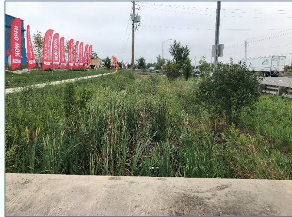
FIGURE 14 Culvert 7 Looking Downstream
