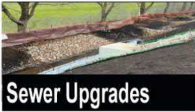
Sewer Upgrades and Replacements
