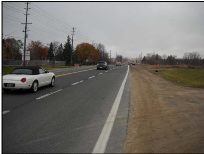
Bovaird Drive eastbound approaching Heritage Road
