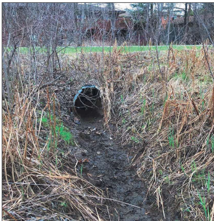
Culvert DS of C2 (DS end) 2 of 8
