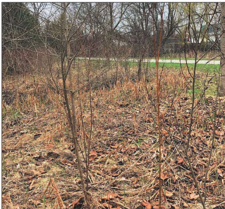
Culvert DS of C2 (DS end) 6 of 8
