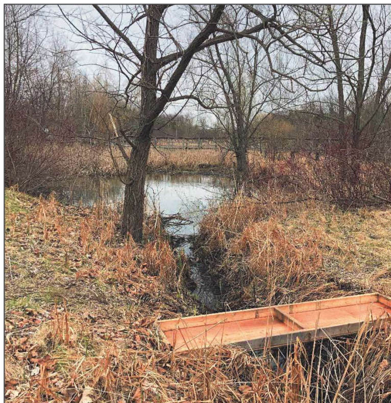
Culvert DS of C2 (DS end) 8 of 8
