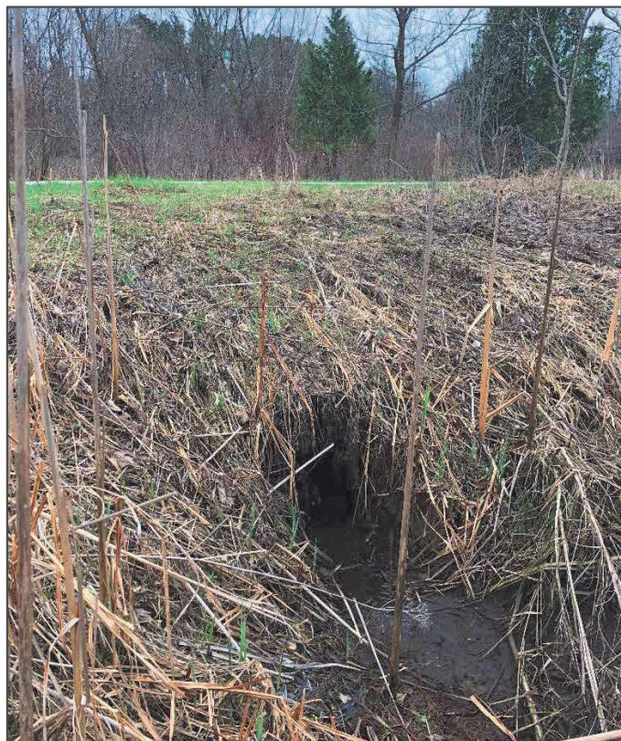
Culvert DS of C2 (US end) 2 of 2
