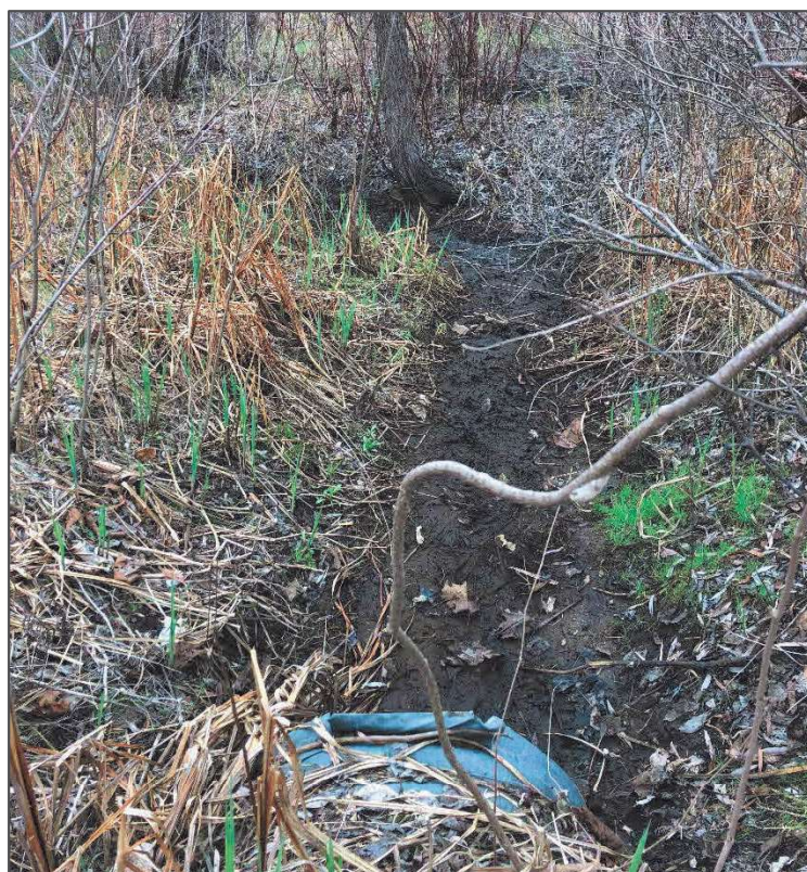
Culvert DS of C2 (DS end) 7 of 8
