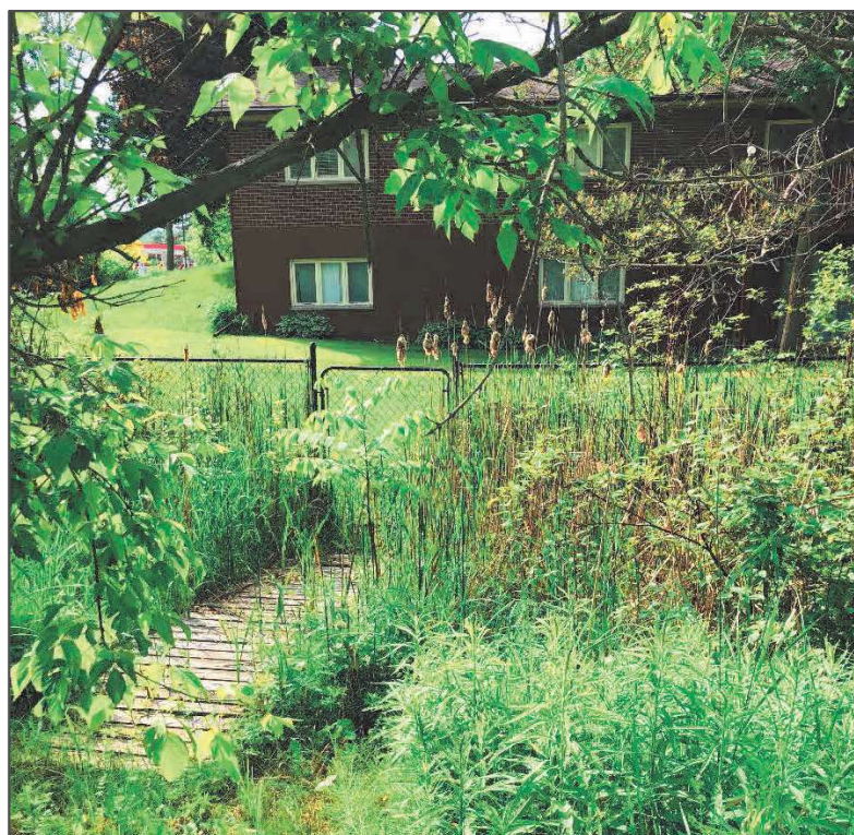
Culvert DS of C2 (US end) 1 of 2
