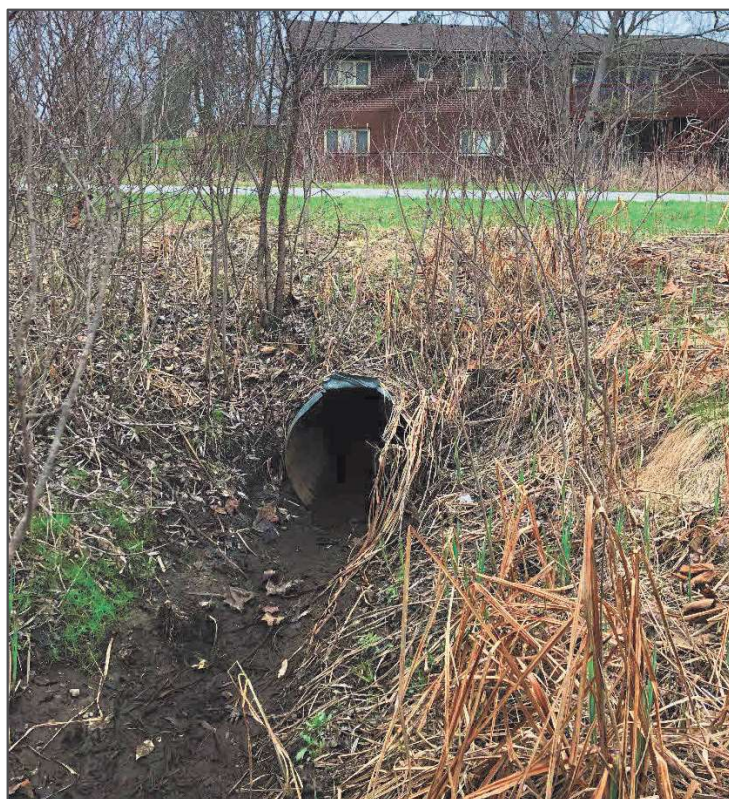
Culvert DS of C2 (DS end) 3 of 8
