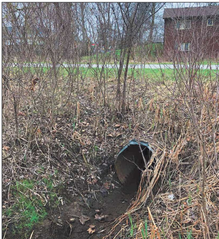
Culvert DS of C2 (DS end) 4 of 8
