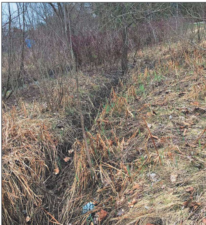
Culvert DS of C2 (DS end) 5 of 8
