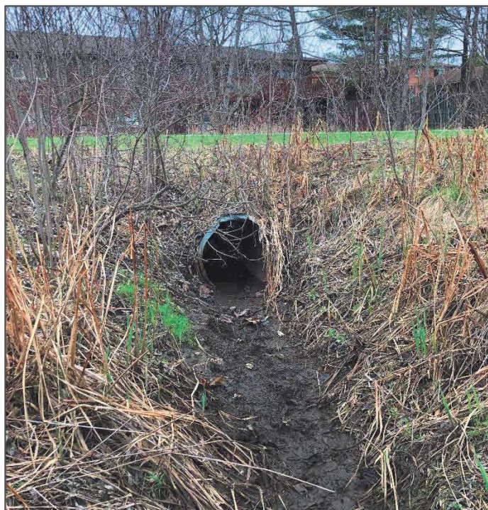
Culvert DS of C2 (DS end) 1 of 8
