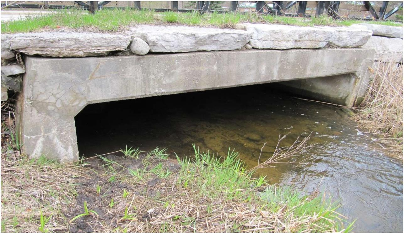
Pic 013 – Culvert Inlet (West Side) – Note Shrinkage Cracks at the Exterior Surfaces (End)
