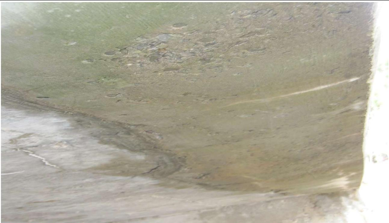
Pic 016 – Scaling at The Interior Surfaces (Soffit) – East End
