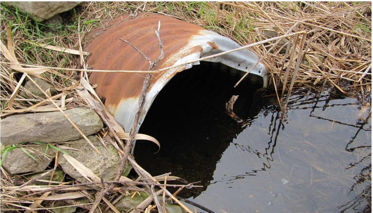
Pic 006 – Culvert Outlet (East Side) – Note Damaged CSP
