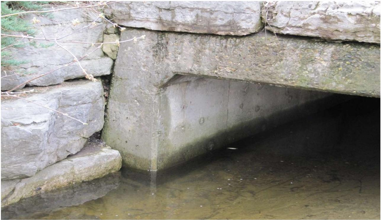
Pic 015 – Concrete Scaling at the Culvert Outlet – Exterior Surfaces (End)
