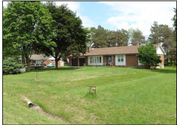
Plate 2: Example of mid- to late-twentieth century housing stock found along the study corridor.
