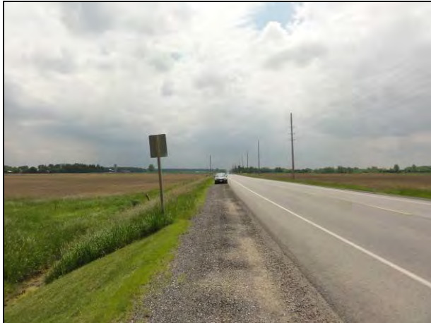
Plate 1: View west along Mayfield Road between Chinguacousy Road and McLaughlin Road.
