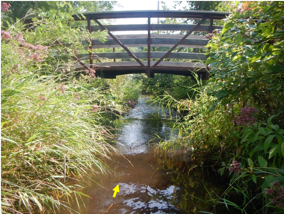
The creek passes beneath the Caledon Trailway before crossing Airport Road. An artificial riffle composed of gravel and cobble was present downstream of the bridge.
