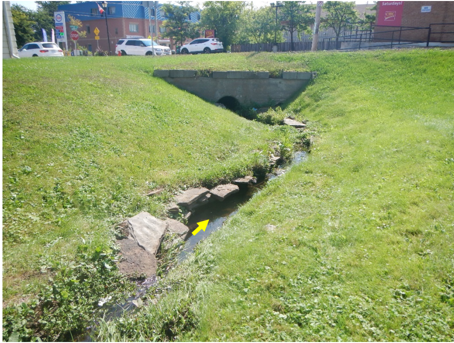
The watercourse was bounded by manicured grass. One bank was largely armoured with flagstone.
