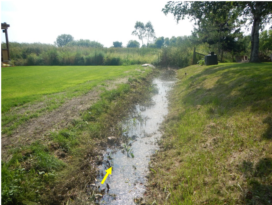
Riparian vegetation consisted of manicured lawns within the residential properties. At the edge of the property material has accumulated against the fence, which spans the channel, and is creating a backwater which extended to Crossing 7.
