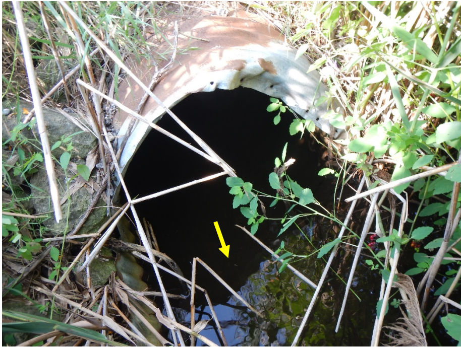
The downstream end of Crossing 1 on the east side of Airport Road was free of debris.
