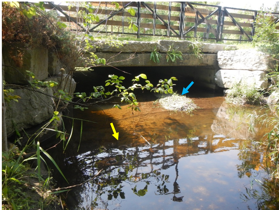
A sandy lag deposit (blue arrow) was present downstream of the debris jam within Crossing 3. Downstream of the crossing was a shallow pool with bed material composed of sand and silt.
