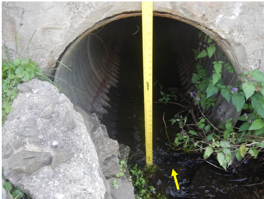
Crossing 2 is a 0.8 m diameter CSP culvert.
