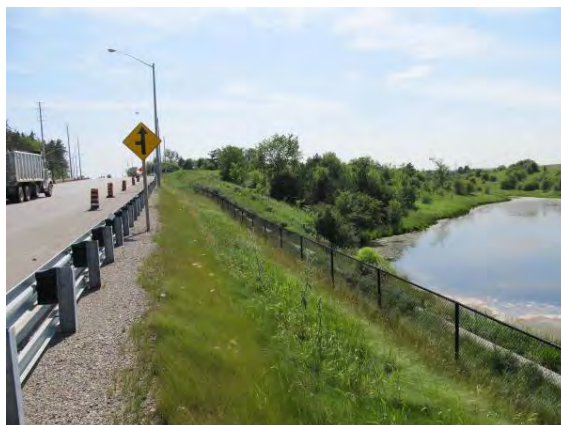
Plate 28: Southwest view along Mayfield Road. Storm water management pond, slope, and disturbed ROW. No potential.
