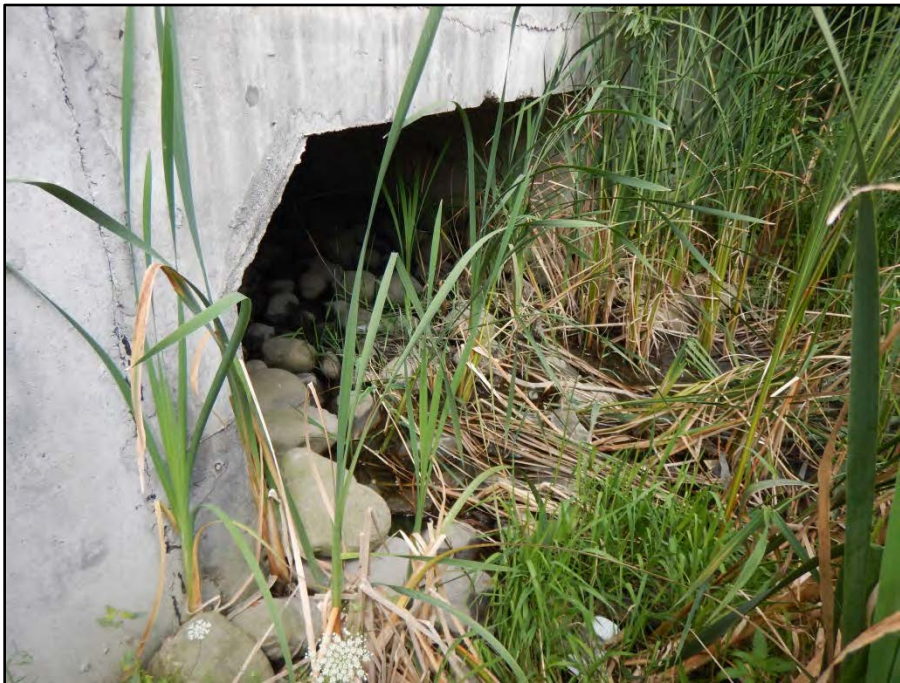
10. Downstream culvert outlet with boulder rip rap and cat tail vegetation.
