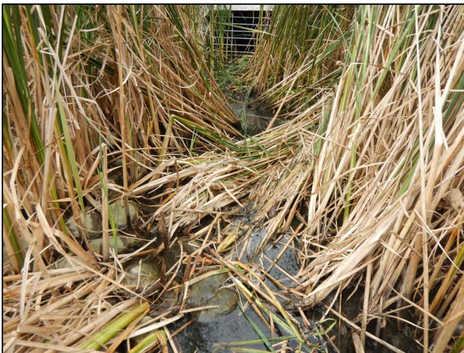
12. Looking upstream to the Airport Road culvert outlet. Cat tail grown increases bed roughness resistance and slows the velocity of downstream flow.
