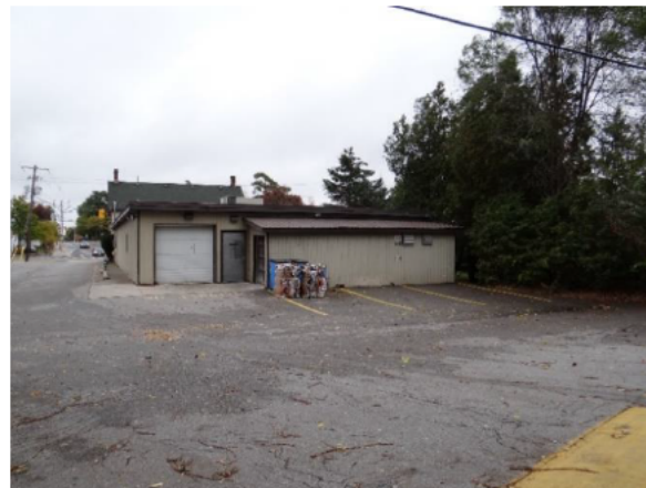
Figure 18: West elevation of the 1985 addition and the rear of the property with garage entrance and extension.
