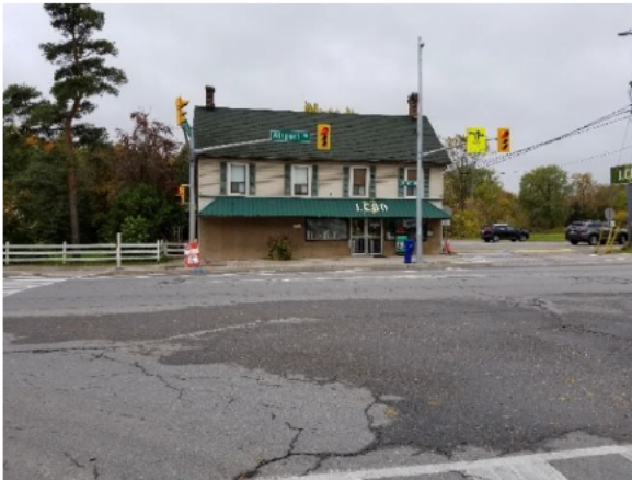
Figure 11: East elevation of the structure at 16000 Airport Road.
