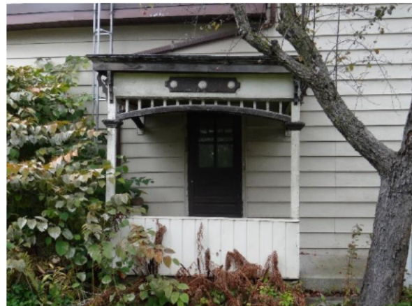
Figure 14: Detail of the original covered southern entrance.
