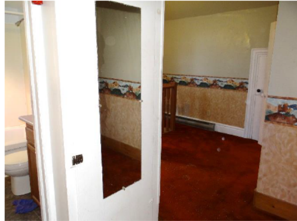
Figure 24: View to landing area at the top of the staircase with the bathroom at left and crawlspace door at right.
