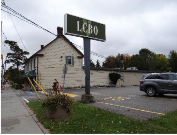
Figure 33: Parking lot to the north of the building, looking southwest.
