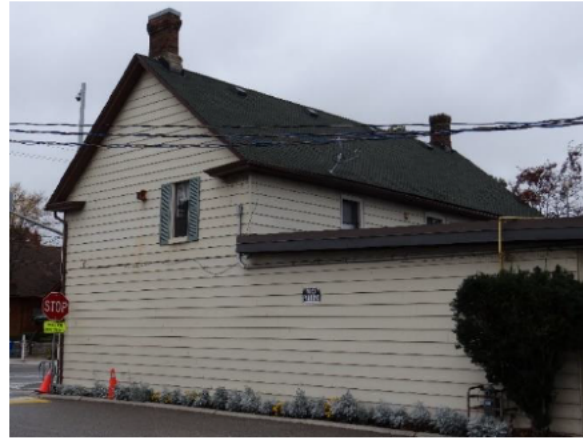
Figure 16: North elevation and west elevation of the original portion of the building, looking southeast.
