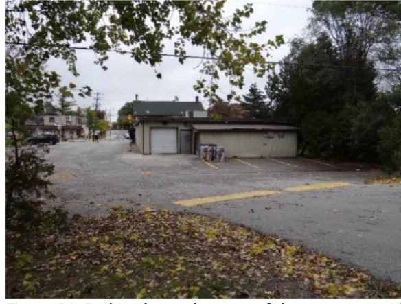
Figure 34: Parking lot at the west of the structure with access from Ivan Avenue, looking east.
