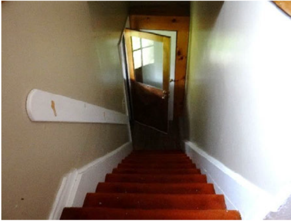
Figure 23: Staircase to upper floor, looking down to the exit.
