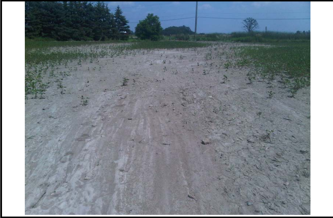
PHOTOGRAPH NO.: 19 FROM: LOOKING: Upstream COMMENT: Reach L
