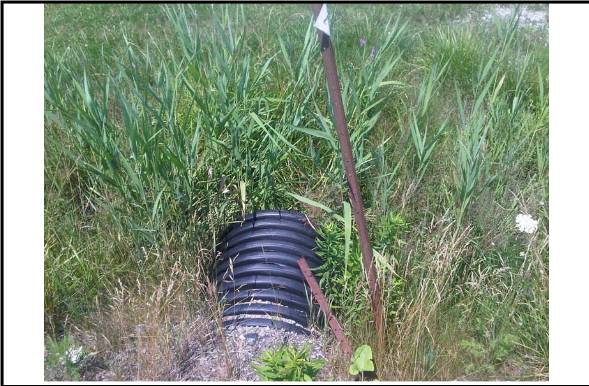
PHOTOGRAPH NO.: 9 FROM: LOOKING: Upstream COMMENT: Reach G
