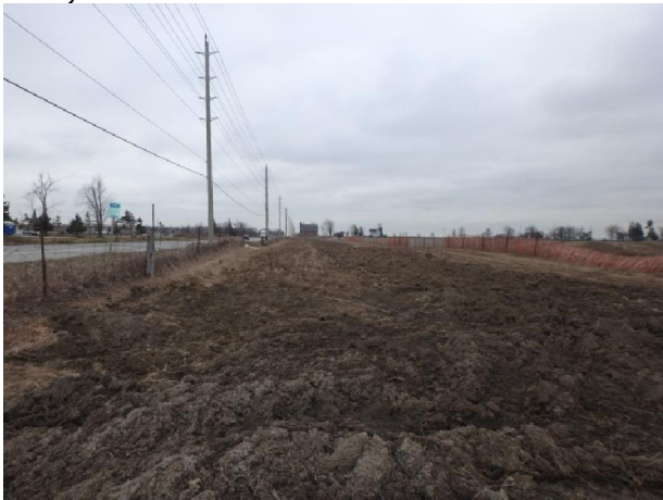
Plate 27: View SW of study corridor. Lands assessed by test-pit survey complimented by pedestrian survey
