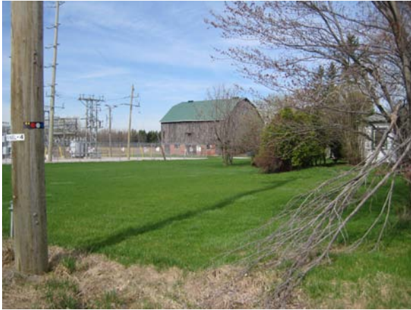
Plate 33: View west from Mayfield Road. Transformer station disturbed. Lawn has potential. Requires Stage 2 test-pit survey.
