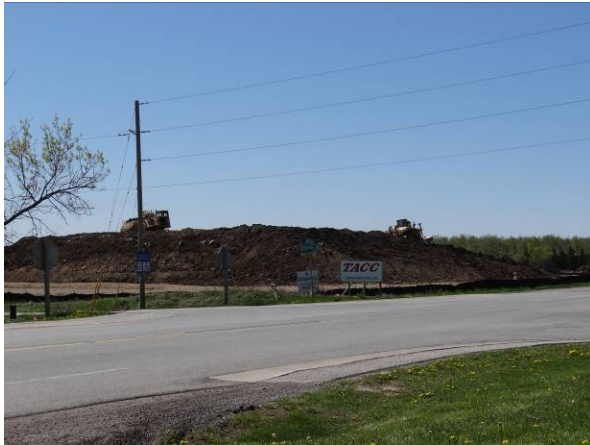
Plate 7: South view across Mayfield Road towards construction. Property is under development.
