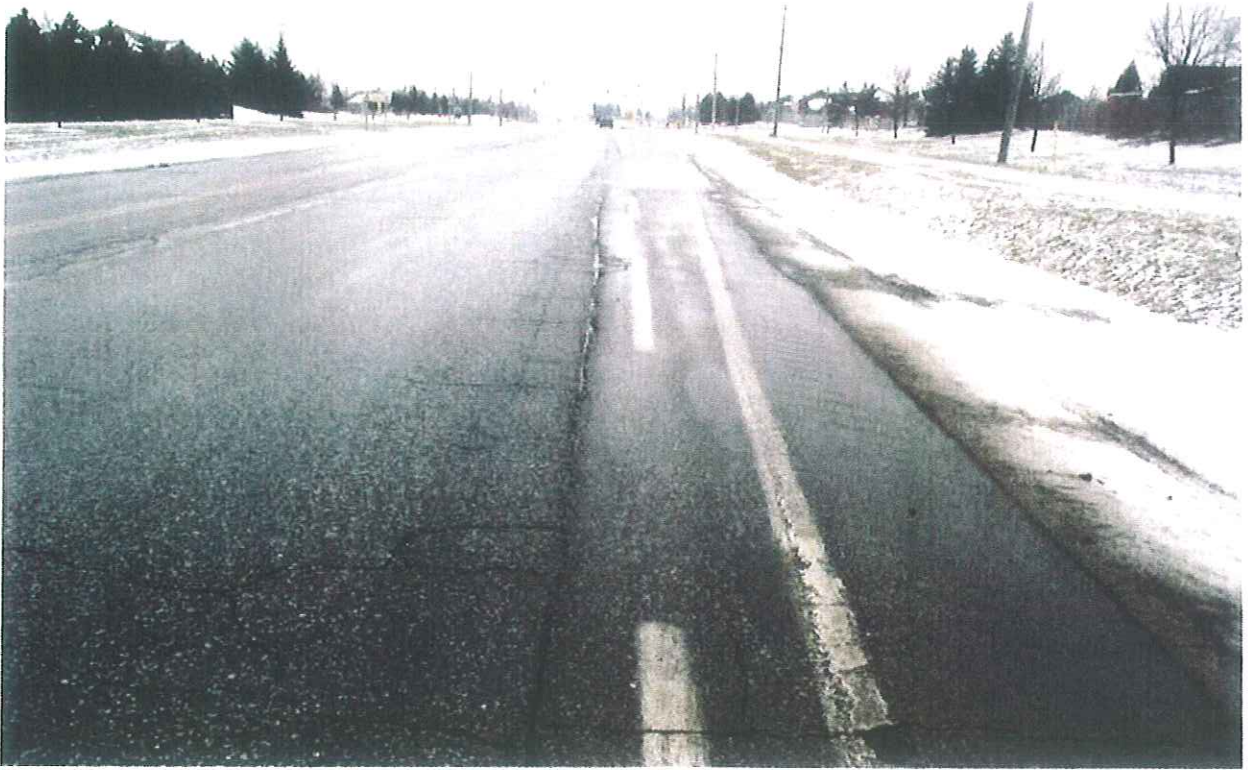
Mayfield Road\Section 4\Looking towards West
