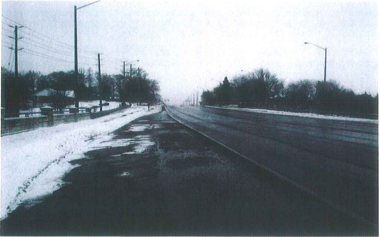
Mayfield Road\ Looking towards West\Structural Bridge crossing a Tributary\700 m West of Kennedy Road
