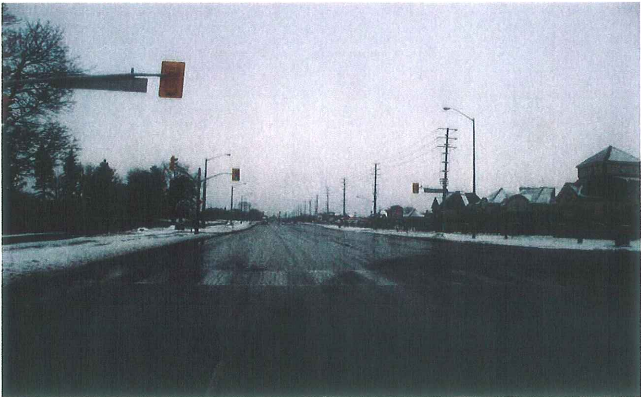
Mayfield Road\ Section 3\Looking towards West\1100m west of Kennedy Road
