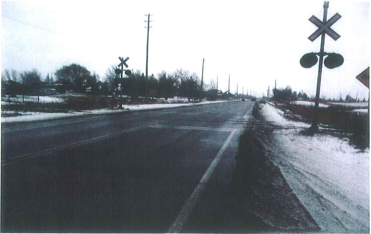
Mayfield Road\Section 4\Looking towards West\Railway Crossing
