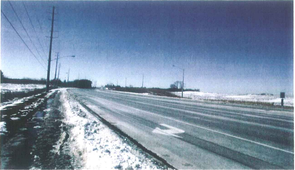
Mayfield Road\Section1\ Looking Towards West
