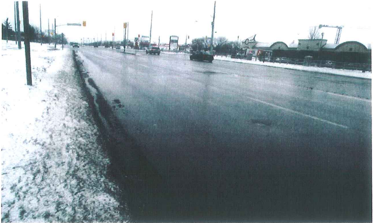
Mayfield Rd\Section 3\Looking towards West, 250 m East of Hurontario Street
