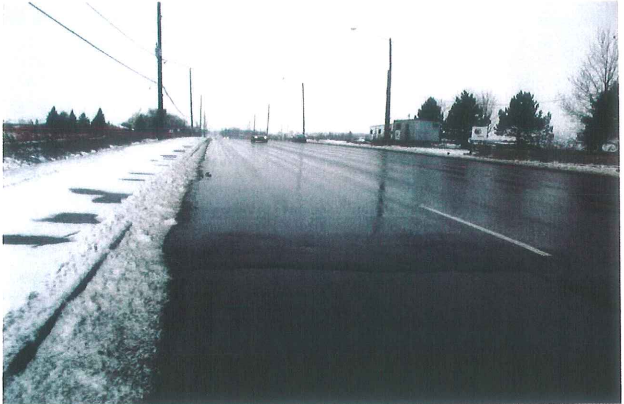
Mayfield Road\Section3\Looking towards West
