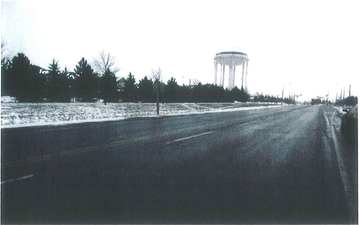
Mayfield Road\Section 4\Looking towards West, 400 m West of Hurontario Street
