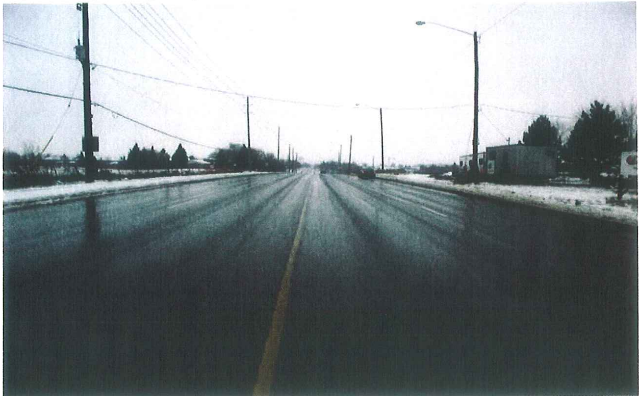
Mayfield Road\Section3\Looking towards West, 200 m East of Kennedy Rd.
