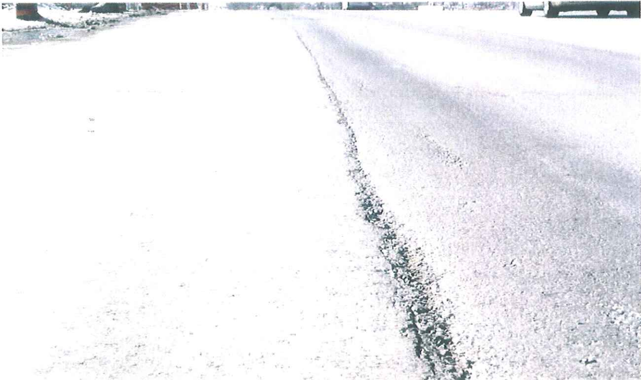
Mayfield Road\Section2\ Looking towards West\East Bound of Mayfield Rd.
