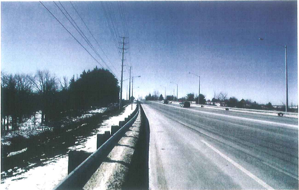
Mayfield Road\Section1\ Looking towards West\South side of Mayfield Rd., High Fill Embankment
