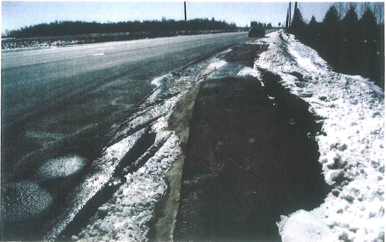
Mayfield Road\Section 5\Looking towards West
