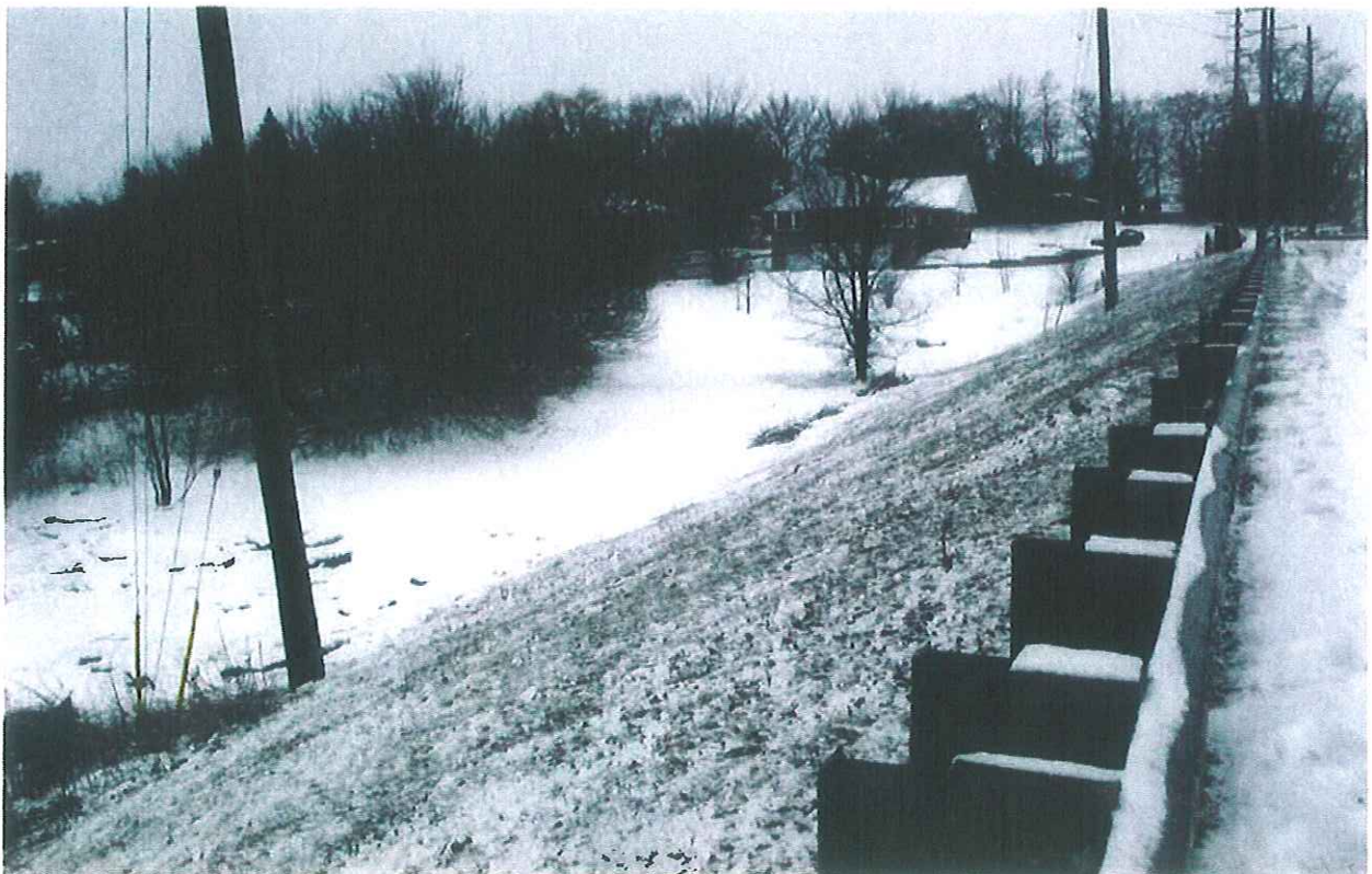
Mayfield Road\ Section 3\Looking towards West\Embankment Fill west of the Structural Bridge \ South side of Mayfield, West of the Bridge
