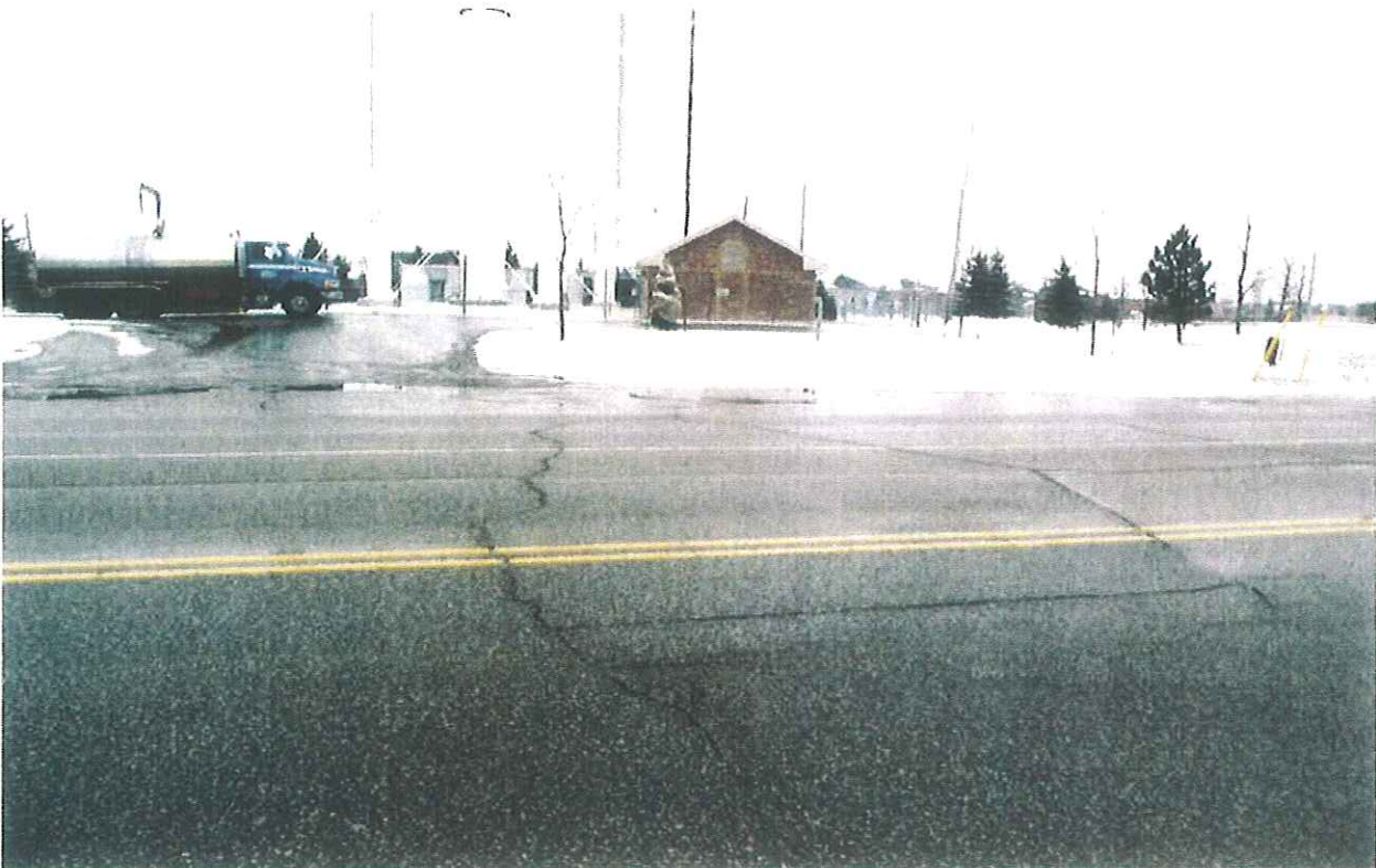
Mayfield Road\Section 4\Looking towards South
