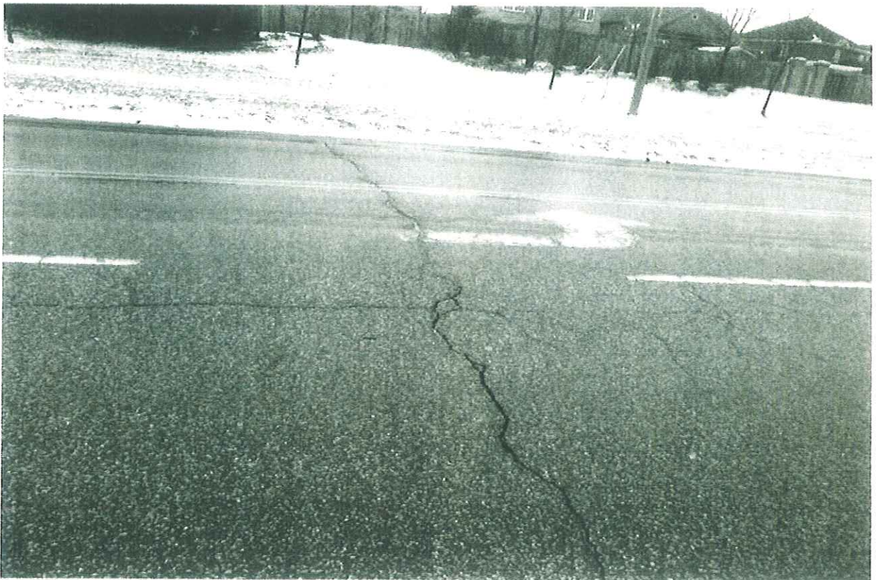
Mayfield Road\Section 4\Looking towards South
