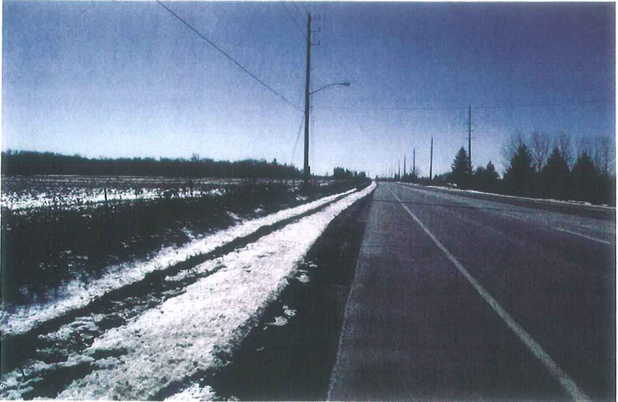
Mayfield Road\Section 5\Looking towards West
