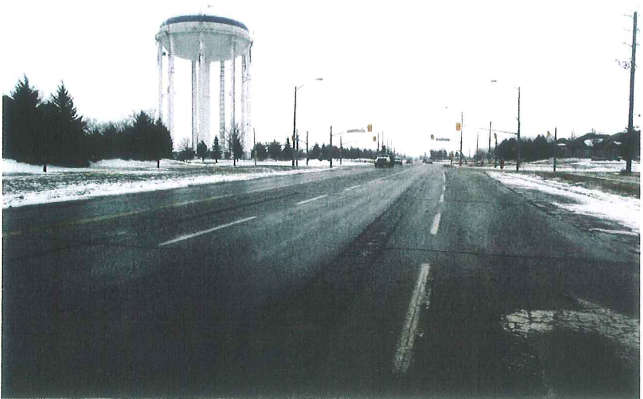
Mayfield Road\Section 4\Looking towards West
