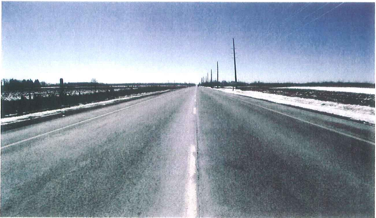
Mayfield Road\Section 5\Looking towards West
