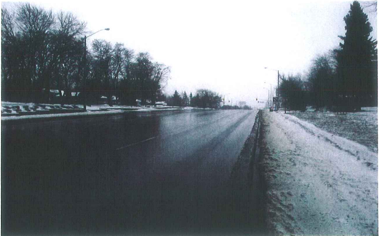
Mayfield Road\Section 3\ Looking towards West\900m west of Kennedy Road
