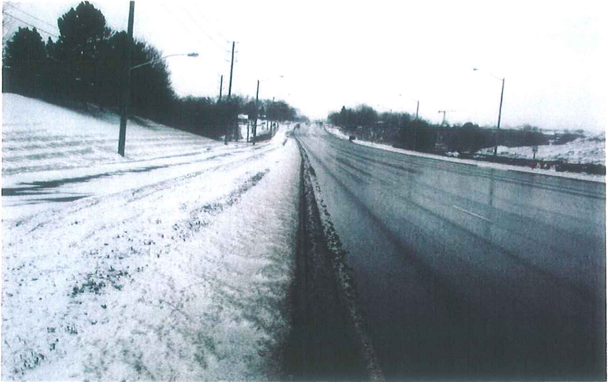
Mayfield Road\Section3\Looking towards West
