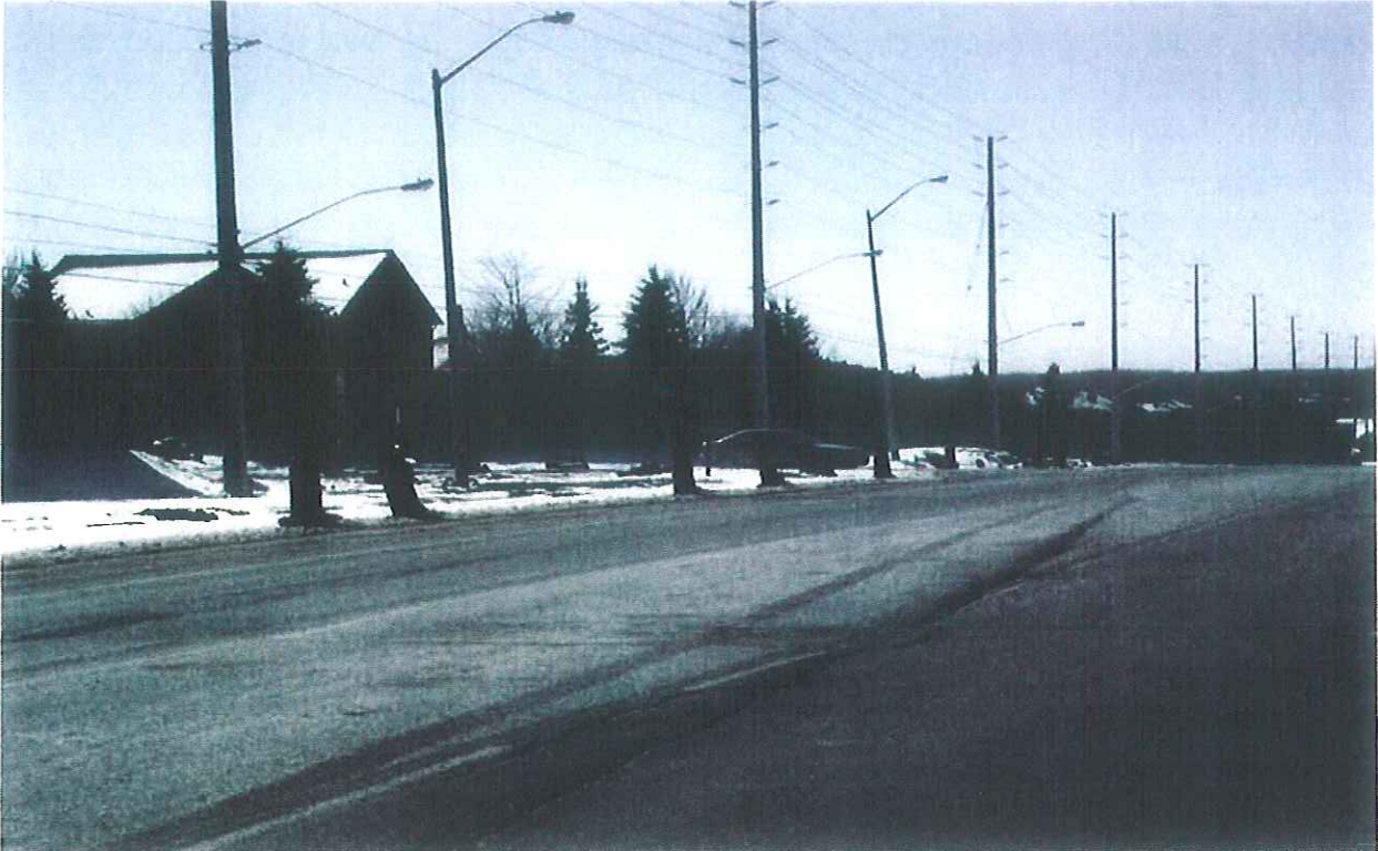
Mayfield Road\Section2\ Looking towards West\cracks and Distortion Area \See Noise Wall along the South Side of Mayfield Road
