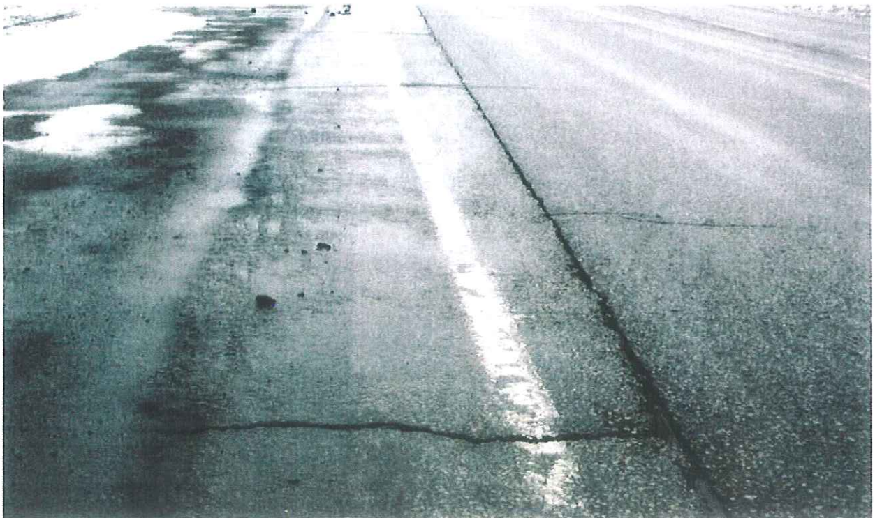
Mayfield Road\Section 4\Looking towards West, 500 m West of Hurontario Street
