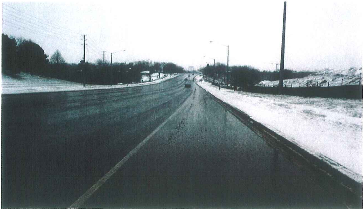
Mayfield Road\Section3\Looking towards West, 500 m West of Kennedy Rd.
