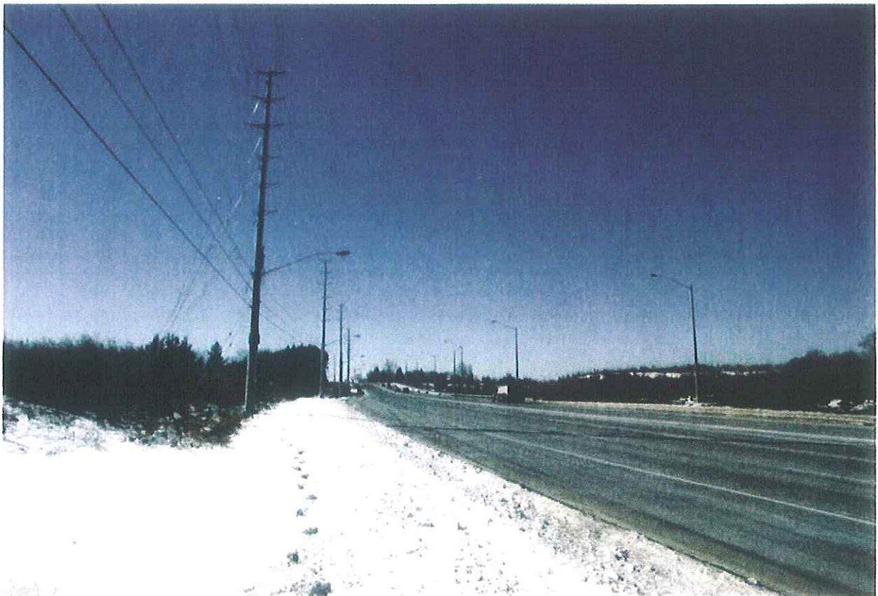
Mayfield Road\Section1\ Looking Towards West
