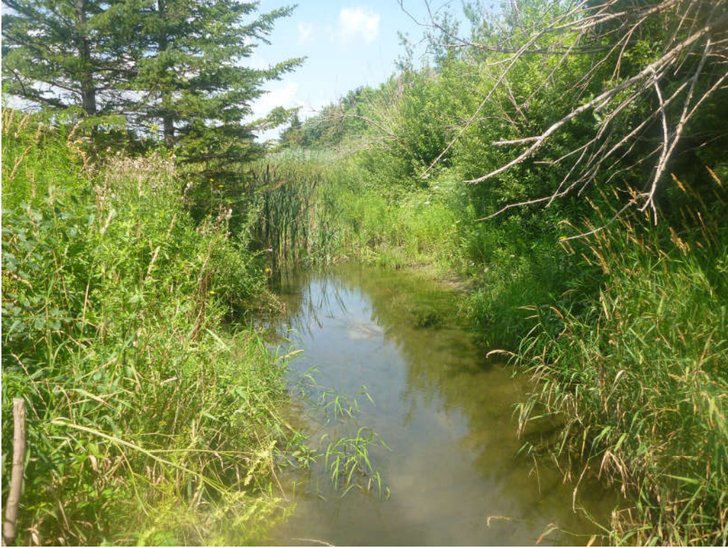
Photo 7 – Facing upstream towards culvert, parallel to Airport Road
