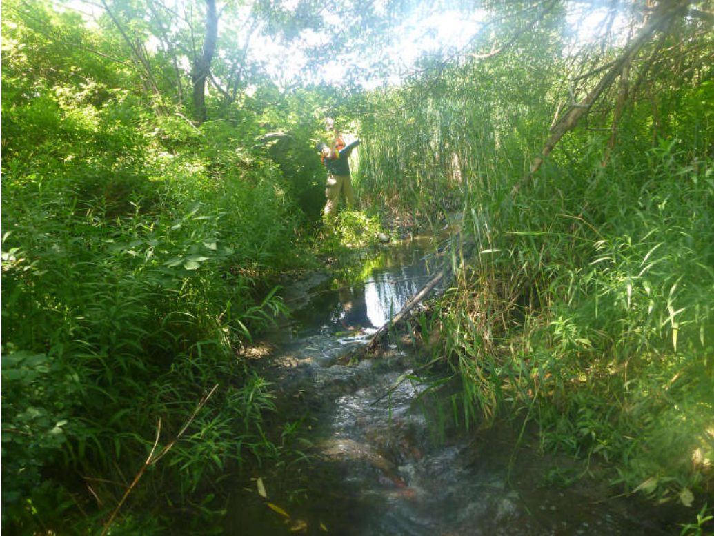
Photo 17 – Facing towards Airport Road downstream of the culvert (flowing channel)
