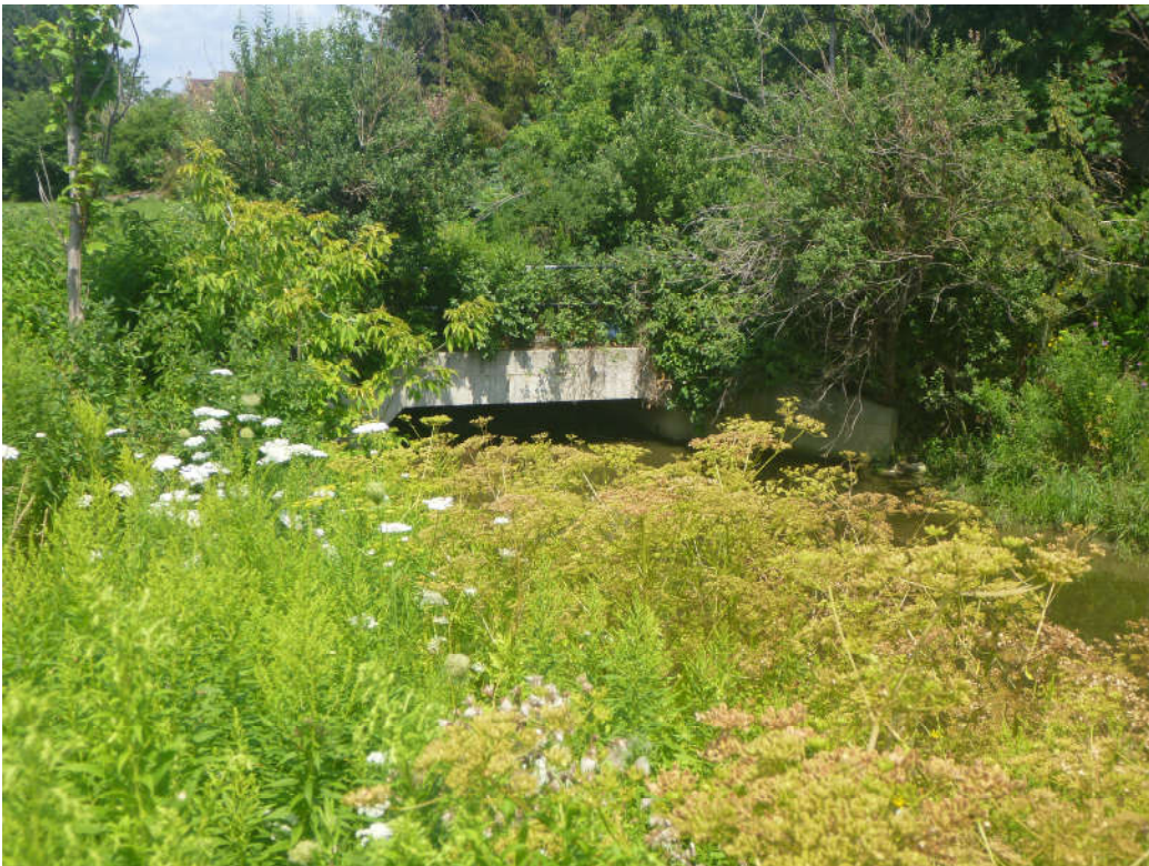
Photo 6 – Culvert and Pool feature facing upstream towards Airport Road
