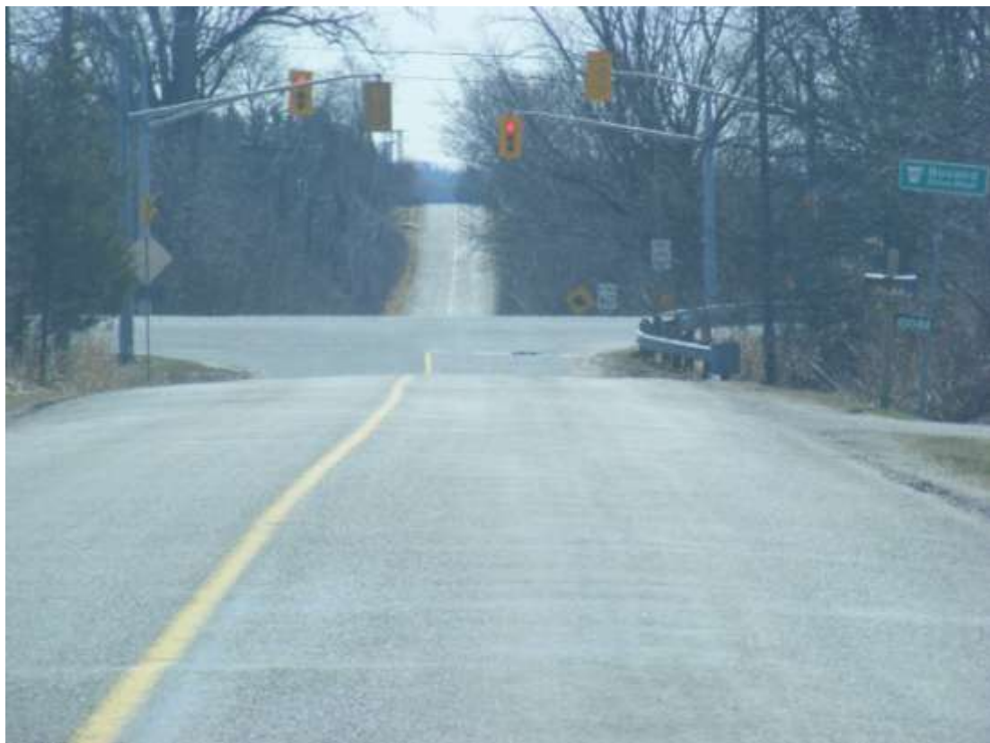
FIGURE 4.2: Signal Head Obstructed by Mast Arm at Heritage Road
