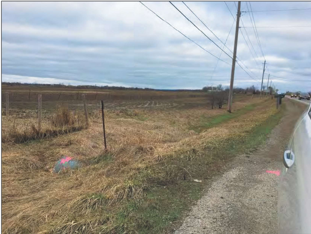
Crossing 6: HUM6-A (roadside ditch on the west side of Airport Road), looking north
