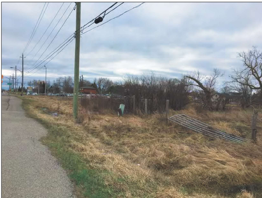
Crossing 6: HUM6-A (roadside ditch on the west side of Airport Road), looking south
