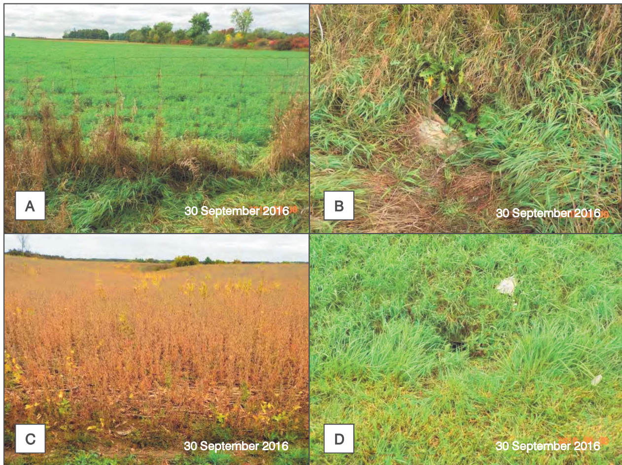
Figure 22. Crossing 4: (A) Looking west of the crossing structure; (B) Looking at the crossing structure west end; (C) View east from the crossing structure; (D) Crossing structure east end.
