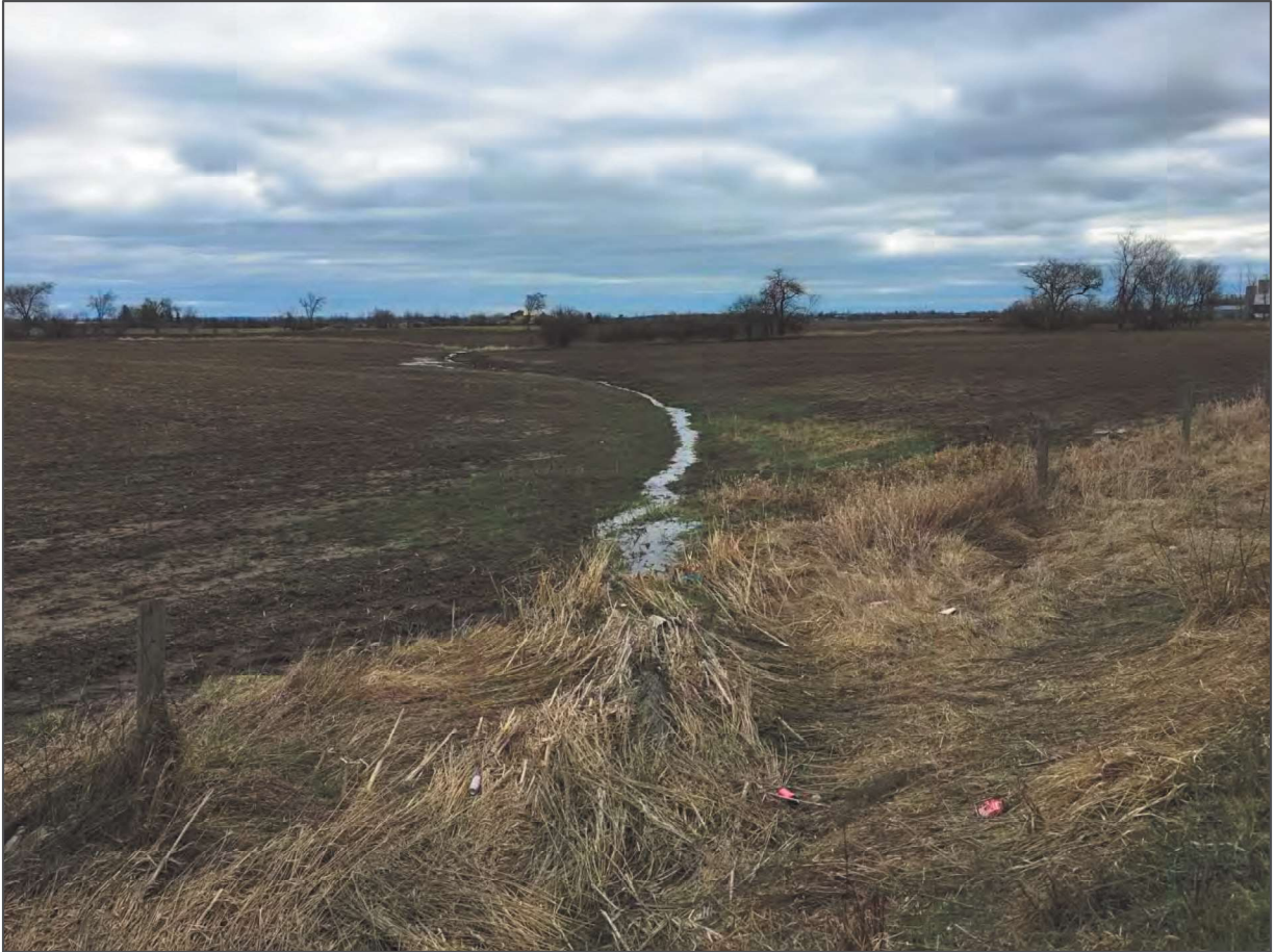
Crossing 5: HUM5-C, or view south-east of the crossing structure
