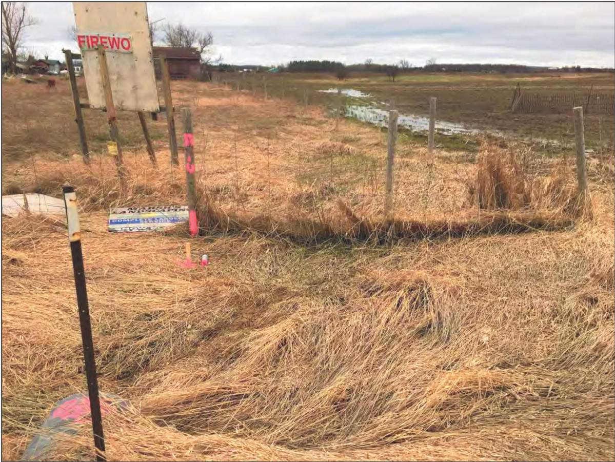
Crossing 6: HUM6-B (undefined feature on the west side of Airport Road), or looking west from the crossing structure
