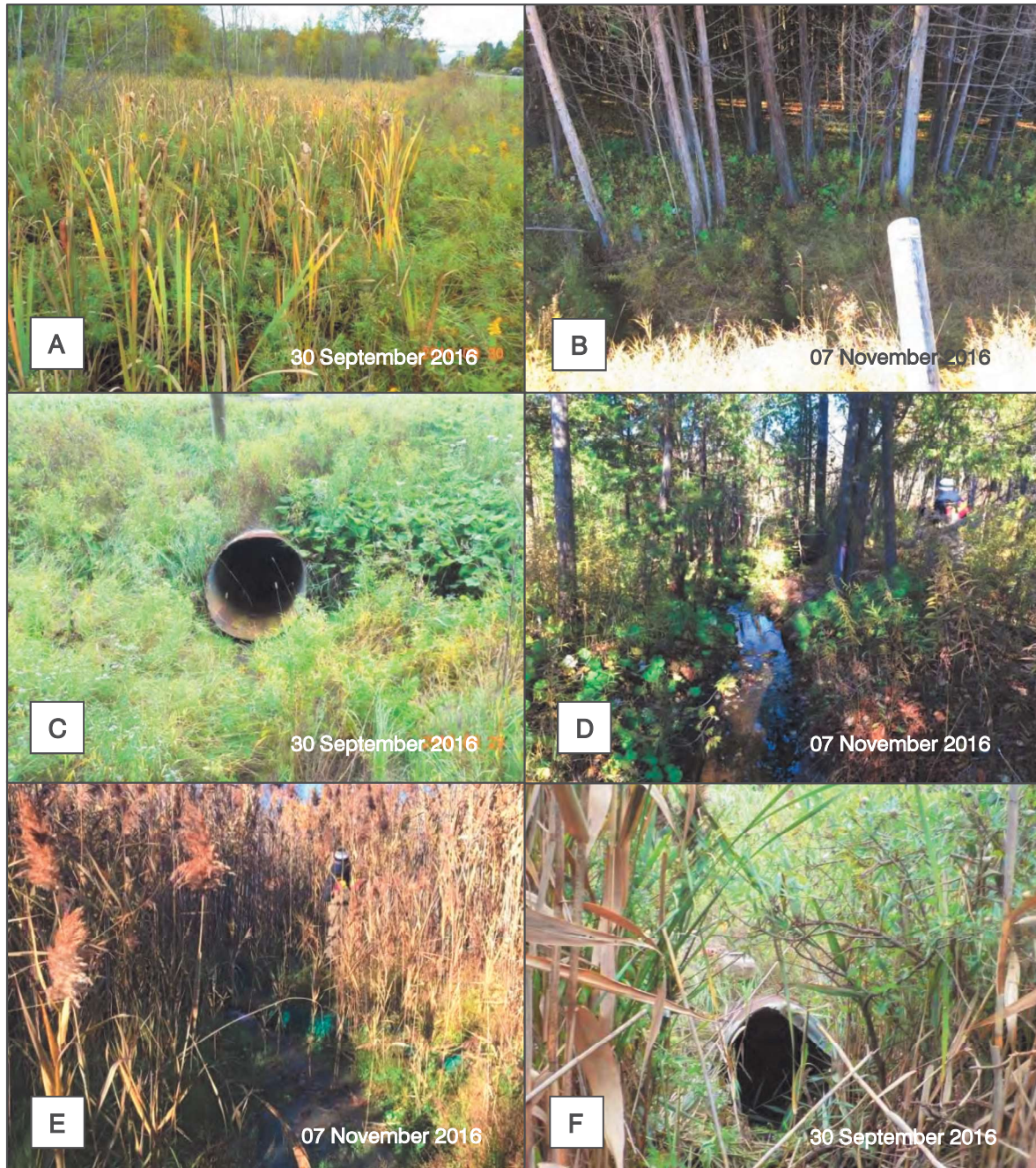
Figure 19. Crossing 1: (A) Wetland area west of Airport Road; (B) View west from where culvert passes under Airport Road; (C) View of the culvert structure from the west side; (D) Forested area east of Airport Road; (E) View of channel from culvert opening on the east side of Airport Road; (F) View of the culvert opening on the west side of Airport Road.
