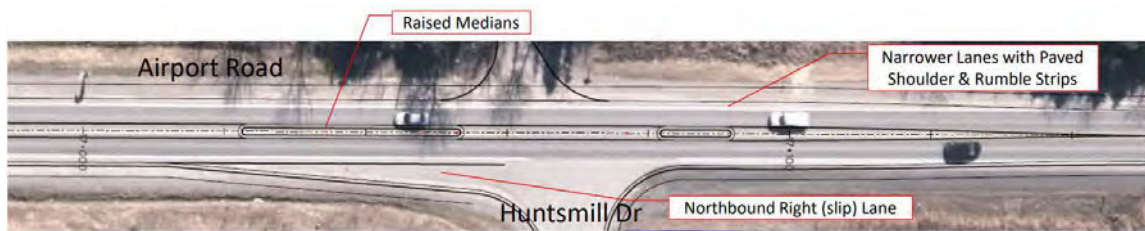
Figure 9: Airport Road and Huntsmill Drive
