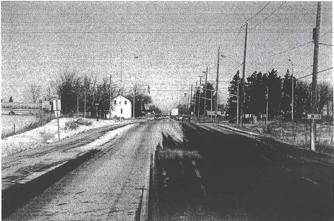
Figure 3: Mayfield Road Looking West To Dixie Road at Mayfield
