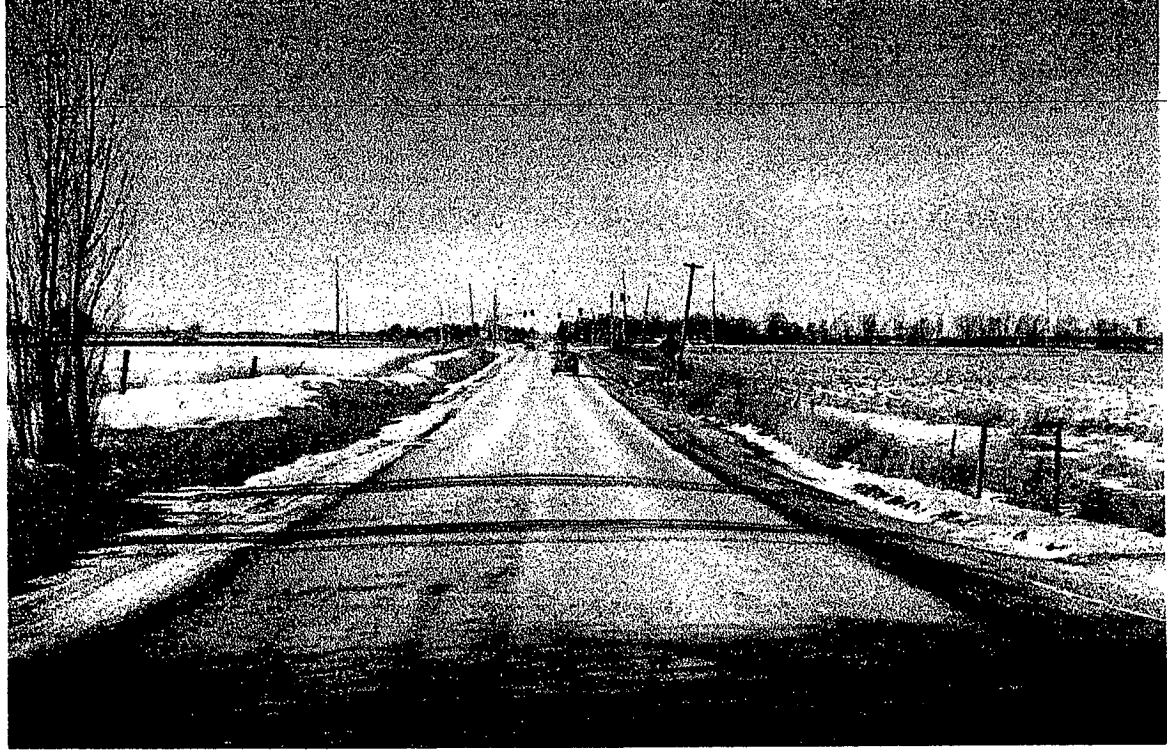
Photograph 20: Looking north along Torbram Road toward the Mayfield Road intersection.
