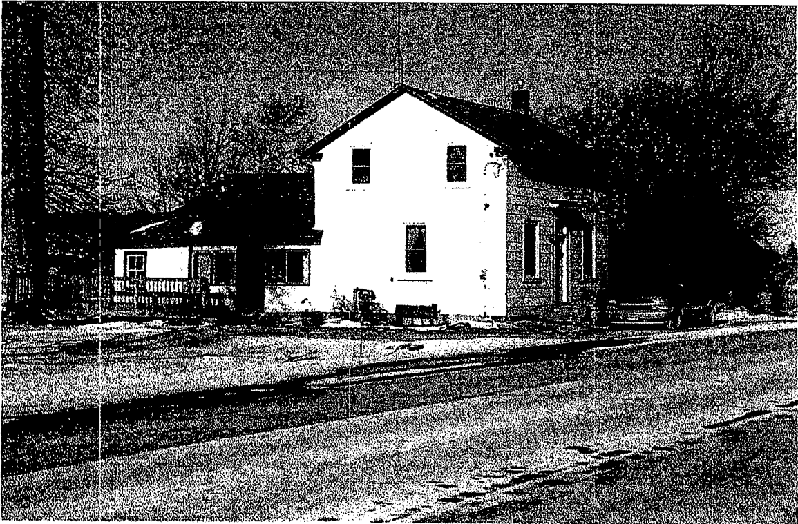
Photograph 10: Looking east at 4524 Mayfield Road. White asbestos shingled house with green roof.
