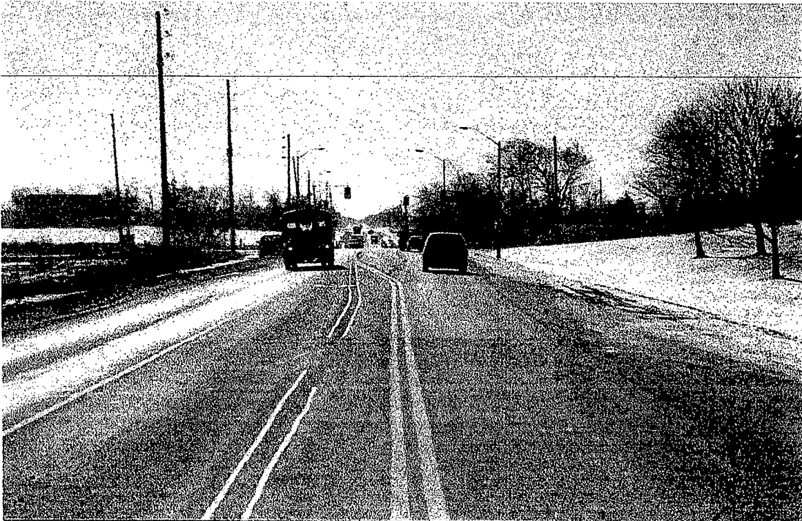
Photograph 16: Looking west along Mayfield Road toward the Bramalea Road intersection.
