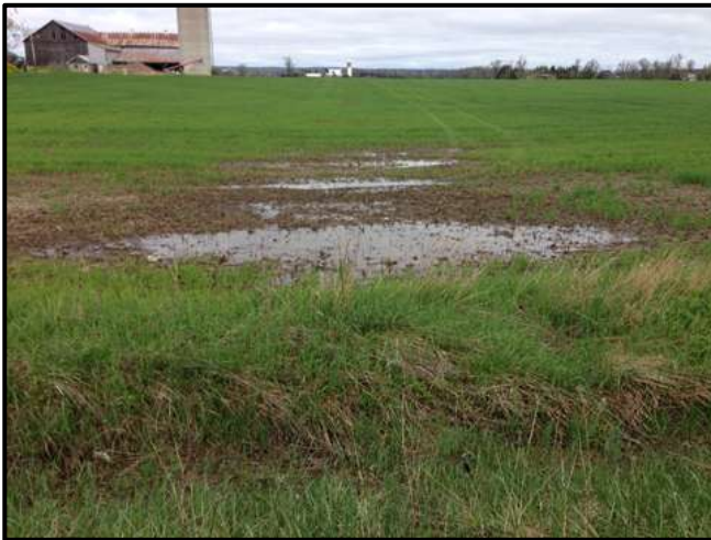
Photo 23. North of Mayfield Road. No culvert connection.
