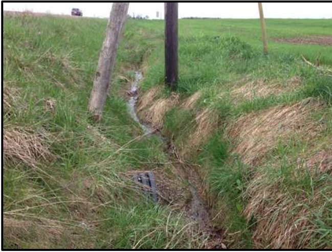
Photo 25. Upstream of Mayfield Road. Flows from ditch.
