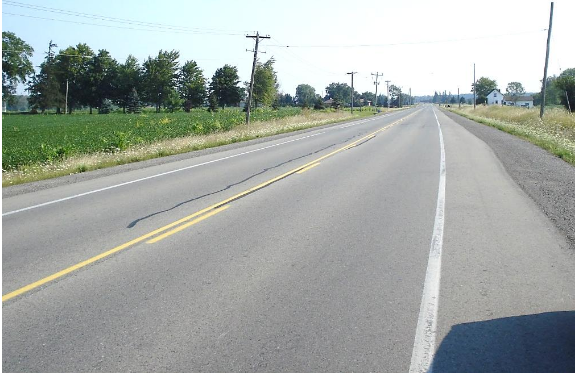
Typical Photograph #3 Mayfield Road – Station 1+260 (Looking Easterly)
