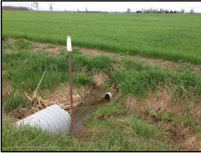
Photo 21. Upstream of Mayfield Road. Note tile drain outlet.
