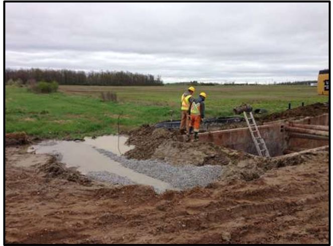
Photo 6. Downstream of Mayfield Road. Note active construction and flow diversion.
