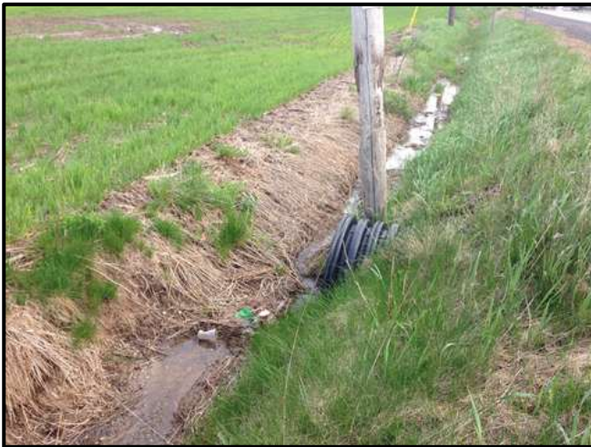
Photo 27. Upstream of Mayfield Road. Flows from ditch.
