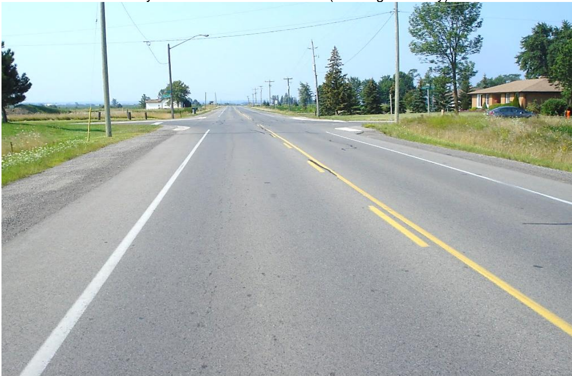
Typical Photograph #4 Mayfield Road – Station 1+845 (Looking Westerly)
