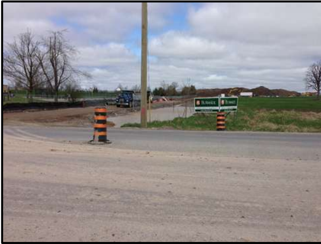
Photo 13. North of Mayfield Road. No feature and no culvert connection.
