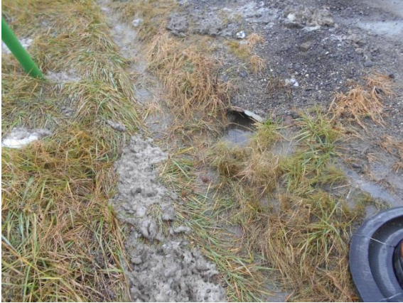
#3 – Mayfield Road looking North at Culvert Inlet
