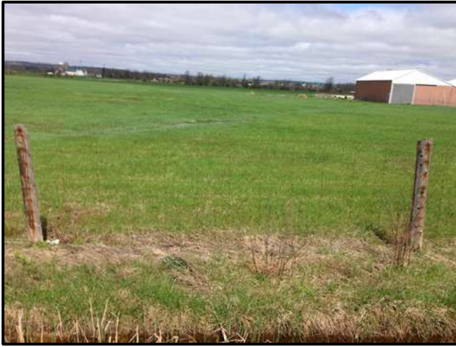
Photo 29. North of Mayfield Road. No culvert connection.
