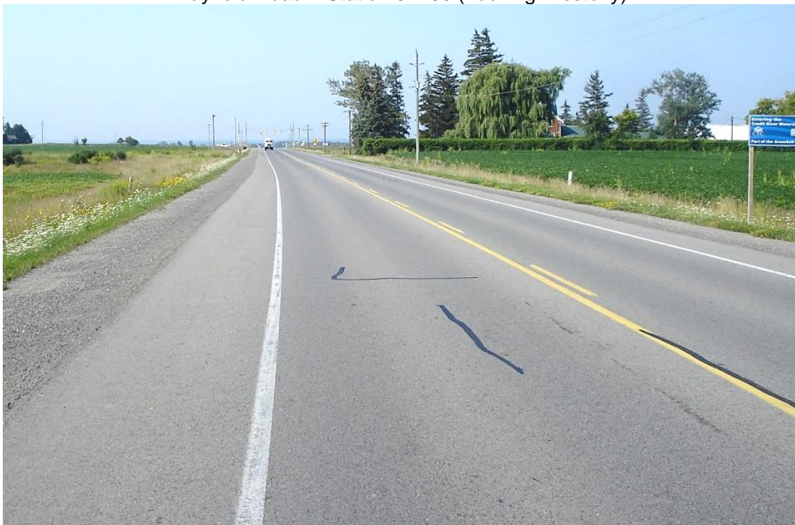
Typical Photograph #2 Mayfield Road – Station 0+760 (Looking Westerly)
