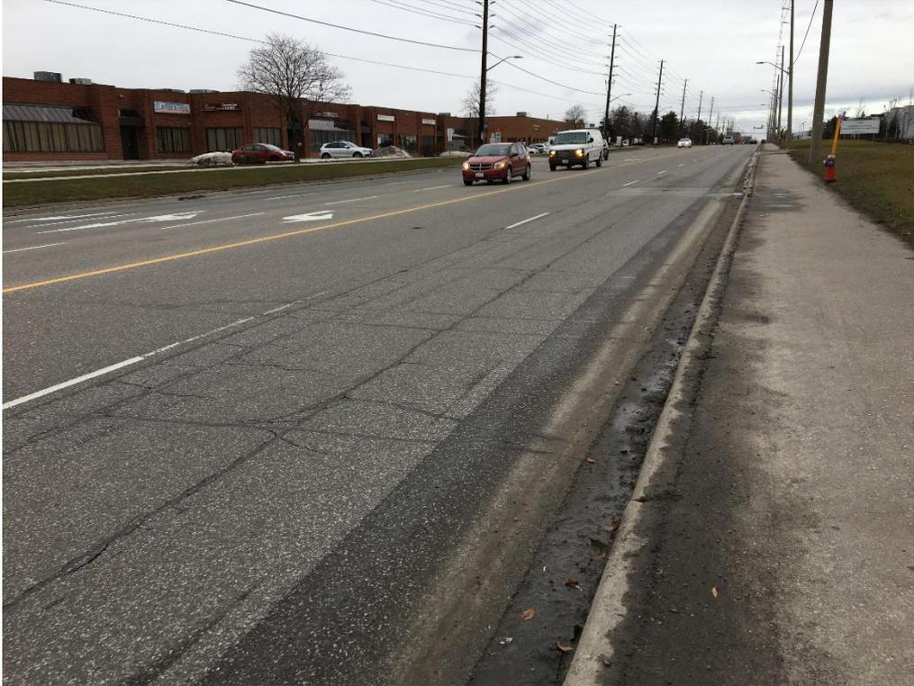
**Photo 1: Longitudinal and Transverse Cracking (Slight to Moderate Severity)-Bramalea Road WB**
