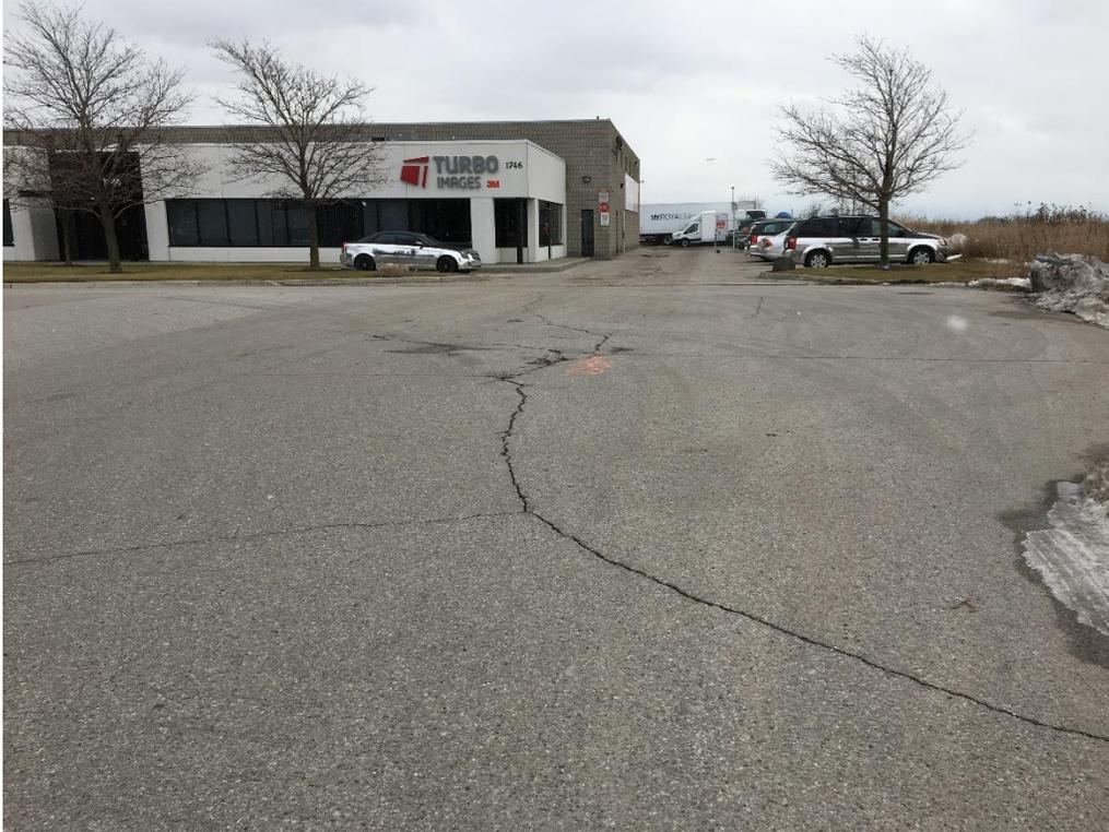
**Photo 16: Localized Random Cracking (Moderate Severity)- Menkes Dr**
