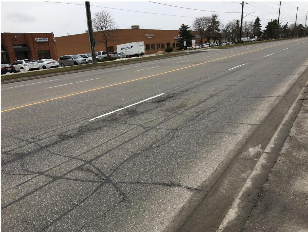
**Photo 4: Localized Potholes and Cracking (Slight to Moderate Severity)-Bramalea Road WB**
