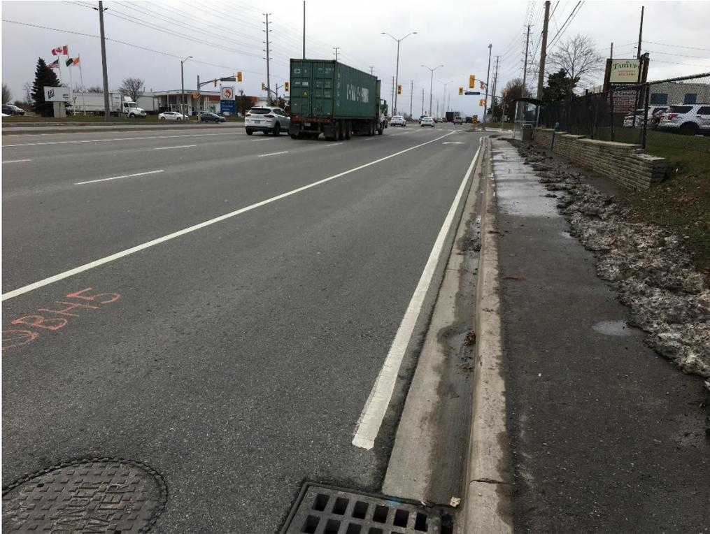
**Photo 20: Ravelling (Low Severity)- Derry Road E SB**
