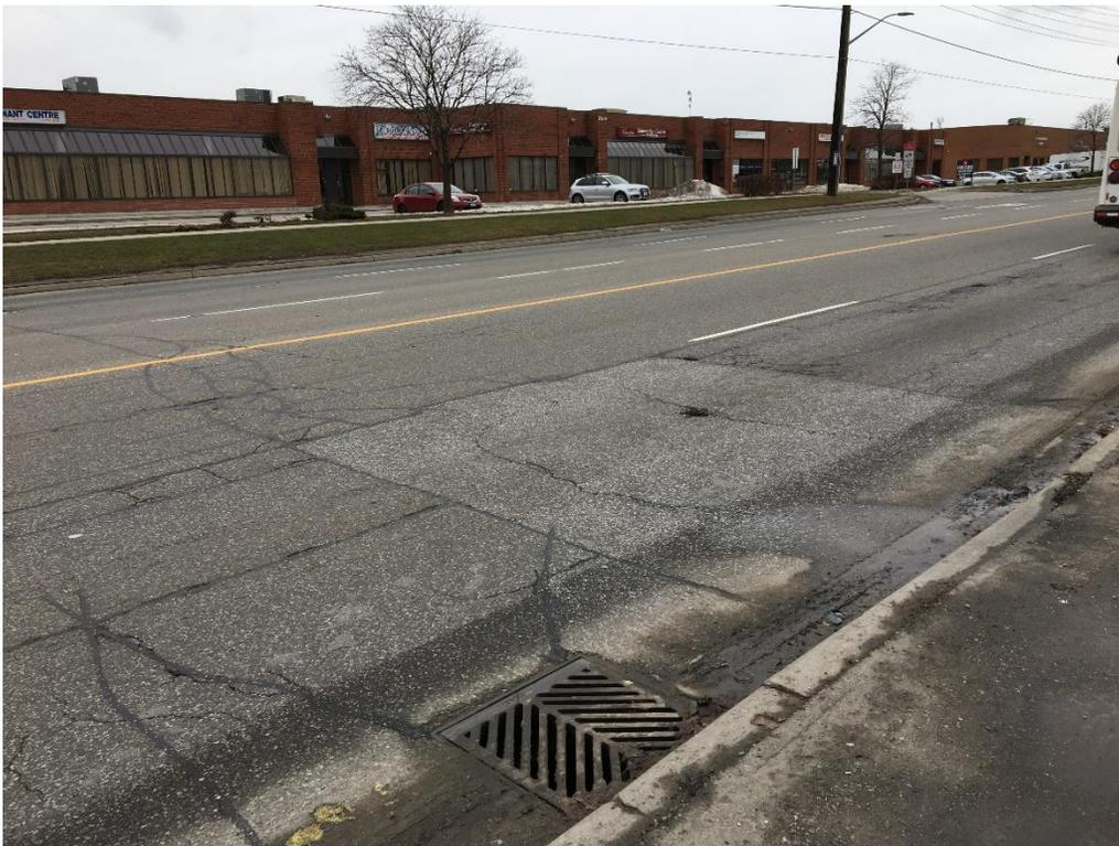
**Photo 2: Localized Patch and Alligator Cracking (Slight to Moderate Severity)- Bramalea Road WB**
