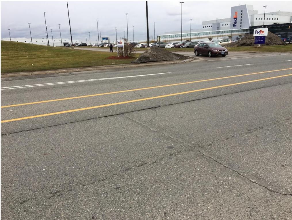
**Photo 10: Transverse and Longitudinal Cracking (Low to Moderate Severity)-Bramalea Road WB**
