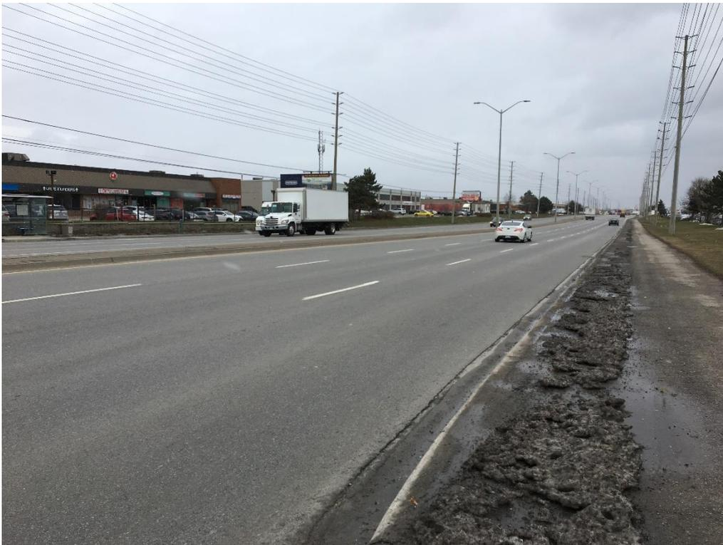
**Photo 19: Ravelling (Slight Severity)- Derry Road E NB**
