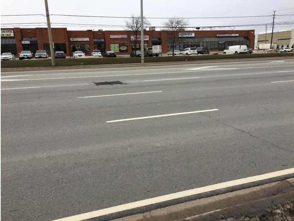
**Photo 13: Localized Transverse Cracking (Slight Severity)- Derry Road E NB**
