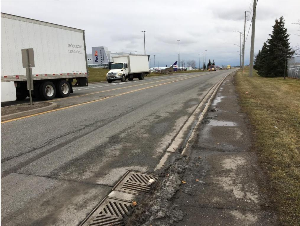
**Photo 9: Transverse and Longitudinal Cracking (Slight to Moderate Severity)-Bramalea Road EB**
