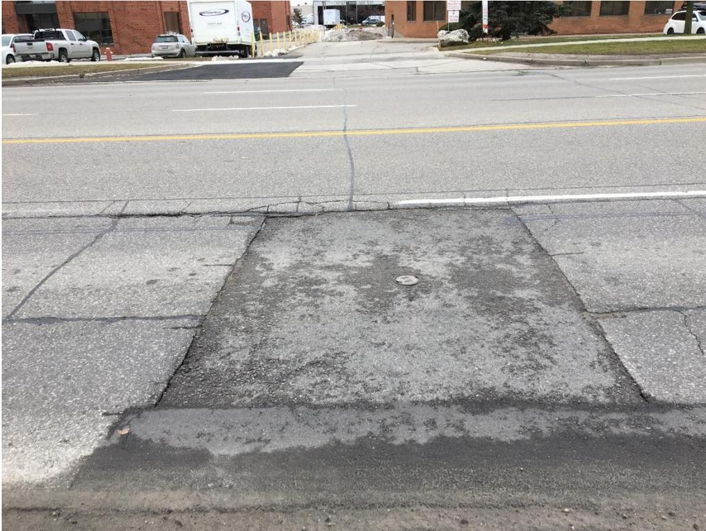
**Photo 5: Localized Patch Repair Due to Utility Repair- Bramalea Road WB**
