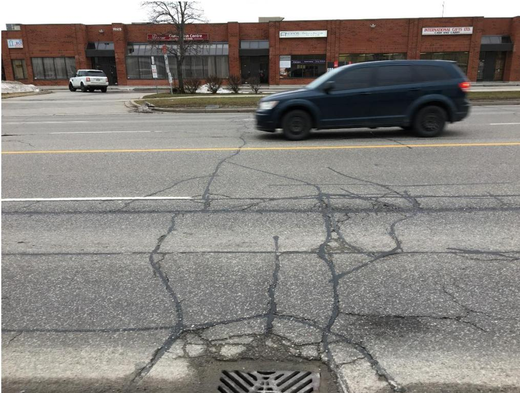
**Photo 3: Catch Basin Settlement and Transverse Cracking turning to Alligator Cracking (Slight to Moderate Severity)-Bramalea Road WB**
