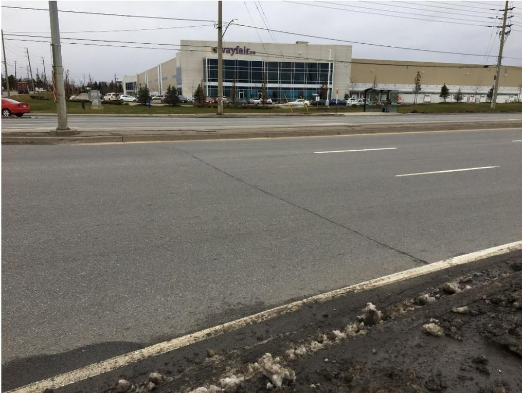
**Photo 11: Localized Transverse Cracking (Slight Severity)- Derry Road E NB**
