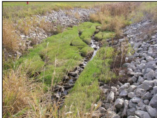
Site 12 facing downstream between northern limit of study area and Albion-Vaughan Road crossing: note rip rap substrates and mixed instream vegetation (short & tall grasses, cattails)
