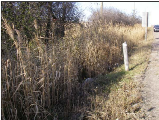
Site 3 upstream (west) of Highway 50 facing north at culvert and ditch
