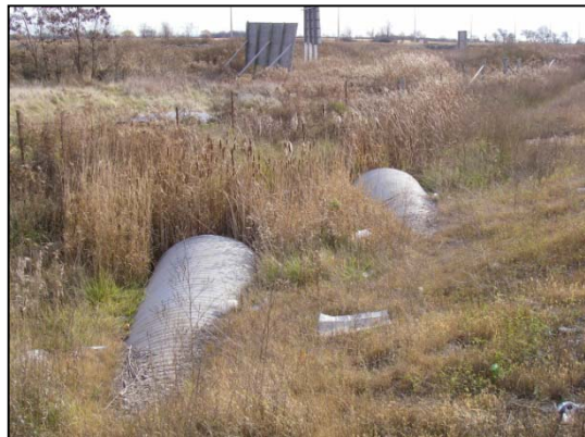
Site 10 downstream (east) of Highway 50 facing southeast at right-of-way and downstream habitat
