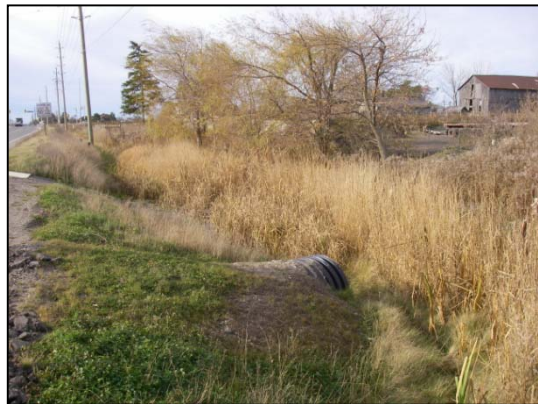
Site 17 upstream (north) of Mayfield Road facing northwest at roadside ditch
