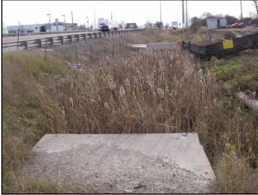
Site 11 facing downstream (south) from downstream end of Mayfield Road culvert
