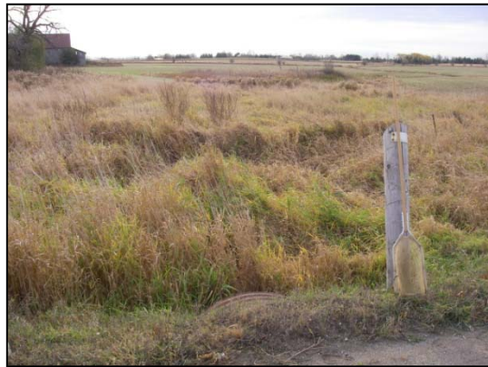
Site 16 downstream (south) of Mayfield Road at natural area and downstream agricultural fields
