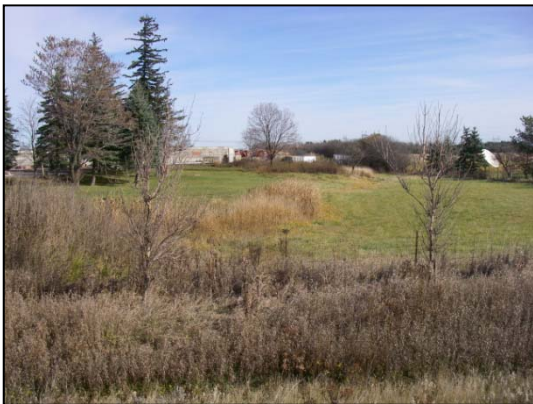
Site 4 channel downstream of berm culvert facing east over berm
