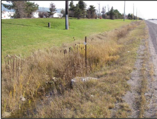
Site 1 upstream (east) of Highway 50 facing south at ditch
