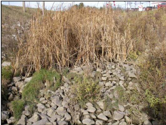
Site 12 facing upstream (north) from Albion-Vaughan Road culvert at rip rap rock check that allows only diffuse flow through when water conditions are low
