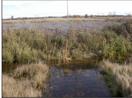
Site 8 downstream (east) of Highway 50 facing east at pooled area within and outside of right-of-way and berm and fill area outside of right-of-way
