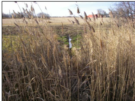
Site 3 upstream (west) of Highway 50 right-of-way facing west at channel leading to culvert
