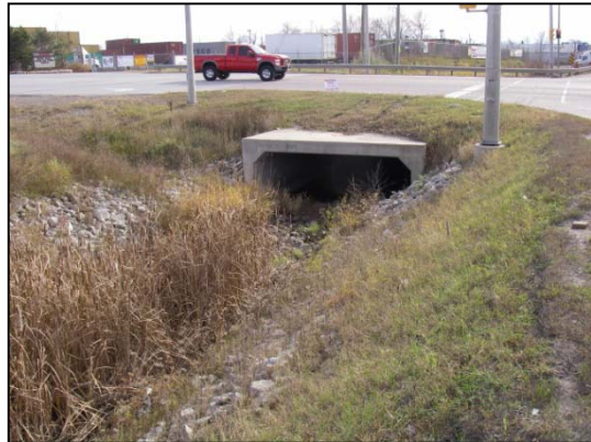
Site 12 facing downstream (south) at upstream end of Albion-Vaughan Road culvert
