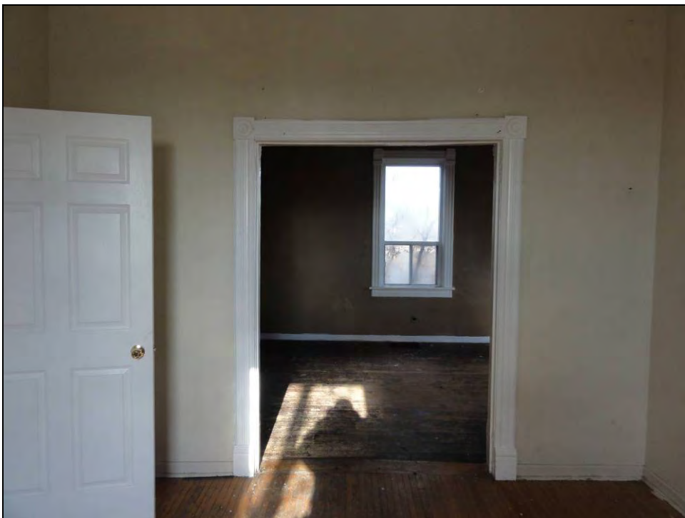
Plate 22: View of the parlour from the den, looking north.
