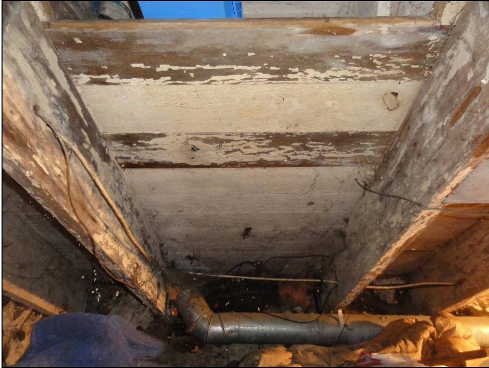
Plate 35: Detail of sawn joists supporting floor boards.
