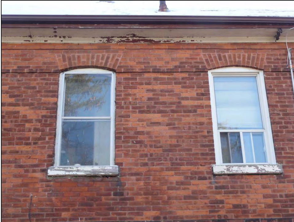
Plate 13: Typical example of modern windows, segmentally-arched brick voussoirs, and wooden sills (second floor of the north elevation).
