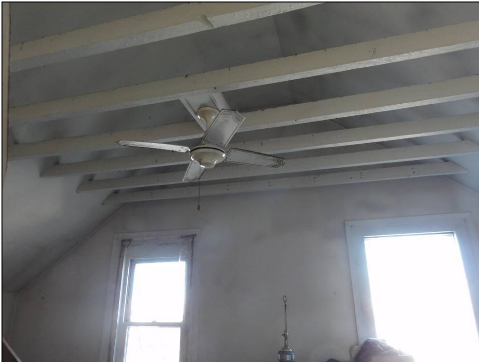
Plate 32: Exposed rafters located in north bedroom of second floor.
