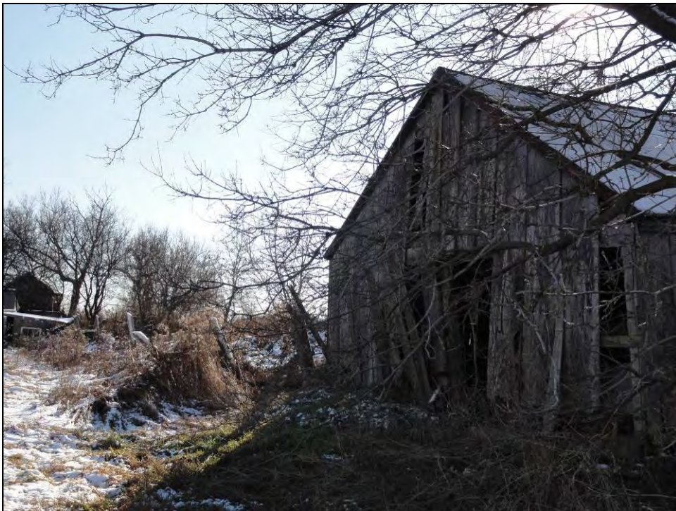
Plate 66: East elevation of the driveshed.
