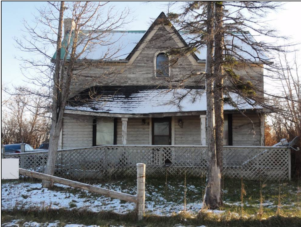
Plate 1: West elevation (front façade).
