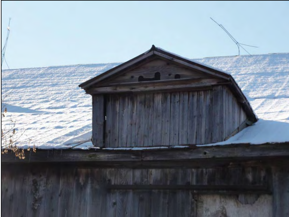
Plate 55: Gable dormer on east elevation of barn.
