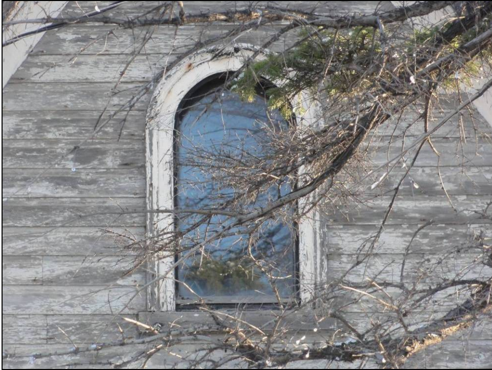
Plate 17: Detail of round-headed window in gable dormer on front façade.
