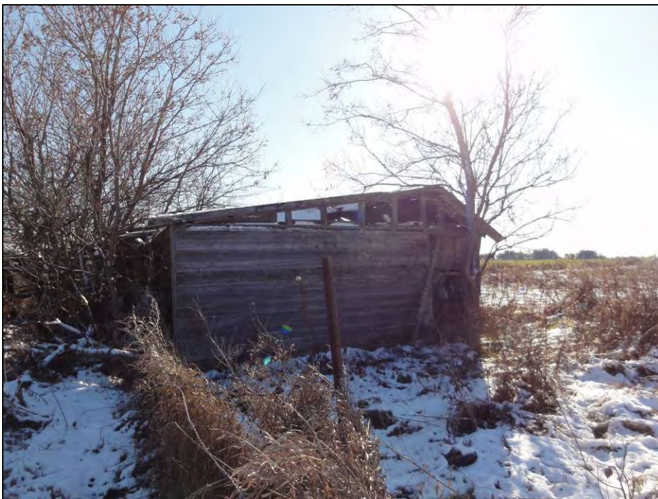
Plate 70: North elevation of the frame shelter.
