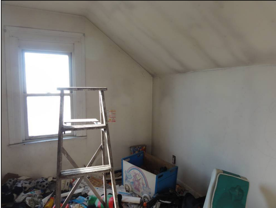
Plate 33: Bedroom located on the south side of the house.
