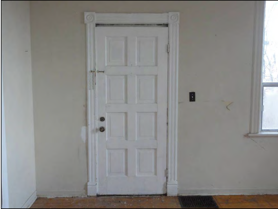
Plate 21: Decorative front door on east wall of the den.
