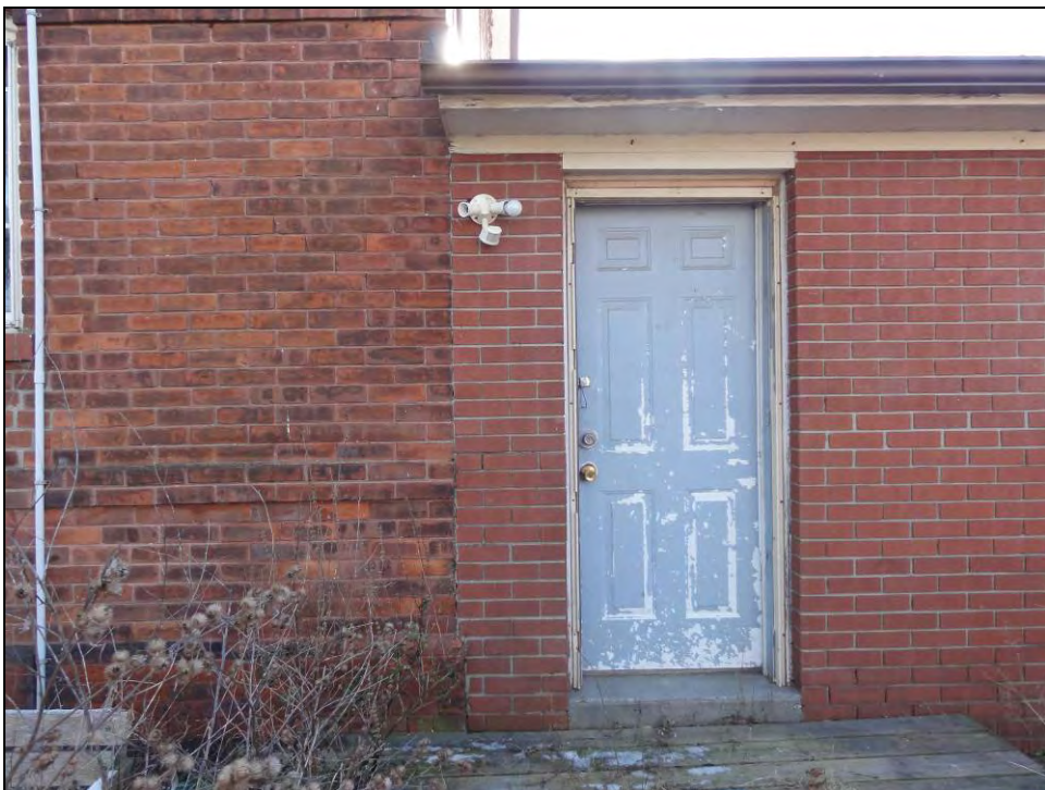
Plate 12: View of side entrance located on north elevation of the modern accretion. Note the change in brickwork between front and back sections of the house.
