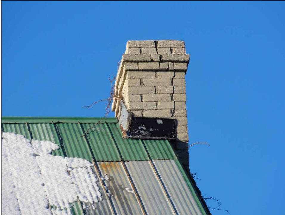
Plate 7: Detail of metal roofing material and chimney at north gable end.
