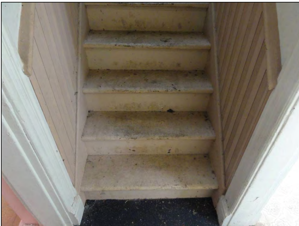
Plate 50: Detail of stairs leading from main floor to second floor.
