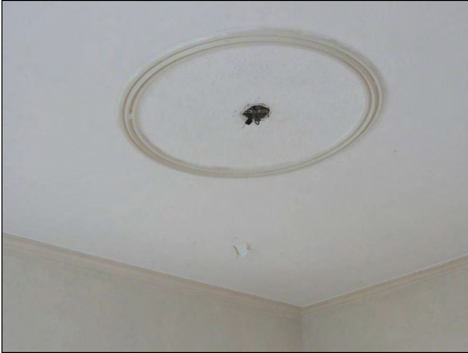
Plate 41: Decorative plaster ceiling in the den.
