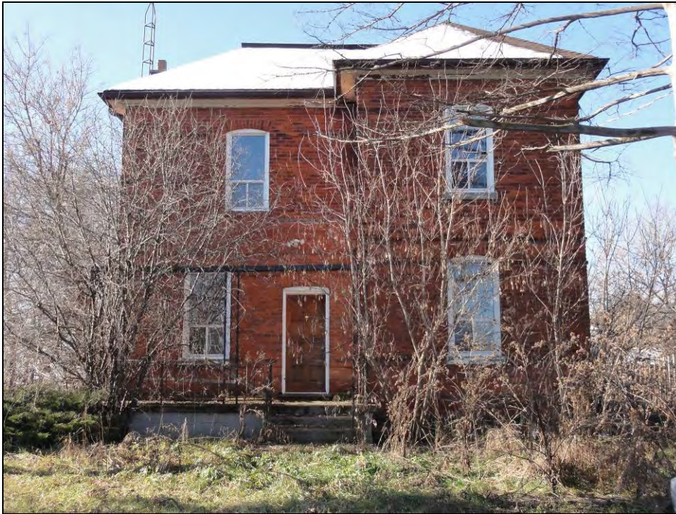
Plate 1: East elevation (front façade).
