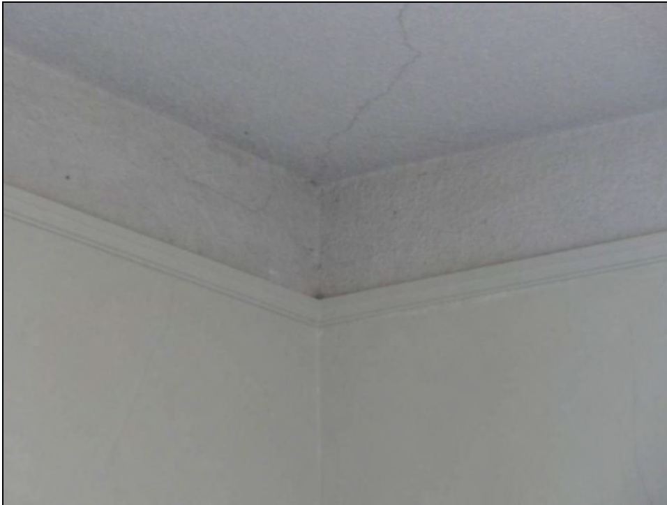
Plate 43: Detail of ceiling in Bedroom No. 2.
