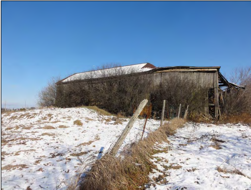
Plate 53: West elevation of barn.
