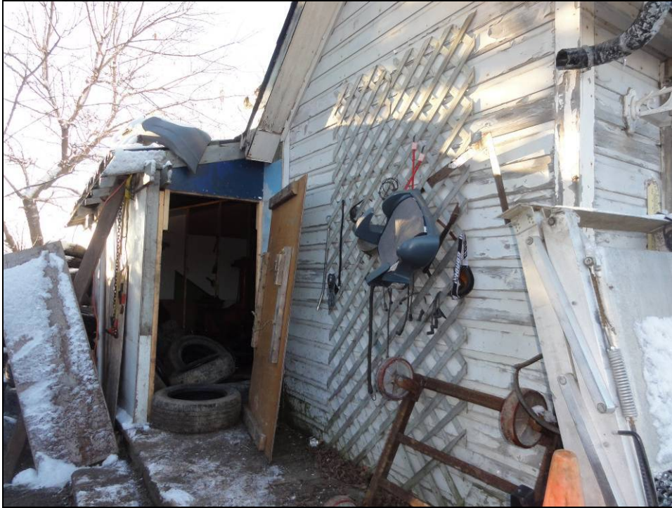
Plate 15: Entrance into modern, frame accretion located on rear elevation.
