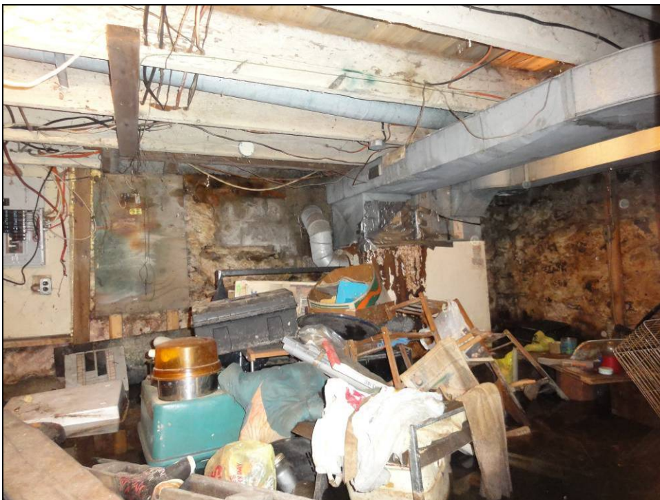
Plate 34: View of the basement, looking northeast.
