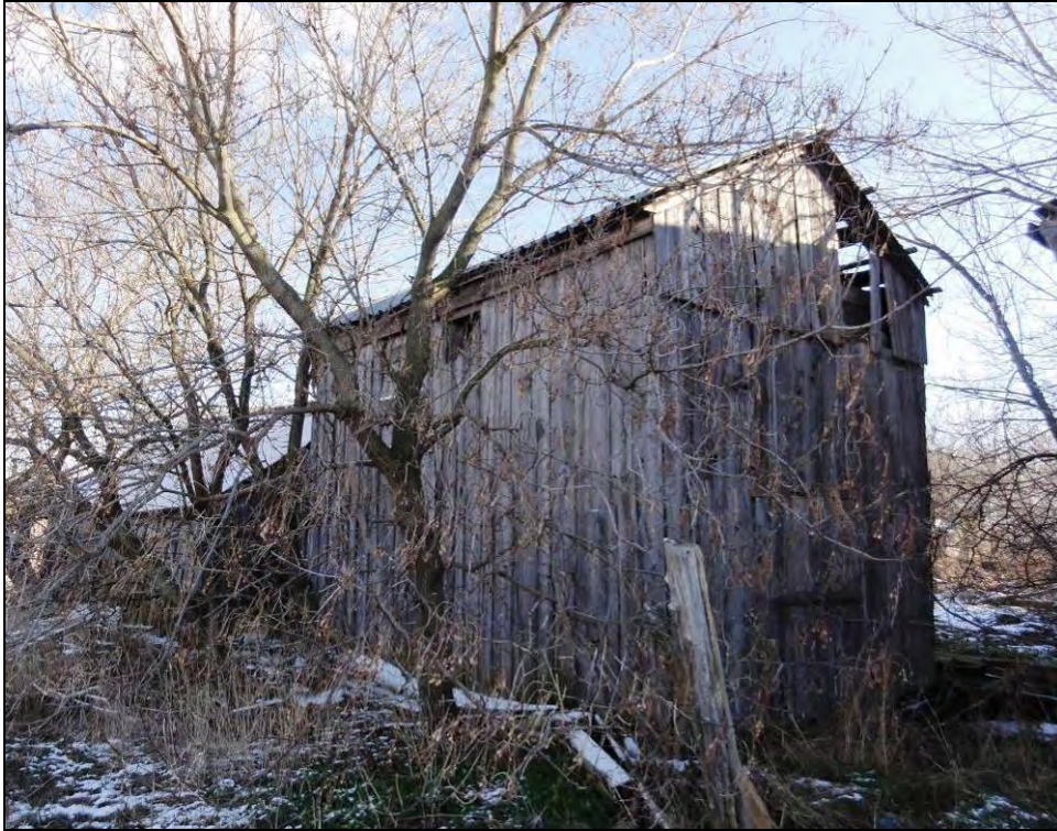
Plate 65: Northwest elevation of the two-storey henhouse.
