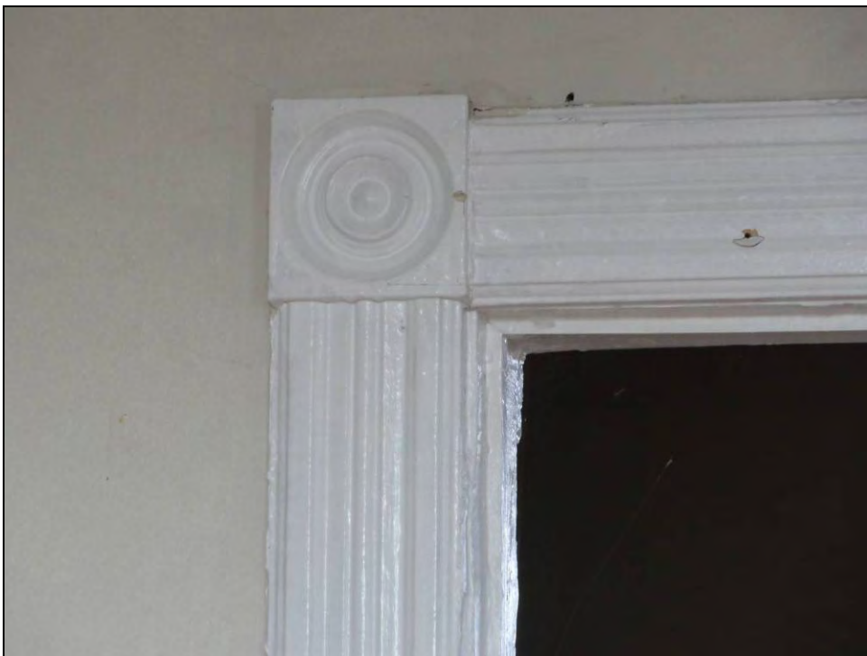
Plate 48: Bullseye rosette corner block and decorative casing around the door leading from the den into the parlour.
