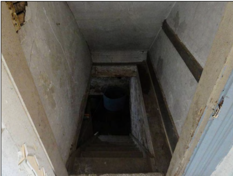
Plate 26: Looking down stairs to the basement.
