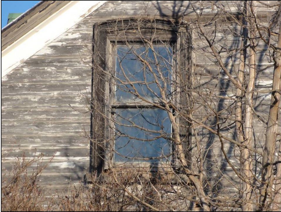
Plate 19: Representative one-over-one sash window in original decorative casing.
