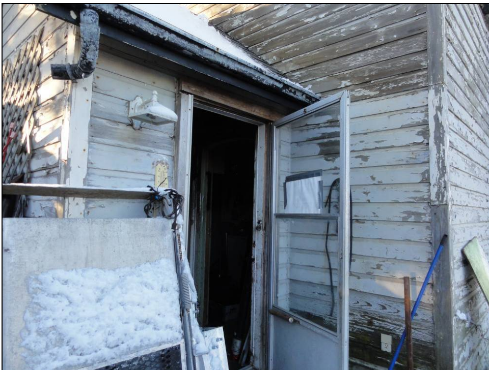
Plate 12: Rear entrance into the vestibule, located on the east elevation.
