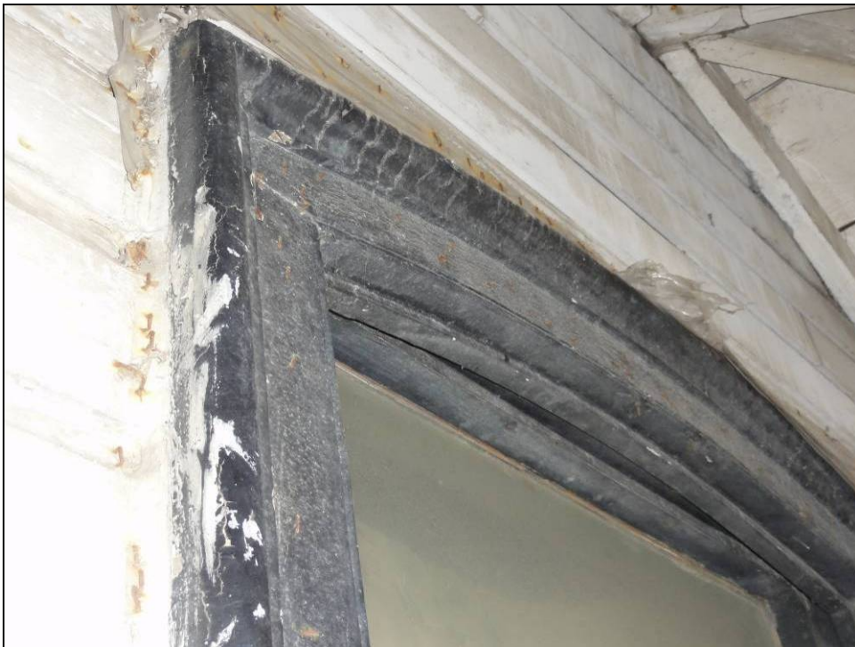
Plate 22: Detail of segmentally-arched window opening with decorative casing.
