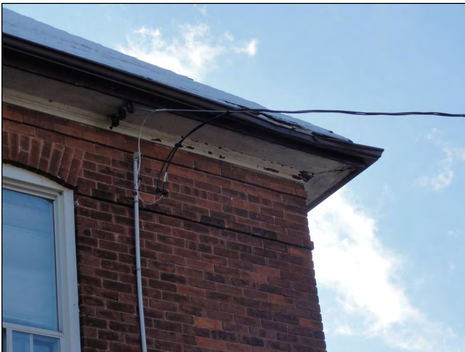
Plate 8: Detail of the brickwork, minimal roof overhang, and wooden soffit.
