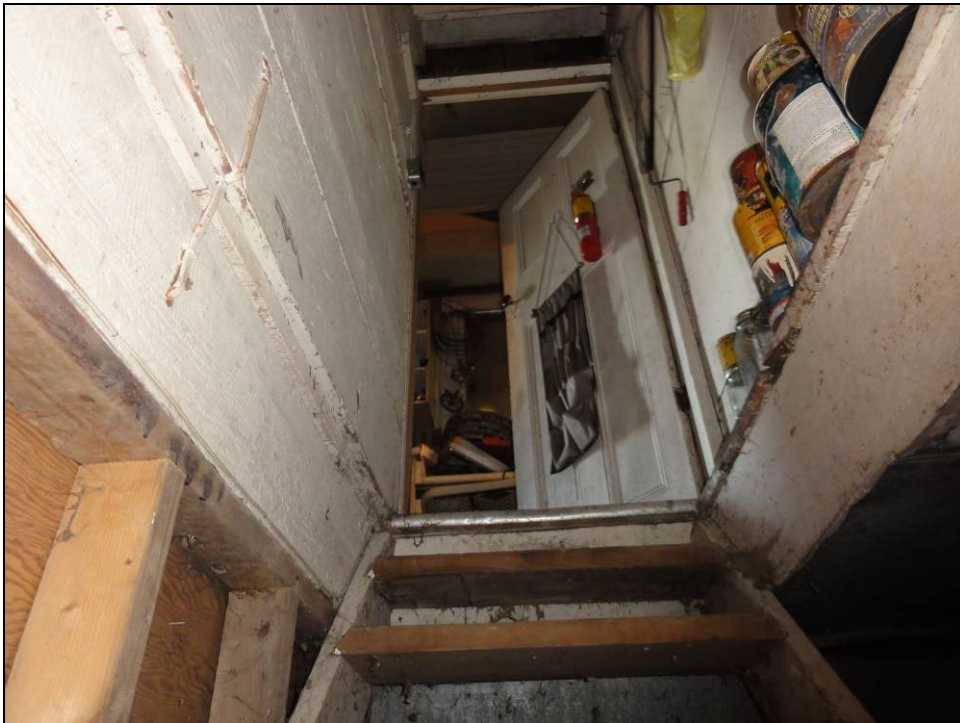
Plate 36 View up the stairs to the entrance into the basement.
