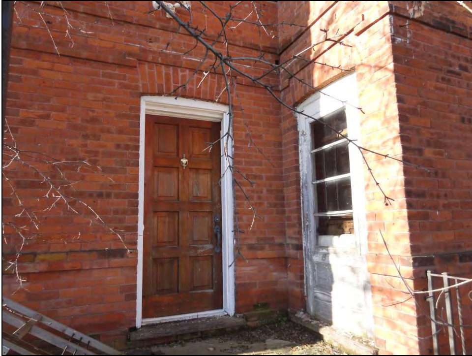
Plate 11: View of two front entrances on east elevation of house.
