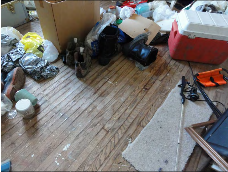
Plate 39: Floorboards located in Bedroom No. 1.
