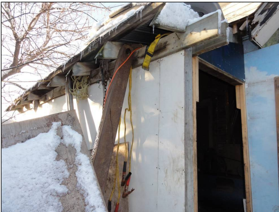
Plate 16: Detail of lean-to addition on rear elevation.
