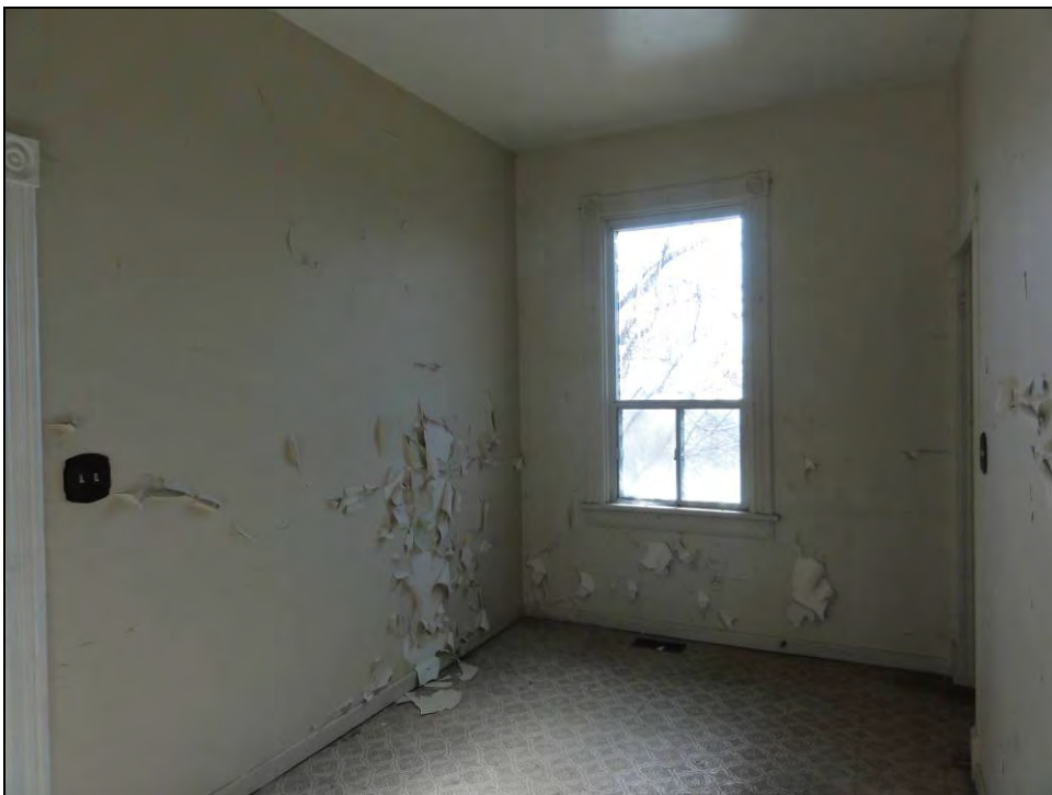
Plate 24: View of the dining room, looking south.
