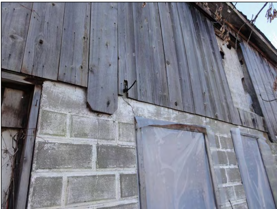
Plate 56: Concrete block foundations on east elevation.
