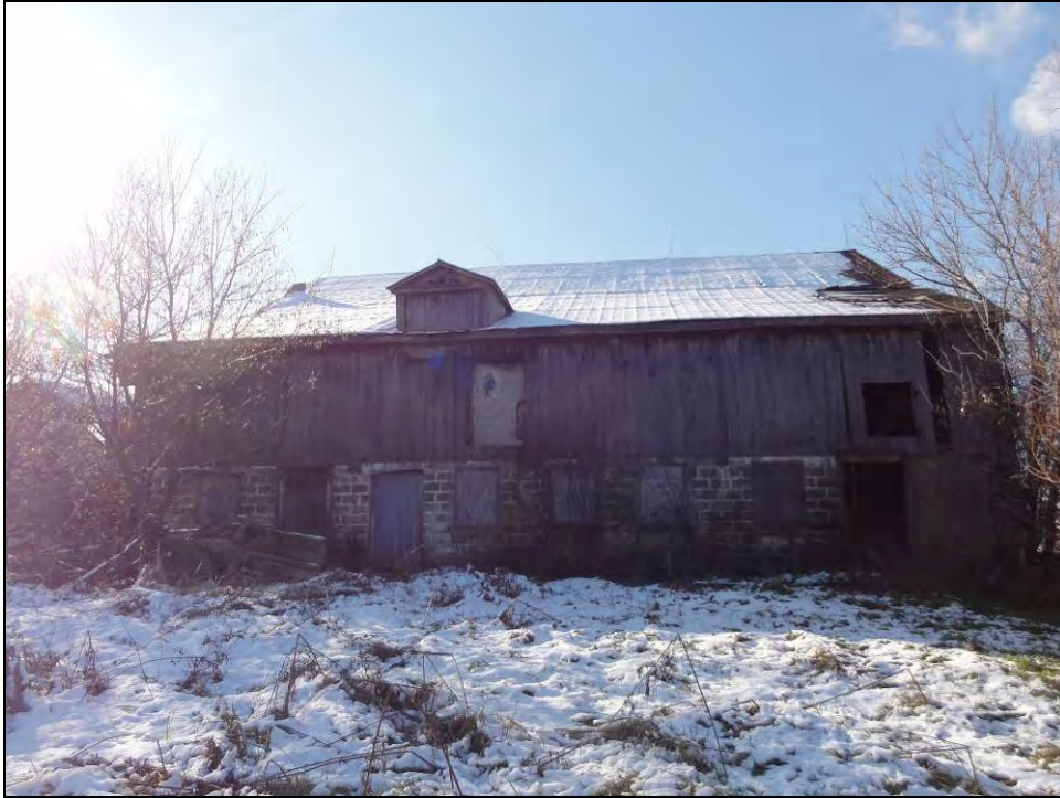
Plate 51: East elevation of barn.
