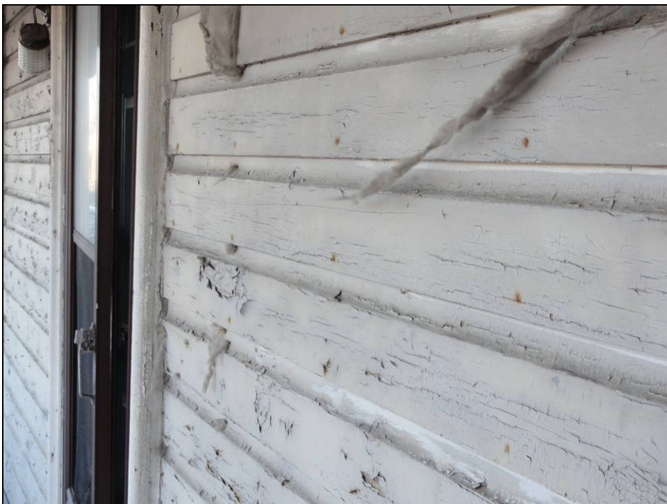
Plate 6: Detail of white painted clapboarding, front elevation.
