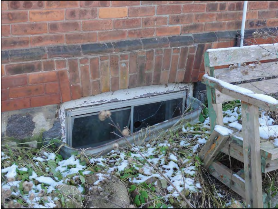
Plate 15: Typical example of basement window with segmentally-arched brick voussoir, wooden frame, and modern window (north elevation).
