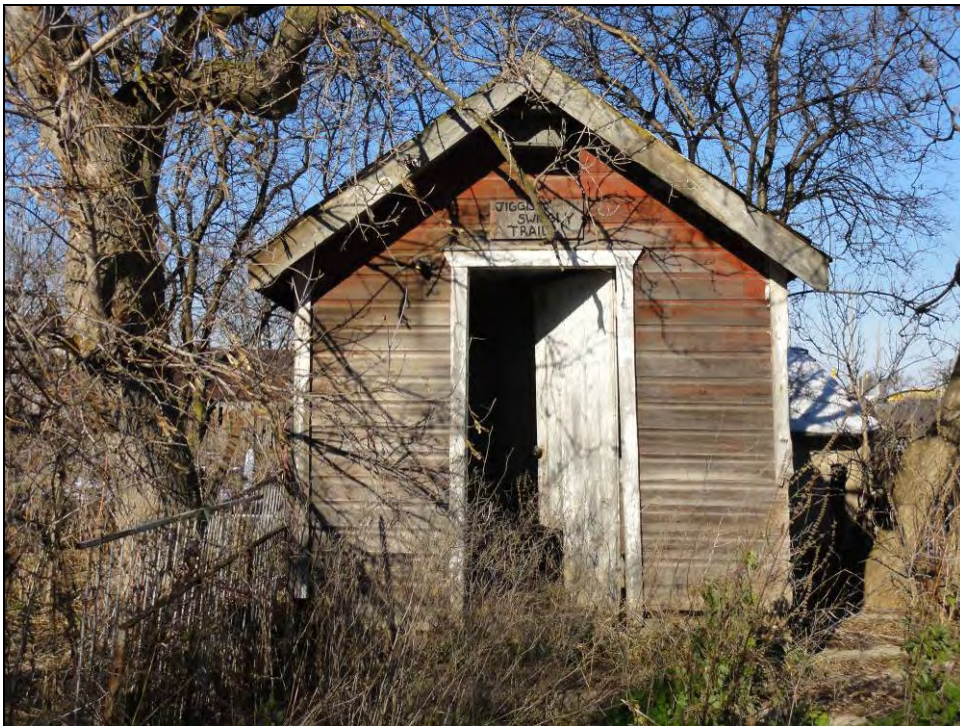
Plate 68: South elevation of the milk house.
