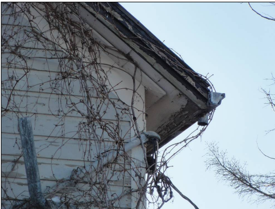
Plate 8: Detail of wooden soffits and fascia.
