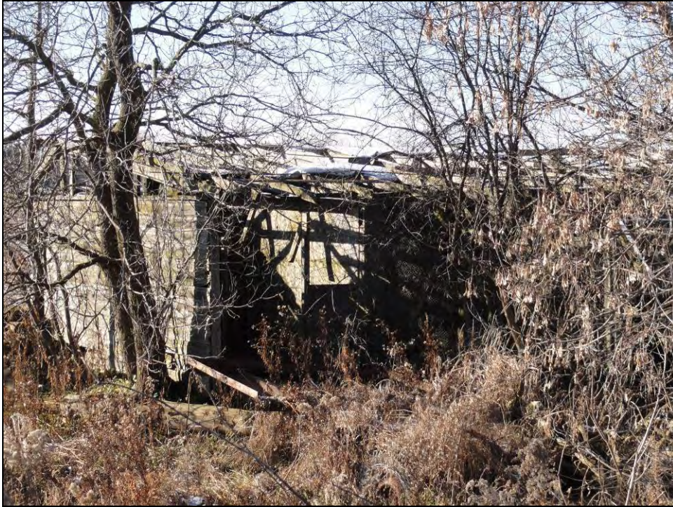
Plate 71: East elevation of the frame shelter.
