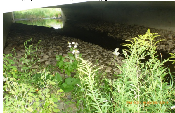
Looking upstream through crossing ↓
