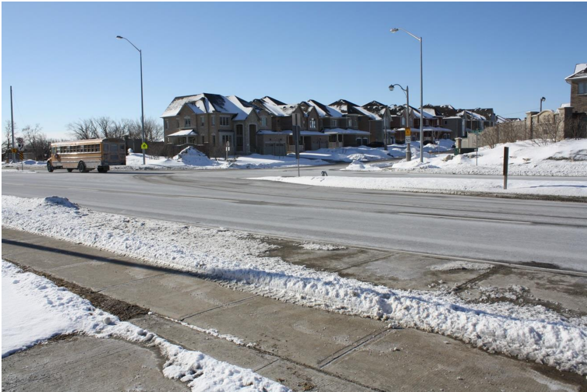
Figure A20 – No Defined Pedestrian Crossing Between Strathdale Road and Northbound Bus Stop – Section between Castle Oaks Crossing and Gardenbrooke Trail / Pannahill Drive
