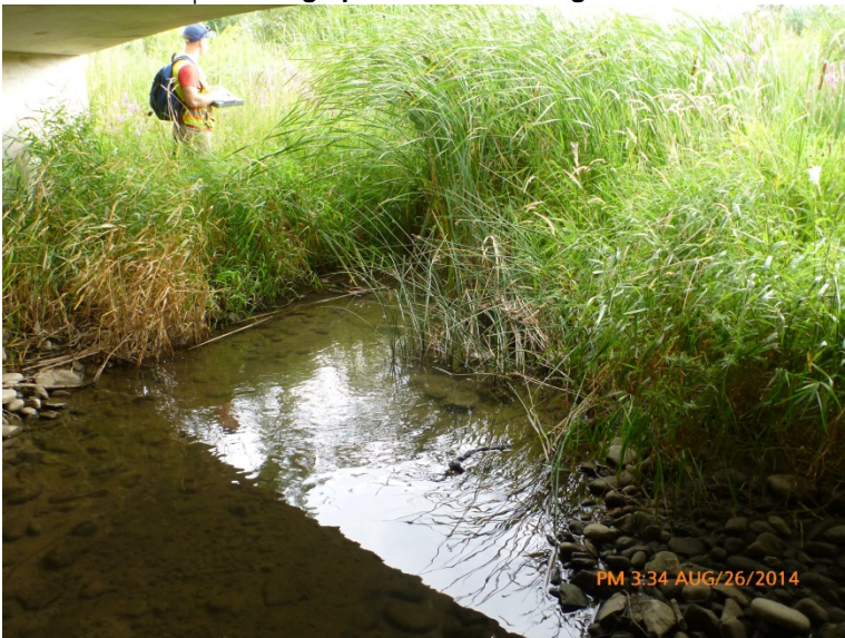
↑ Looking downstream at crossing outlet
