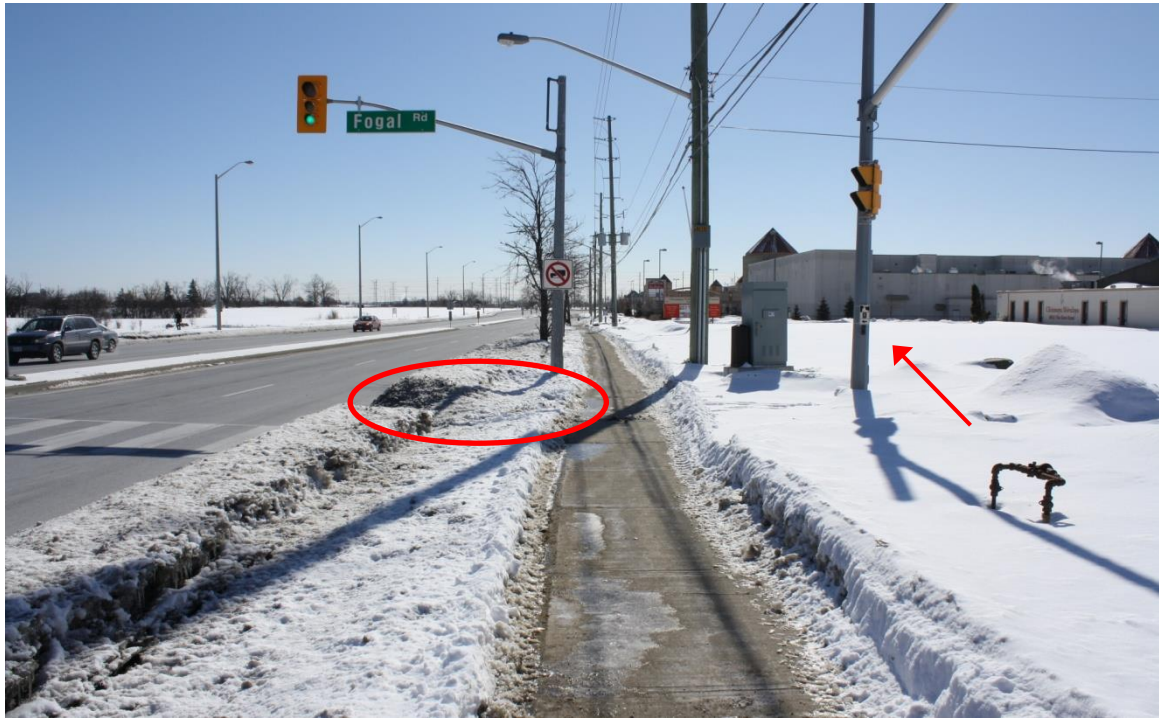
Figure A33 — Unusual Placement of Pedestrian Push-Button Device (without Snow Clearing) and Poor Snow Clearing on Sidewalk Access to Crosswalk – Intersection of The Gore Road and Fogal Road (Southwest Corner)
