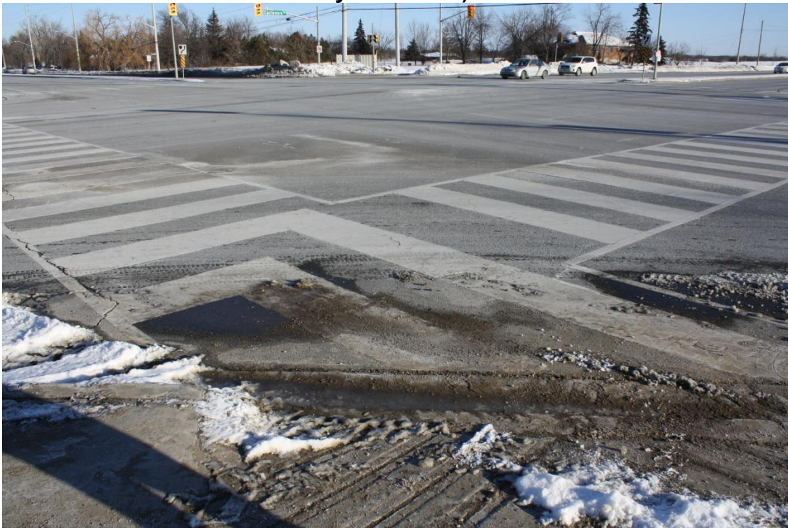
Figure A2 – Crosswalks Intersecting in Travelled Portion of Roadways – Intersection of Castlemore Road and The Gore Road (South-West Corner)
