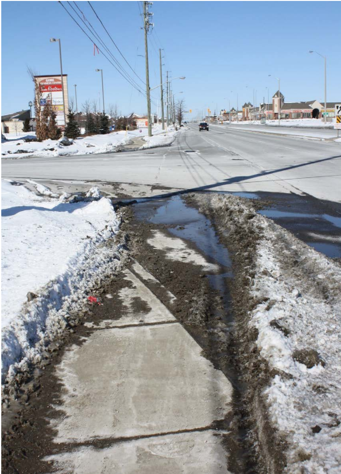
Figure A34 – Sidewalk South of Driveway and Associated Curb Ramp for Section Plowed Not Aligned with Sidewalk North of Driveway – Section between Fogal Road and Queen Street
