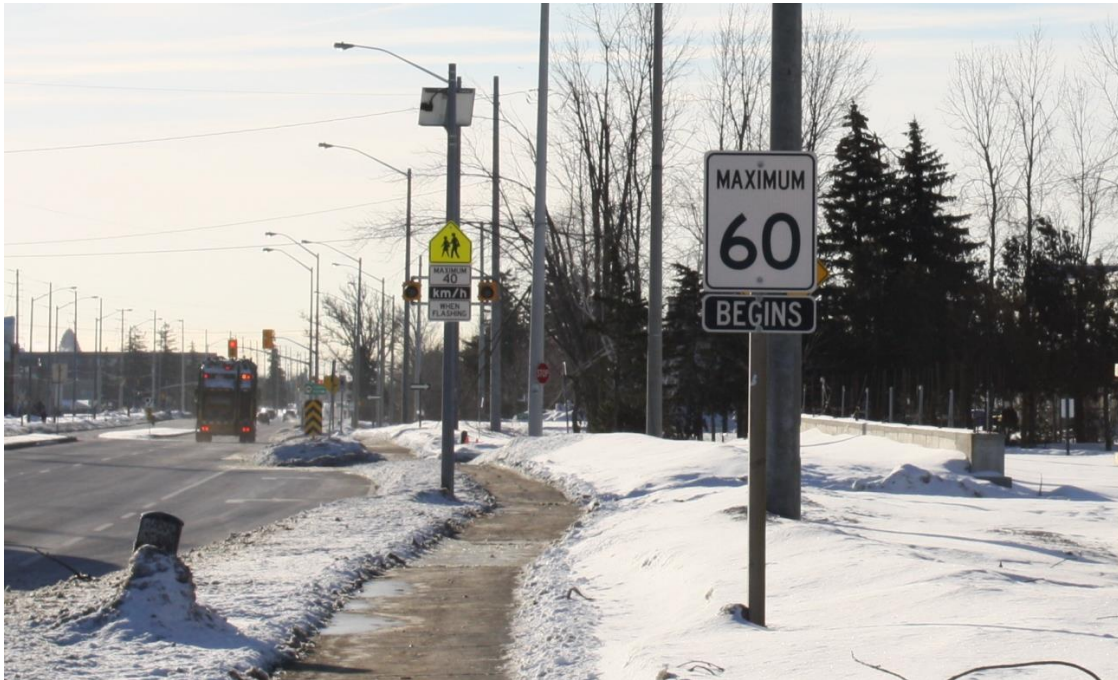
Figure A5 – Too Many Regulatory and Warning Signs - Section between Castlemore Road and Castlemore Public School Intersection
