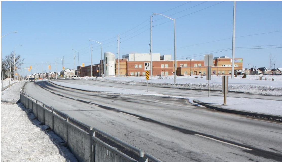
Figure A19 – Openings within Raised Medians – Section between Castle Oaks Crossing and Gardenbrooke Trail / Pannahill Drive
