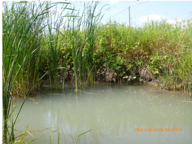
↑ Undercut RB DS of crossing
