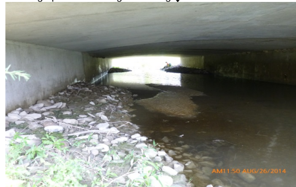
Looking upstream through crossing ↓
