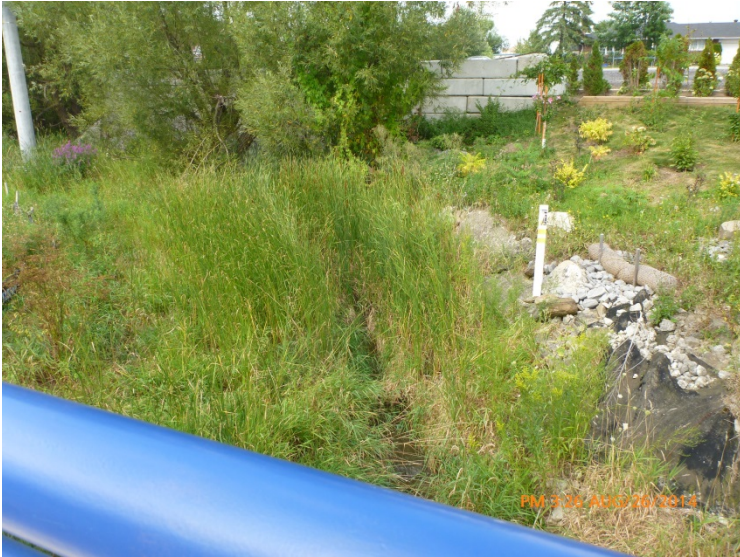
↑ Looking upstream from bridge deck
