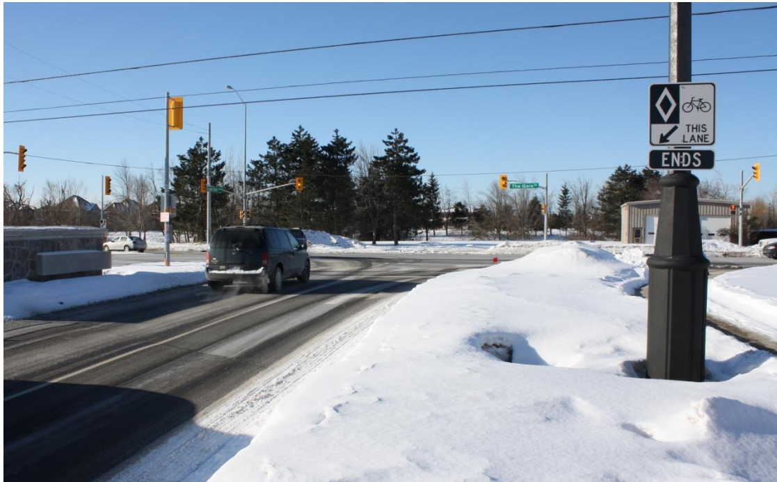
Figure A14 – On-Road Bike Lane Buried under Snow and Improperly Positioned to the Right of a Right-Turn Lane – Intersection of The Gore Road and Castle Oaks Crossing
