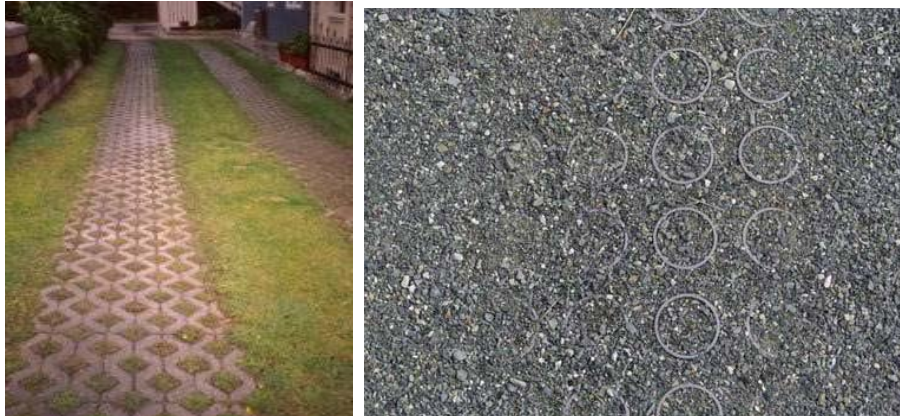
Residential driveway (Source: R. Bannerman); Plastic grid filled with gravel (Source: Gravelpave ® )
