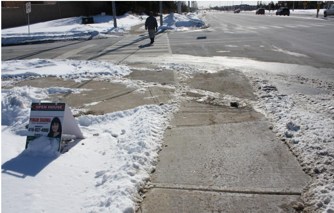
Figure A27 – East Sidewalk and Curb Ramp Not Aligned with Related East Crosswalk – Intersection of The Gore Road and Eastbrook Way / Eastview Gate (Northeast Corner)
