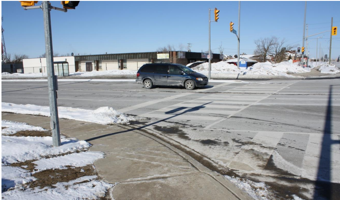
Figure A24 – Crosswalks Intersecting in Travelled Portion of Roadways – Intersection of The Gore Road and Cottrelle Boulevard (Southwest Corner)
