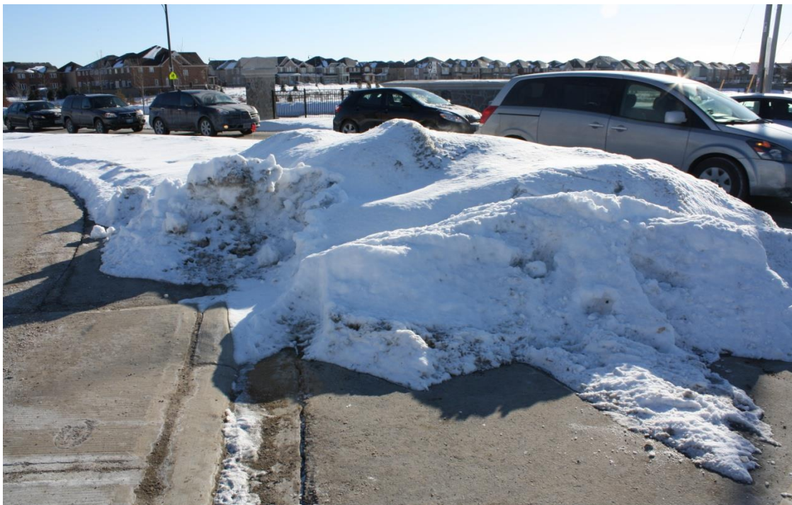
Figure A13 – Snow Bank on Pavement as Potential Sightline Obstruction – Intersection of The Gore Road and Castle Oaks Crossing
