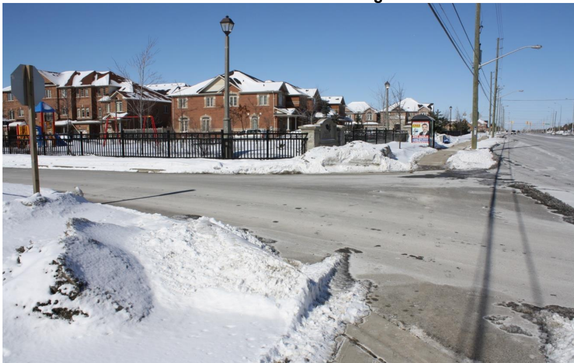
Figure A32 — No STOP Line or Crosswalk Pavement Markings at Royston Street – Section between Ebenezer Road and Fogal Road
