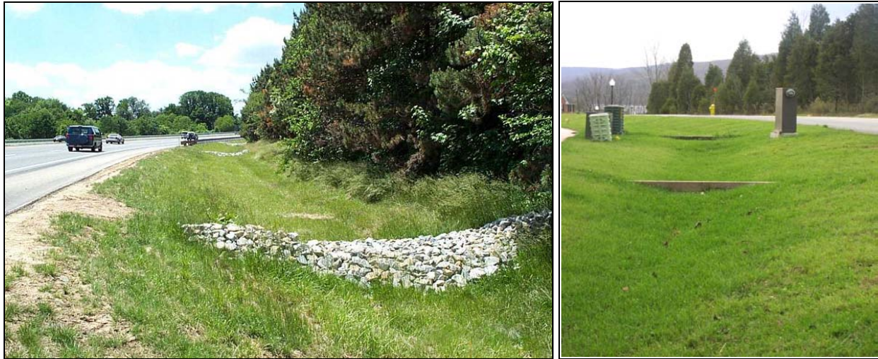
Figure 4.8.2 Enhanced grass swales feature check dams that temporarily pond runoff to increase pollutant retention and infiltration and decrease flow velocity
