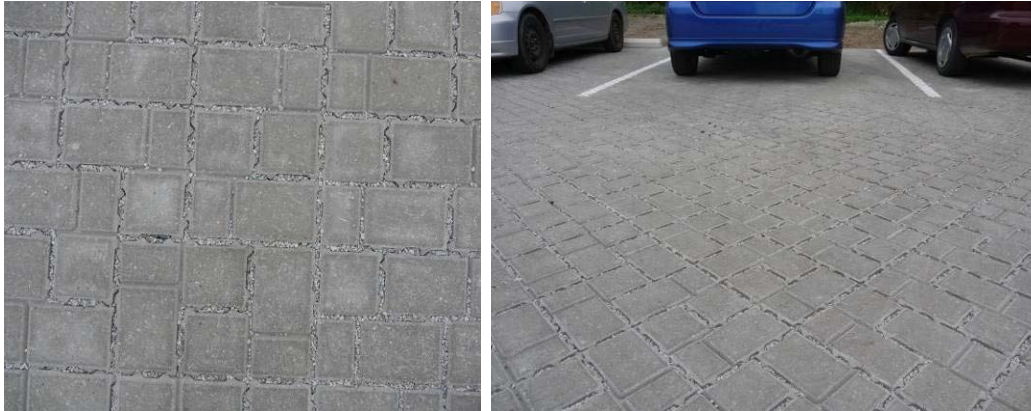
Permeable paver parking lot in Mississauga, ON (Source: CVC)
