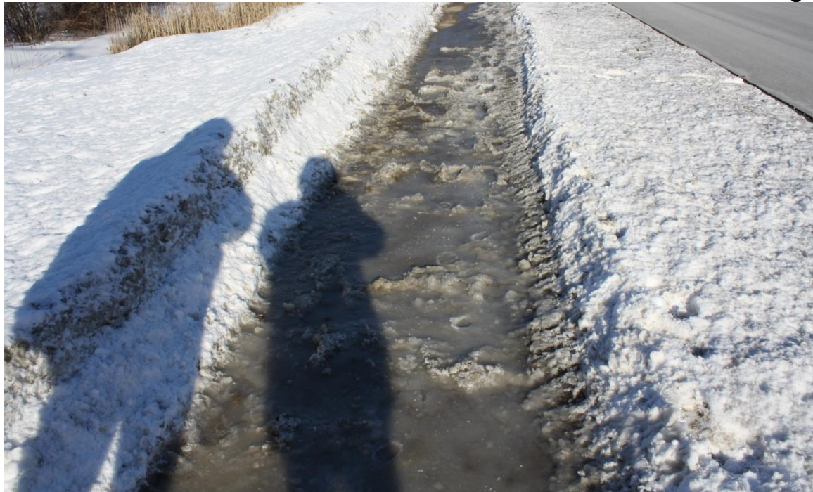
Figure A11 – Slippery Surface Conditions on West Sidewalk – Section between Castlemore Public School Intersection and Castle Oaks Crossing
