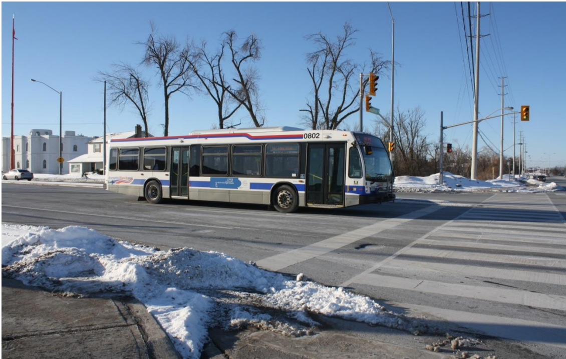
Figure A3 – Pedestrian Signal Head and Push-Button (Shown at Far End) Not Aligned with Edge of South Crosswalk
