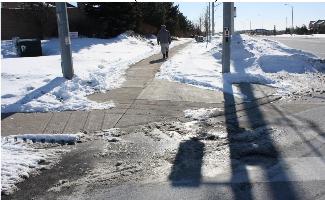
Figure A28 – Groove Marks Not Aligned with Related East and South Crosswalk – Intersection of The Gore Road and Eastbrook Way / Eastview Gate (Southeast Corner)
