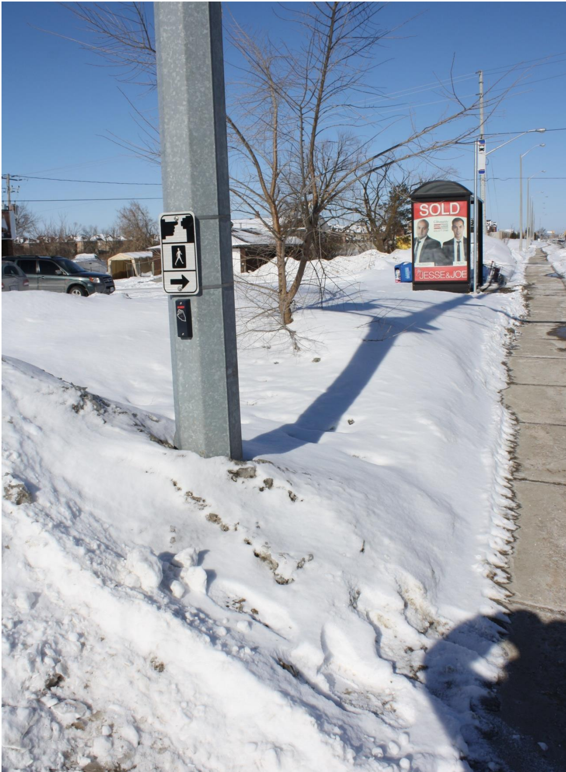
Figure A26 – Snow Pile Hampers Access to Pedestrian Push-Button – Intersection of The Gore Road and Cottrelle Boulevard (Northwest Corner)
