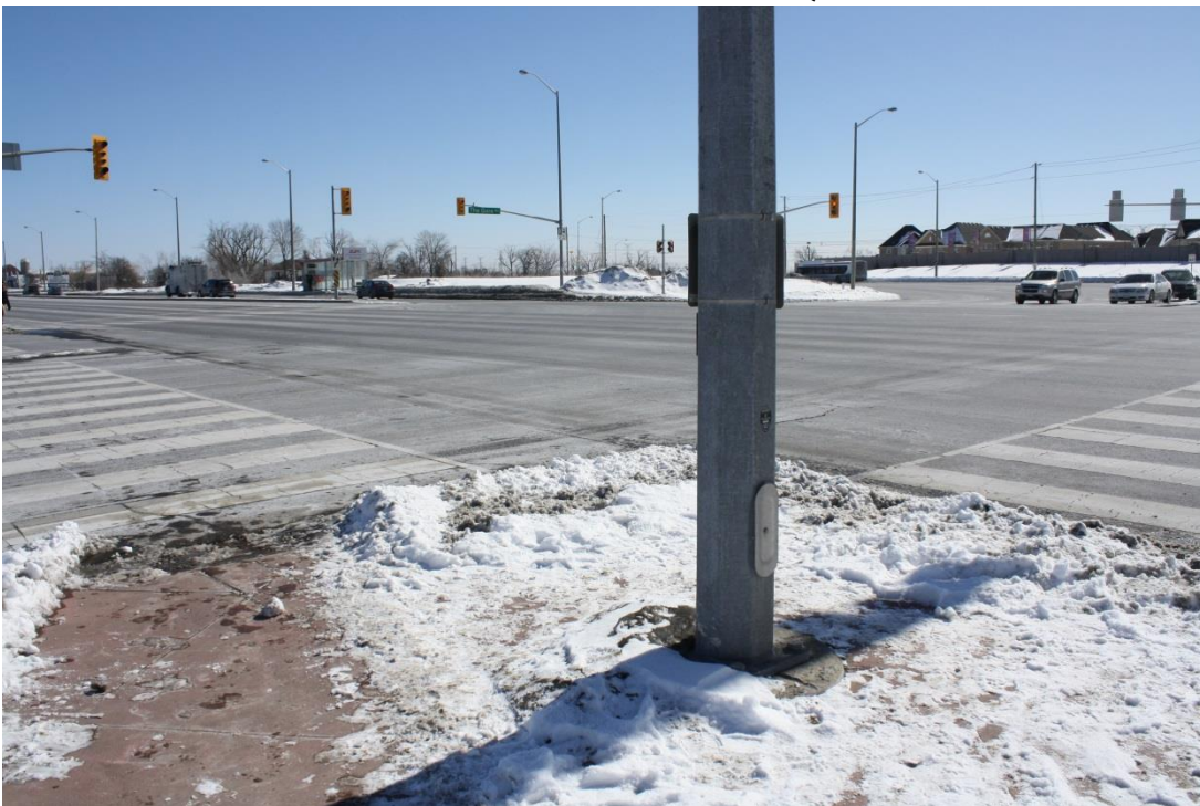
Figure A36 – Pedestrian Push Buttons Not Easily Visible From Crosswalk Across Channelized Right-Turn Lane – Intersection of The Gore Road and Queen Street (Northwest Corner)
