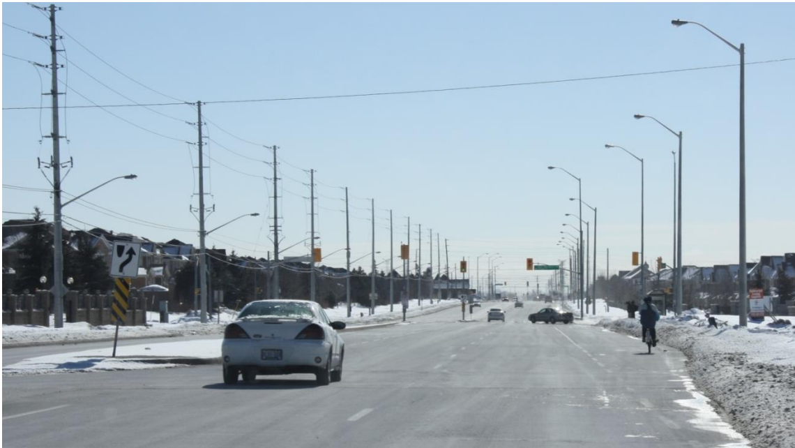
Figure A1 – Straight and Flat Alignment, Wide Through Lanes, and Expansive Right-of-Way (Looking South at North of Don Minaker Drive / Tyler Avenue)
