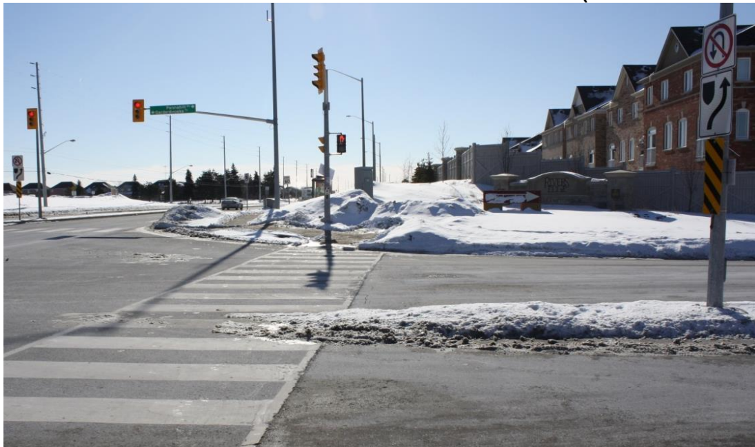
Figure A23 – No STOP Bar Marking on West Approach to Intersection – Intersection of The Gore Road and Gardenbrooke Trail / Pannahill Drive
