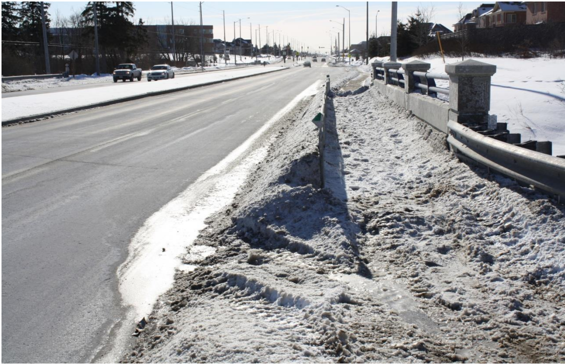
Figure A16 – Pedestrian Fencing Installation and Narrow Sidewalk Hampers Snow Clearing – Section between Castle Oaks Crossing and Gardenbrooke Trail / Pannahill Drive
