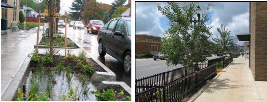
Source: left – City of Portland, BES; right – CVC.
