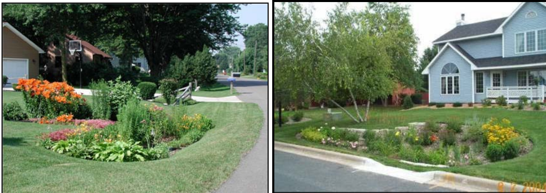
Left and Right - front yard rain gardens that takes runoff from the residential lot and street (Source: City of Maplewood, Minnesota)
