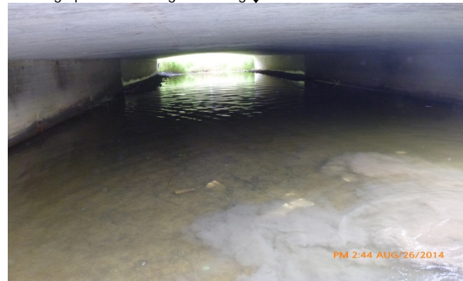
Looking upstream through crossing ↓
