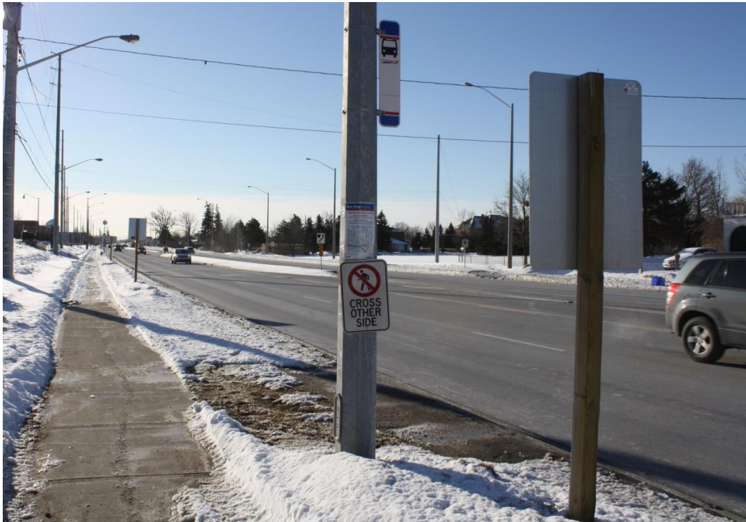
Figure A8 – CROSS OTHER SIDE Sign Not Facing Majority of Intended Pedestrian Audience – Castlemore Public School Intersection
