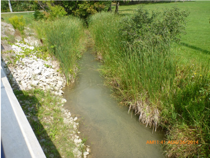
↑ Looking upstream from bridge deck
