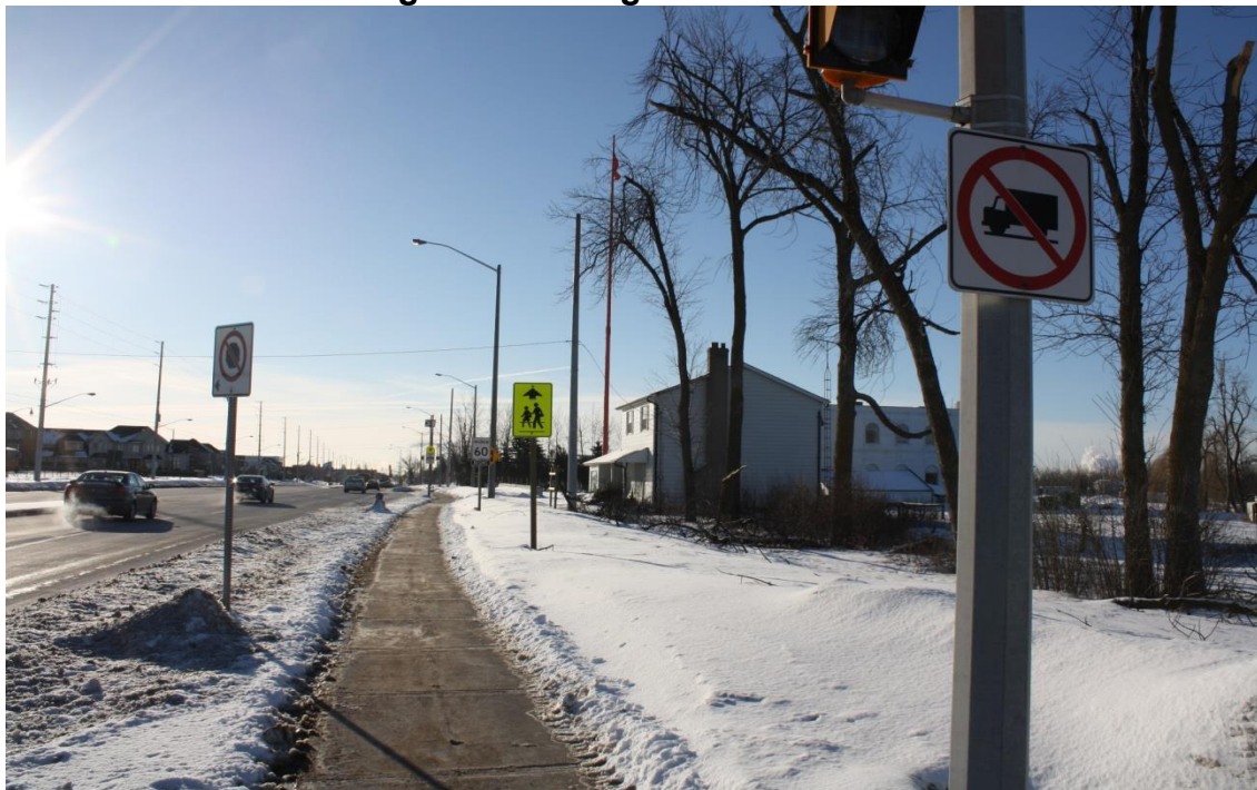
Figure A4 – Improper Positioning of MAXIMUM SPEED LIMIT BEGINS Sign – Section between Castlemore Road and Castlemore Public School Intersection
