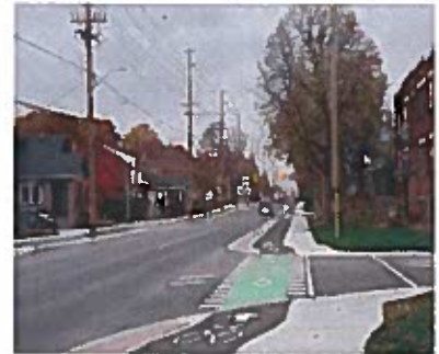
Example of Raised Cycle Track Source of Photo: City of Ottawa
