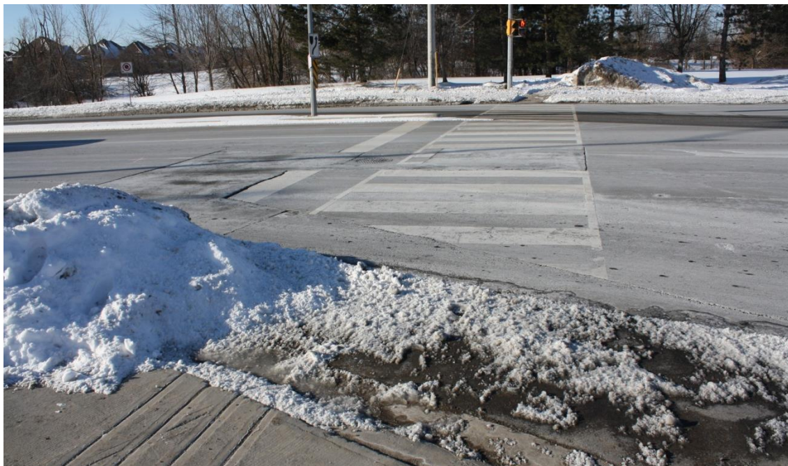
Figure A15 – Incomplete Crosswalk Pavement Marking – Intersection of The Gore Road and Castle Oaks Crossing
