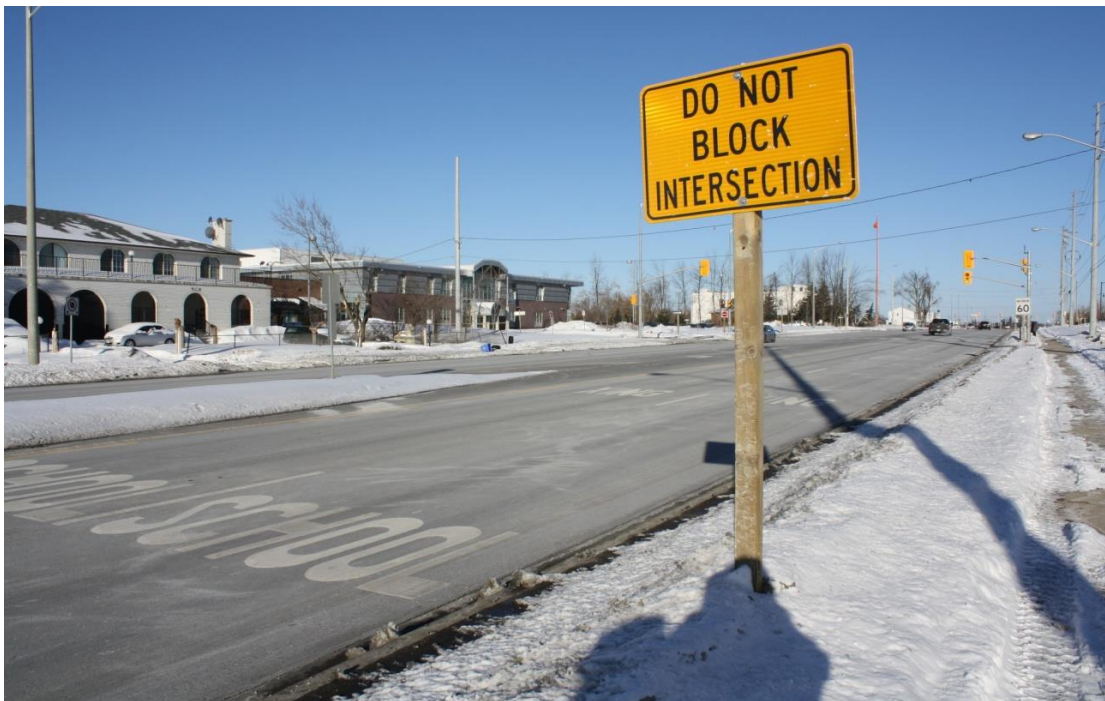
Figure A9 – Unnecessary DO NOT BLOCK INTERSECTION Sign and SCHOOL XING Pavement Markings – Section between Castlemore Public School Intersection and Castle Oaks Crossing
