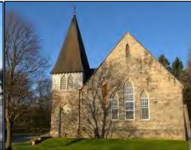
Belfountain Village Church
