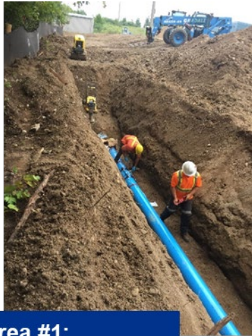
Area #1: Excavation for chlorine contact pipe
