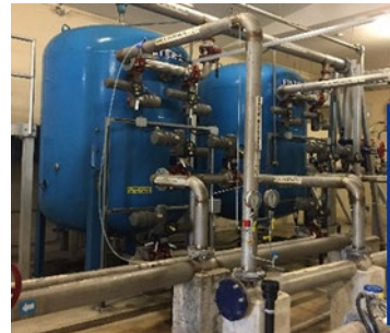
Area #2: Replace filters and piping inside existing building
