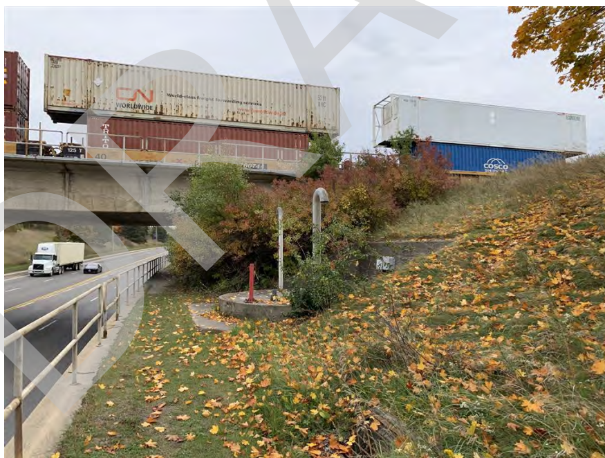
Image 6: View of buried infrastructure along west side of Finch Avenue West, within Proposed Design Alternative A, facing south. 20 October 2022
