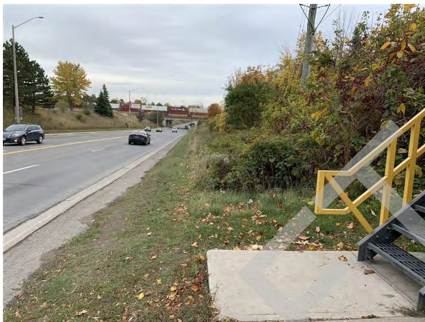
Image 5: View of slope on west side of Finch Avenue West, within Proposed Design Alternative A, facing south. 20 October 2022
