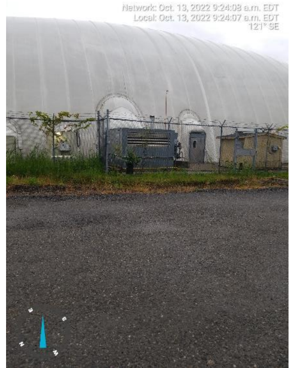
Photograph 16: View showing the western exterior of the soccer and sports dome and electrical transformer unit, from east of Finch Avenue West, facing east.
