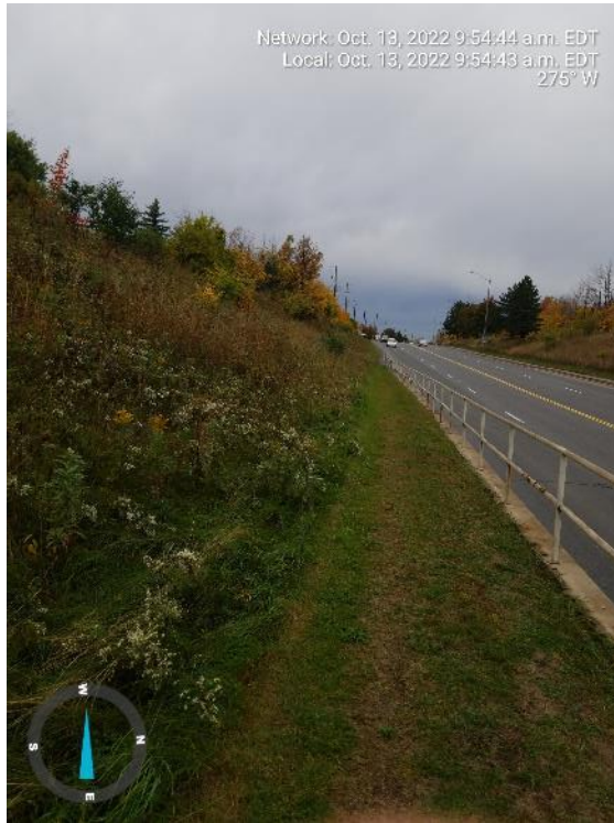
Photograph 7: Site area between wet well and control building, from the west side of Finch Avenue West, facing northwest.
