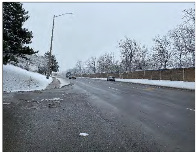
Image 6: View of the Finch Avenue West from the south end of the road looking south.
