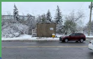
Finch Stormwater Pumping Station
