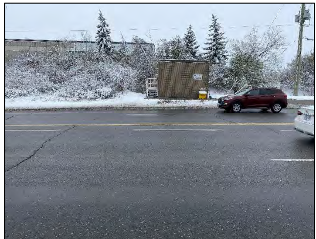
Image 2: View of Finch Avenue West looking west from the north end of the road. The existing SPS control building is visible.
