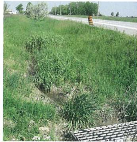
Figure 3. West ditch & DICB
