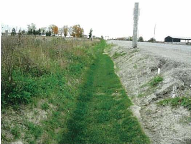
Figure 3. West Ditch facing Upstream
