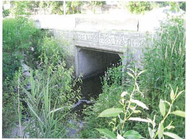
Figure 15. Upstream End of Crossing Culvert
