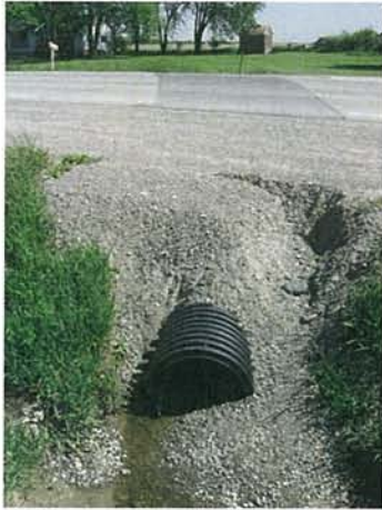
Figure 2. 600mm Crossing Culvert
