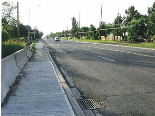
Figure 10. Crossing Culvert facing North
