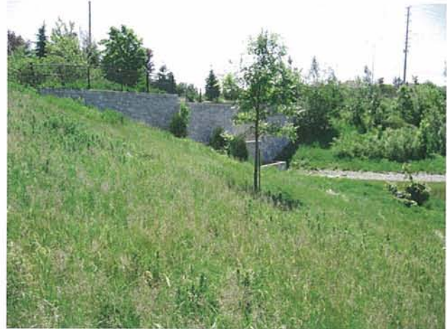
Figure 7. SWM Pond Outlet Structure
