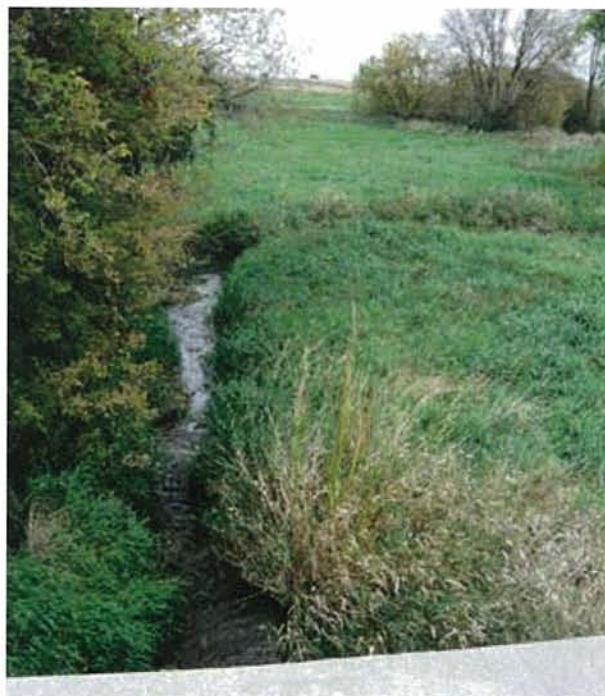
Figure 6. Downstream of Crossing 1
