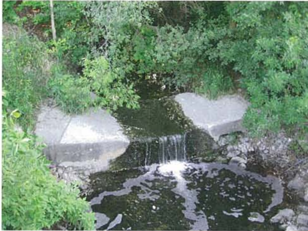
Figure 14. Weir upstream of Crossing
