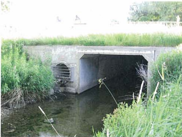
Figure 16. Downstream End of Crossing Culvert
