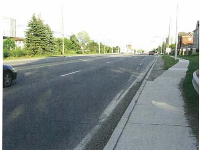
Figure 11. At Crossing Culvert facing South
