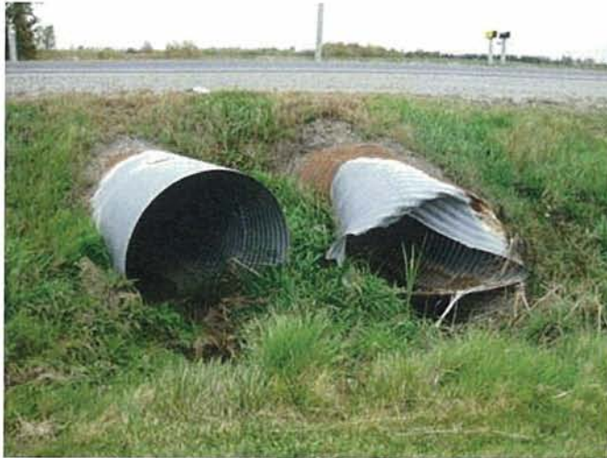
Figure 7. Upstream End of Crossing Culvert 2
