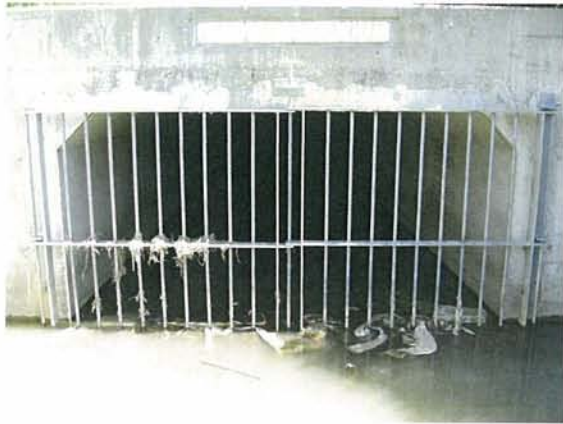
Figure 4. West end of Crossing Culvert
