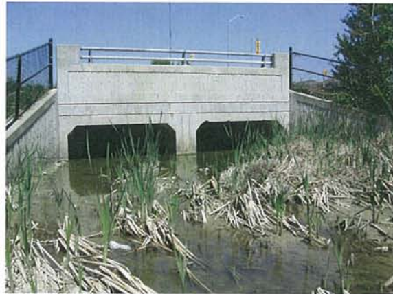
Figure 5. West Watercourse at Sandalwood Pkwy
