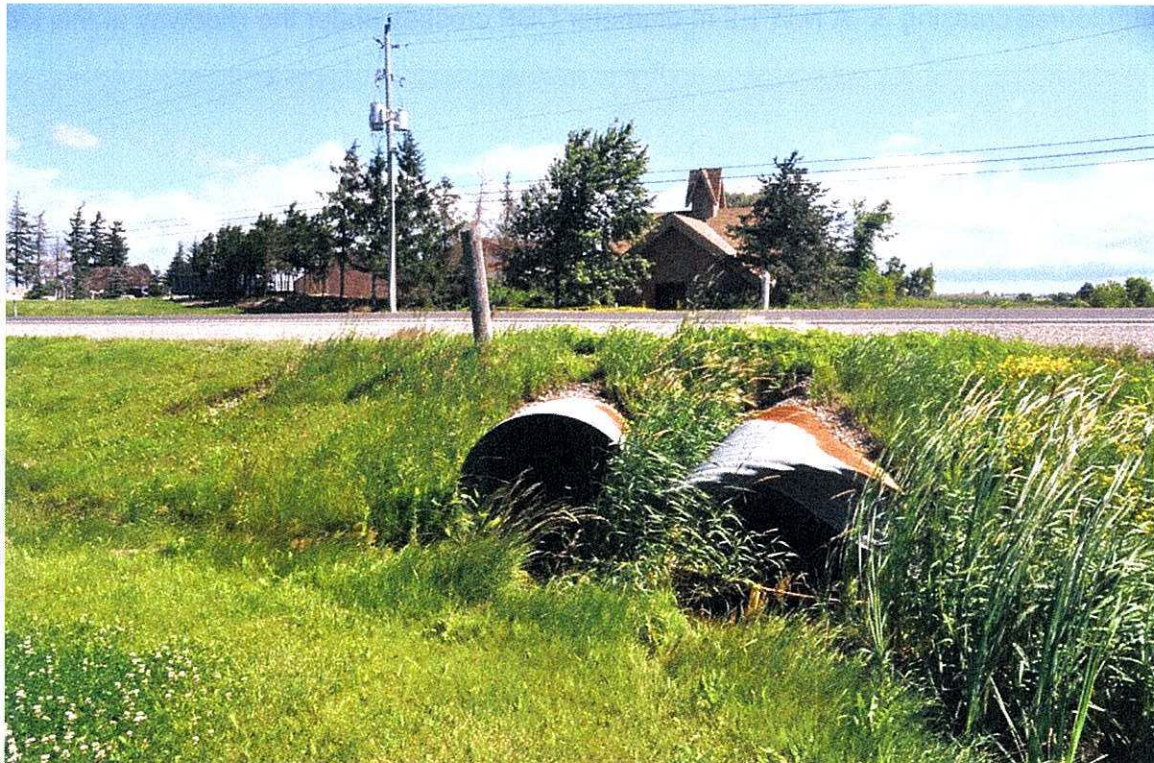
View upstream (above) at the West Humber tributary crossing and at damaged twin culvert inlet (below)
