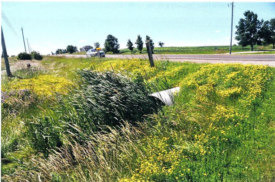
View downstream at the West Humber tributary channel (above) and partially obstructed culvert outlet (below)
