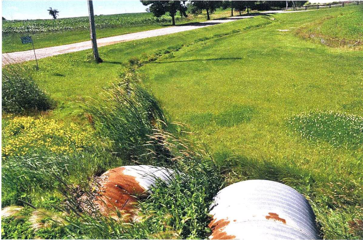
View upstream (above) at the West Humber tributary crossing and at damaged twin culvert inlet (below)
