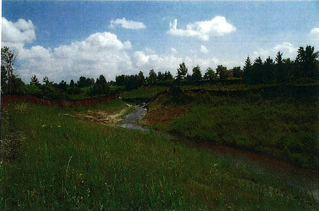
Another Etobicoke Creek tributary has been recently diverted south and west of Dixie Road
