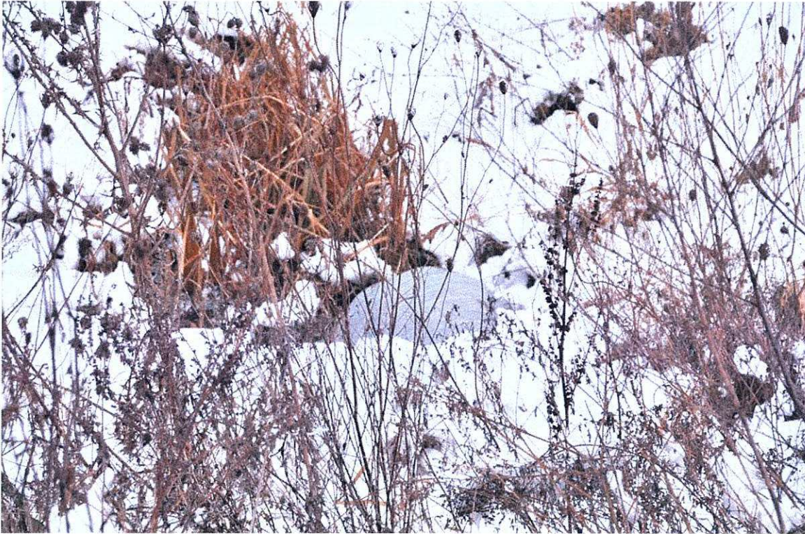
Again, the culvert outlet is almost obscured by vegetation
