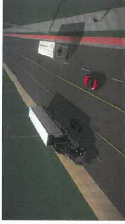
Existing 4 lane roadway
