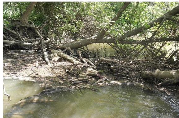
Photograph 12: Cold Creek (CC-01) 75 m downstream from King Street East crossing; looking downstream at the outer meander bend on the eastern side of the valley.
