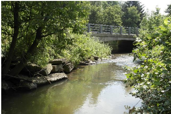
Photograph 3: Cold Creek (CC-01) 25 m upstream from Albion Vaughan Road crossing; looking downstream at the bridge at Albion Vaughan Road.
