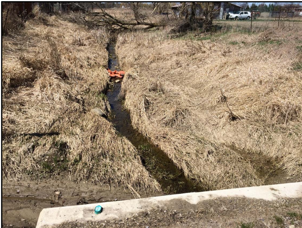
Photo 8: Crossing RB2 facing upstream.
