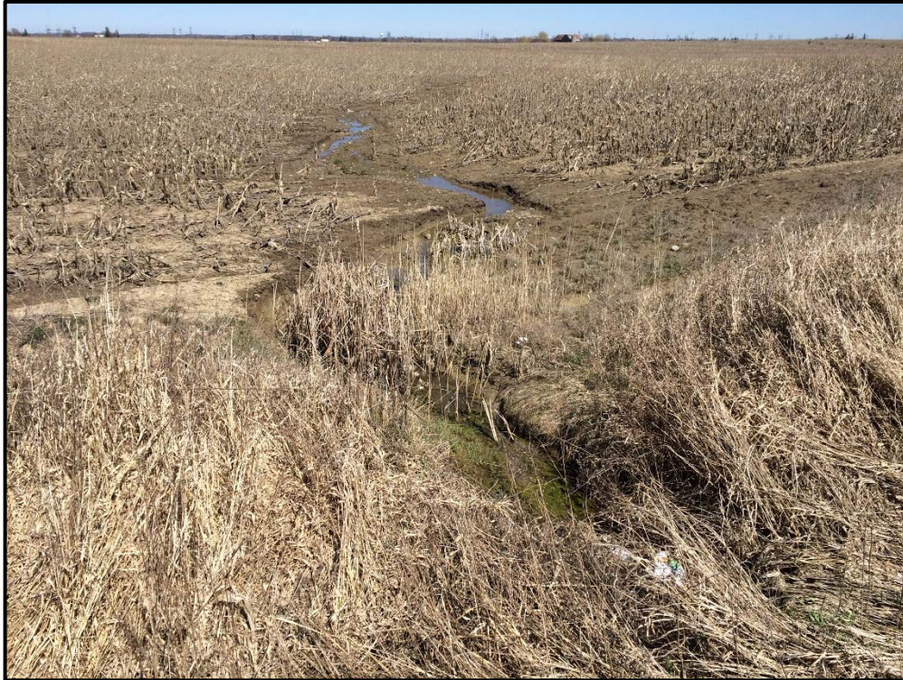
Photo 9: RB4 upstream end of crossing.
