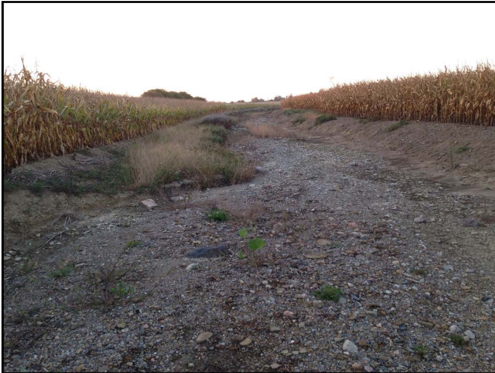
Photo 1: Crossing RB1 downstream. Channel dry with sediment deposition apparent and vegetation within the channel.
