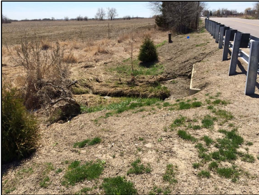
Photo 5: Downstream end of Crossing RB2.
