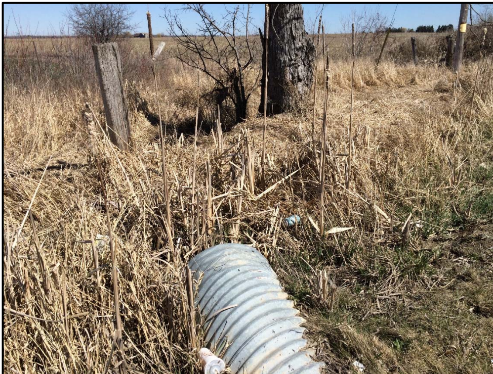
Photo 10: RB4 downstream end of crossing.
