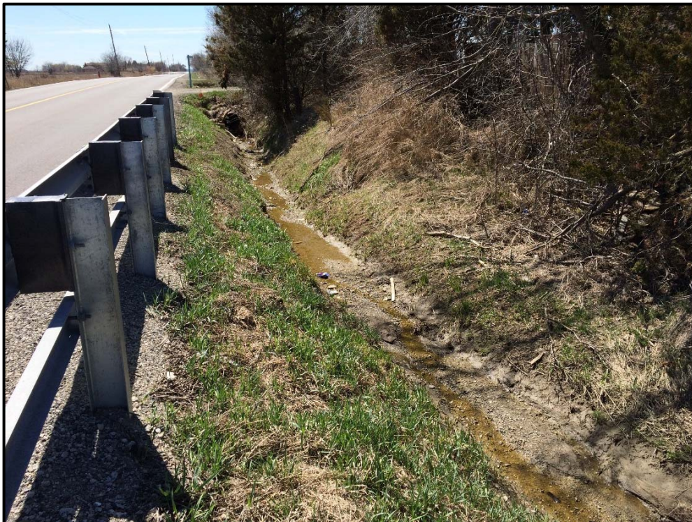
Photo 10: Ditch to west draining to watercourse at Crossing RB2.
