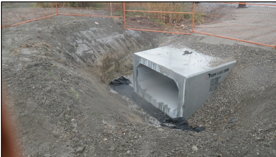
28. Huttonville Creek unnamed tributary – box culvert under construction at the time of field investigations.
