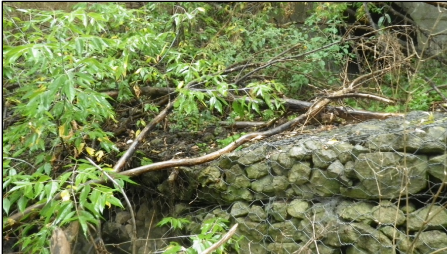
21. Unnamed Credit Trib at Ostrander Boulevard – channel is lined with gabion baskets and scour pad present.
