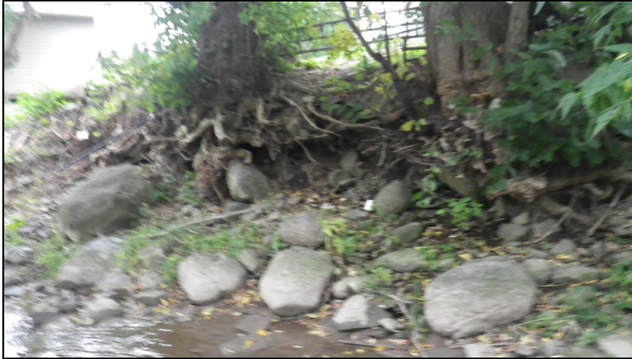
9. Downstream of Credit River Bridge – undercutting of trees and large boulders on right bank
