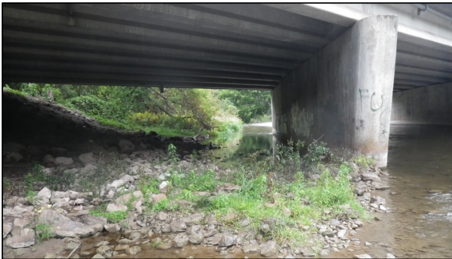
10. Credit River Bridge – channel over widens just downstream of the bridge to compensate for 16 m wide main opening.
