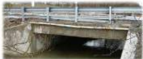
Countryside Drive over Clarkway Tributary
