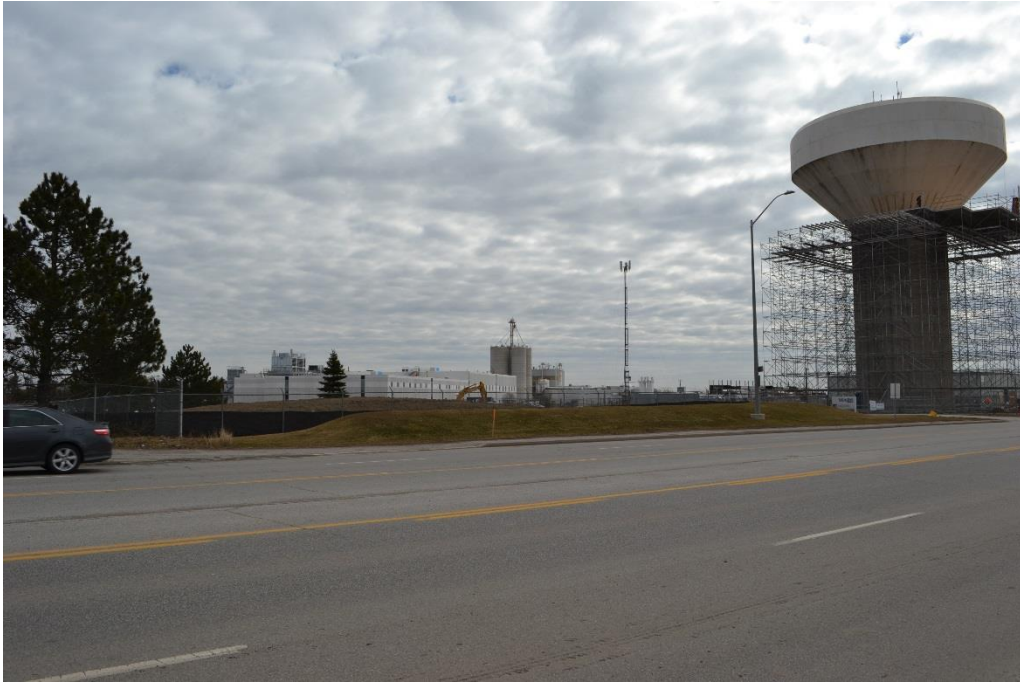
Image 11: Study Corridor; Coleraine Drive; Representative example of industrial disturbance facing southeast, taken March 30, 2017
