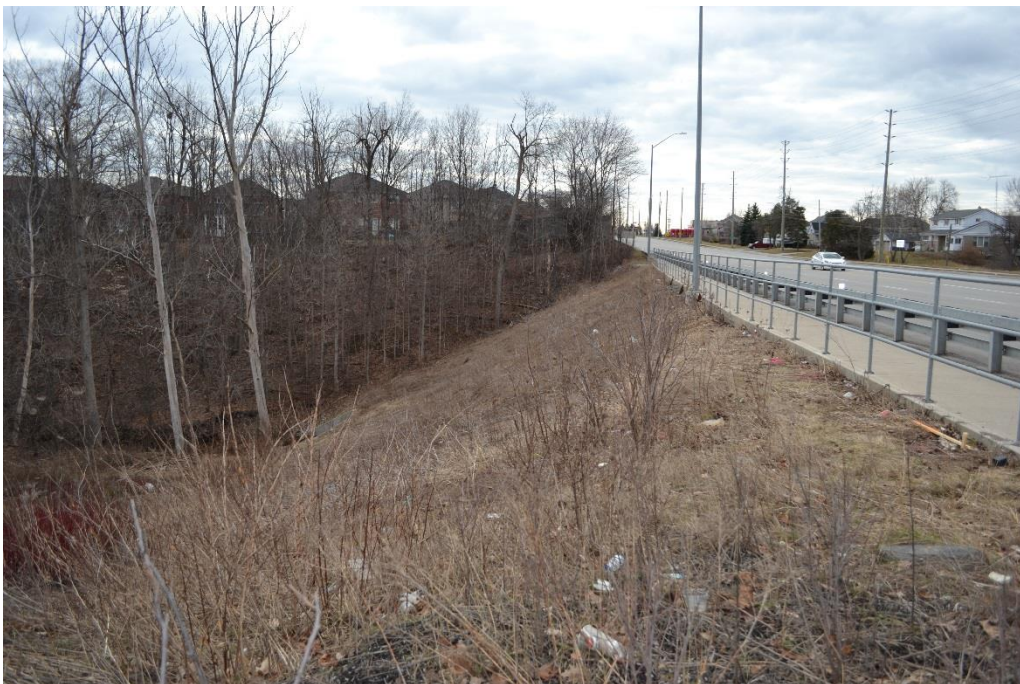
Image 4: Study Corridor; Unnamed tributary of the Humber River showing sloped areas and disturbance from road construction; facing southeast, taken March 30, 2017
