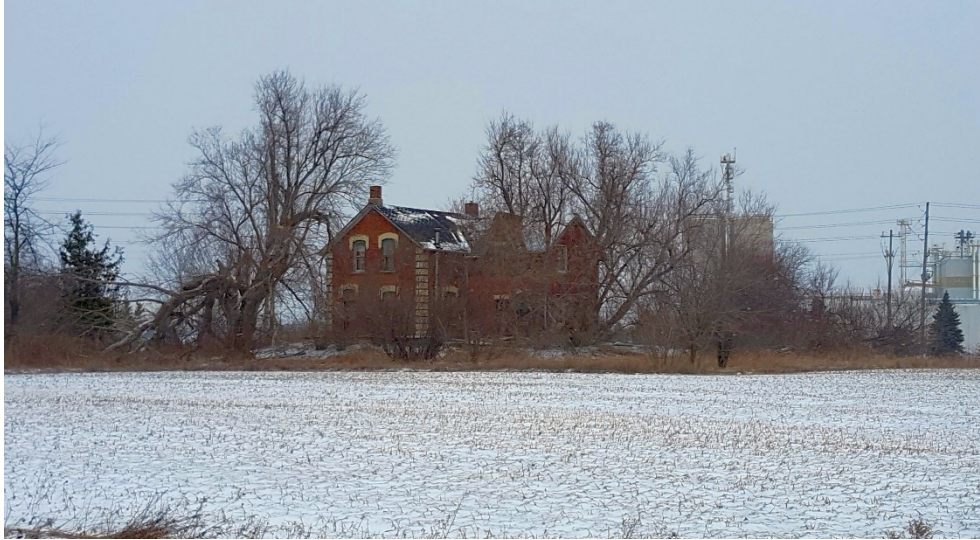
West and south façades, facing northeast
