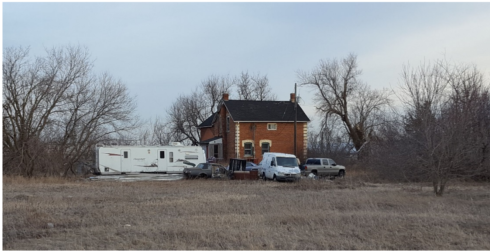
East and north façades, facing south
