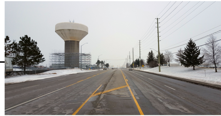
View facing southeast
