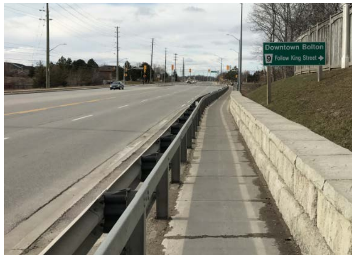
Figure 18 – Narrow Sidewalk Between Guide Rail and Retaining Wall
