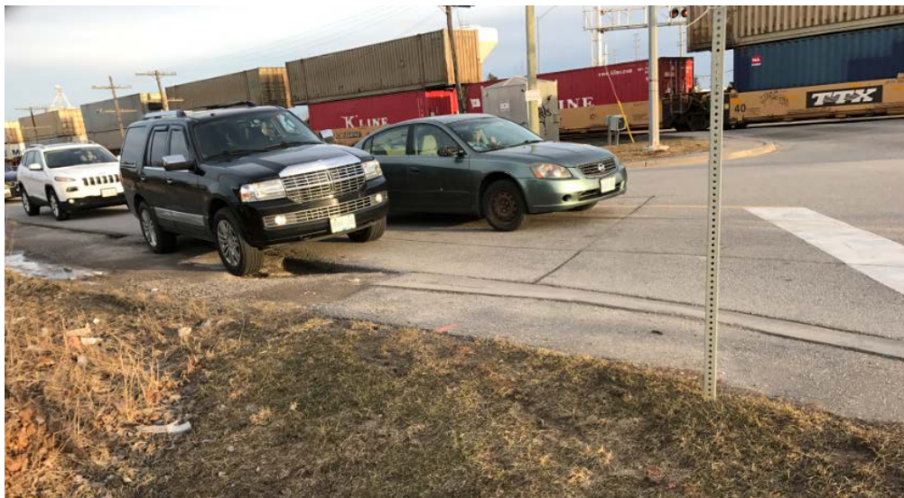
Figure 14 - Right-turning Vehicles Driving Over Shoulder at Old Ellwood Drive
