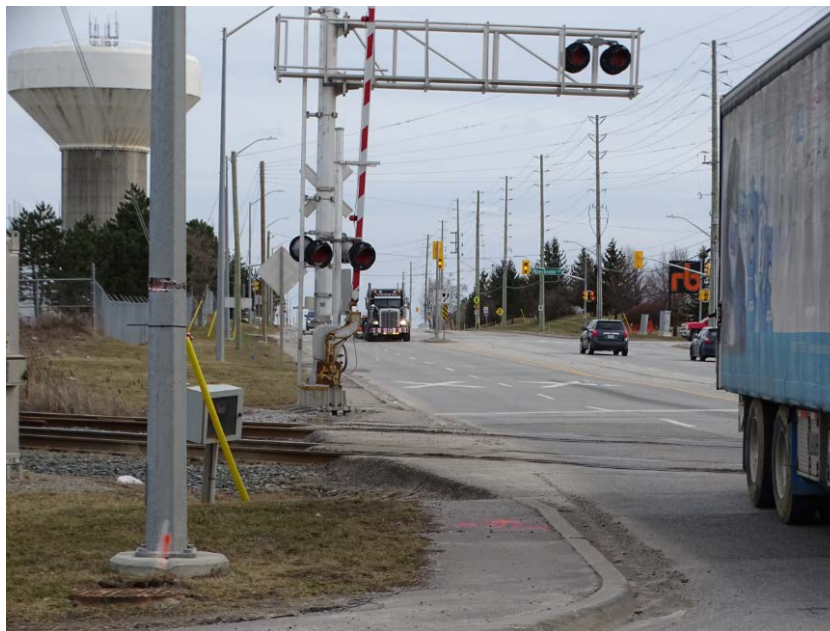
Figure 6 – Railway Signal/Gate Structure Obstructing Sight Line
