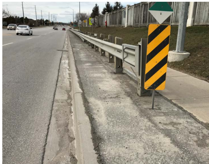
Figure 11 - Guide Rail Installed Behind Barrier Curb
