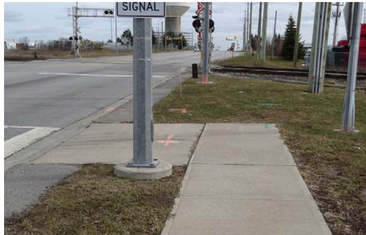
Figure 17 – Sidewalk Termination with No Facilities to Cross Railway Tracks
