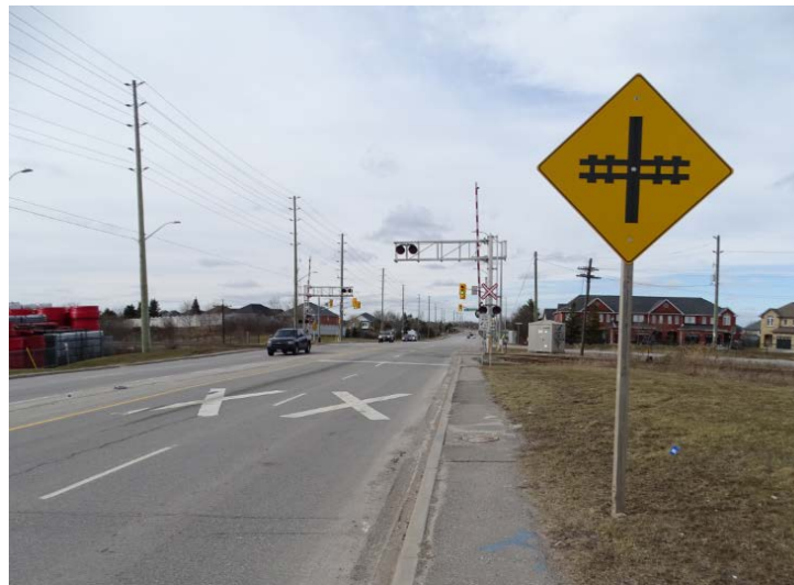
Figure 8 – Railway Crossing Warning Sign Too Close to Tracks
