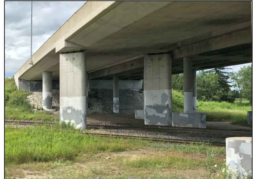
Highway 50, Caledon ON
