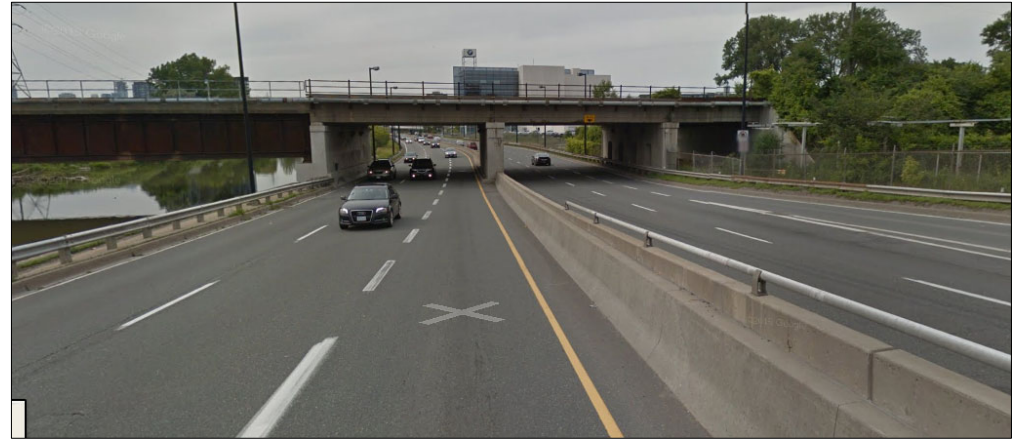
Gardiner Expressway, Toronto ON
