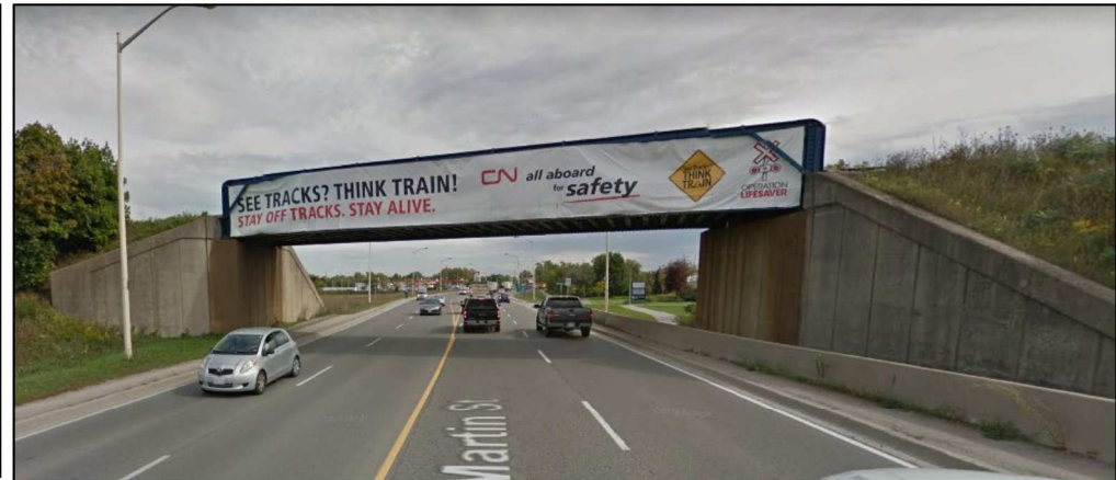
Regional Road 25, Milton ON
