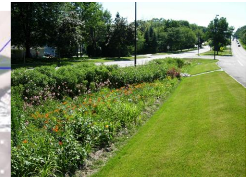
Example of LID stormwater management facility
