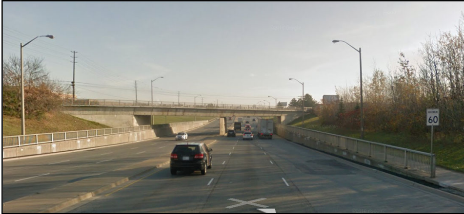
Guelph Line, Burlington ON
