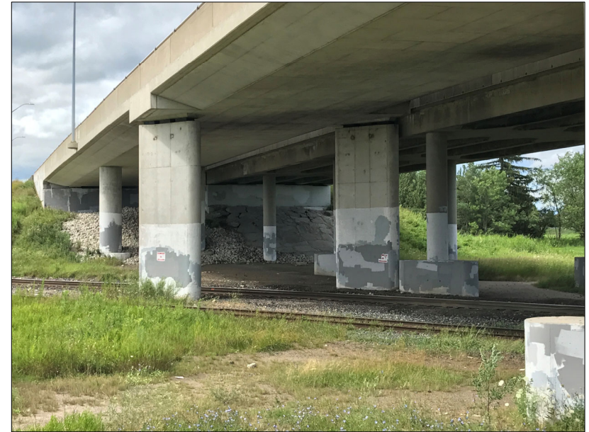
Highway 50, Caledon ON
