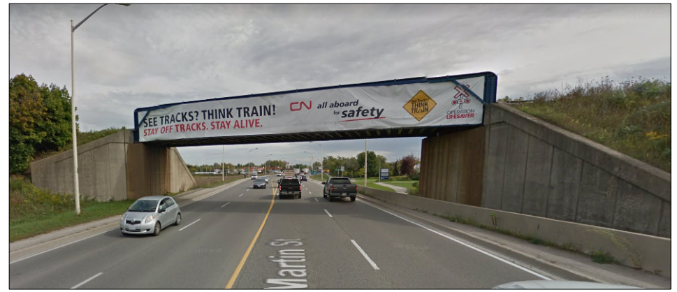
Regional Road 25, Milton ON
