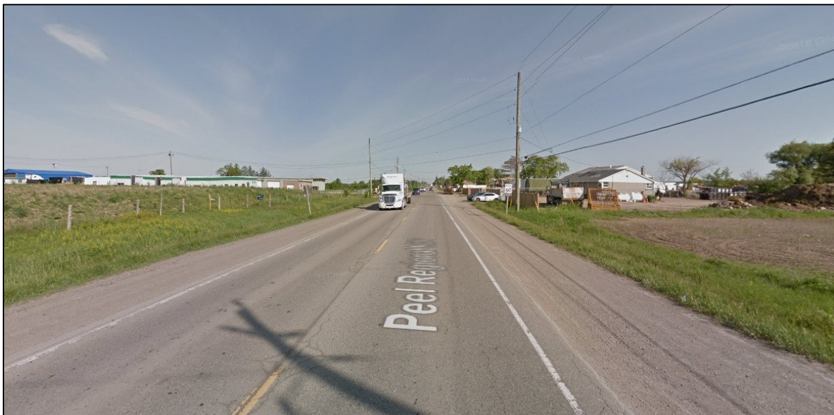
Figure 5: Airport Road, south of Sandhill facing northwest (Google)
