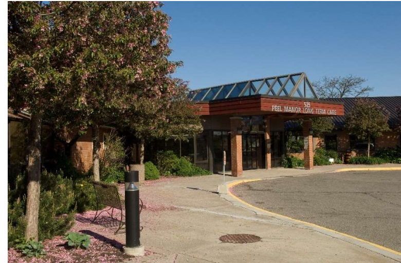
Peel Manor long term care home: currently being redeveloped to the new Seniors Health and Wellness Village.
