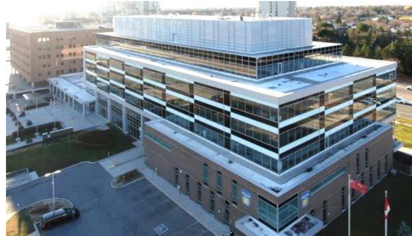
Peel Regional Headquarters at 10 Peel Centre Drive.
