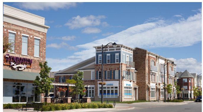
Example of low-rise mixed-use development
